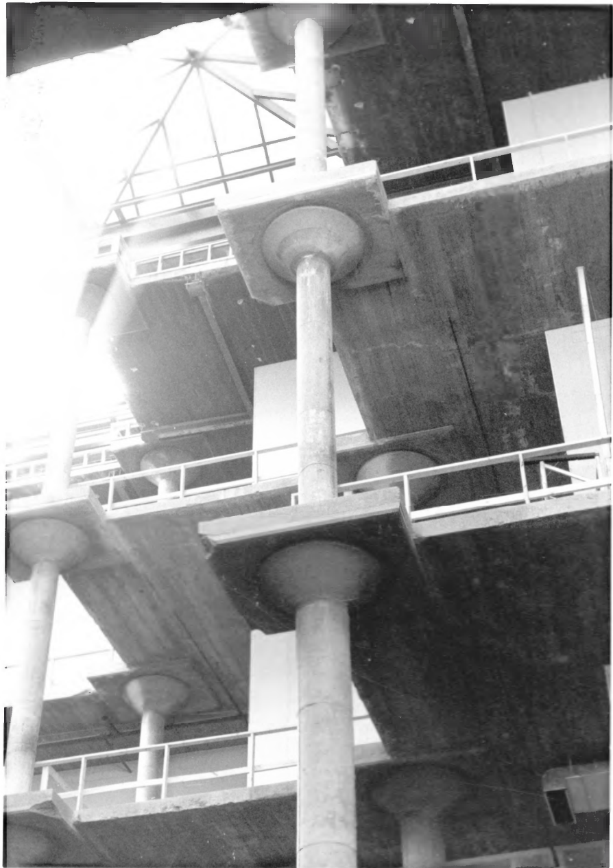
B-F, WAREHOUSE 'A', LOUISVILLE, J&H Co., Ky. PHOTO #12
