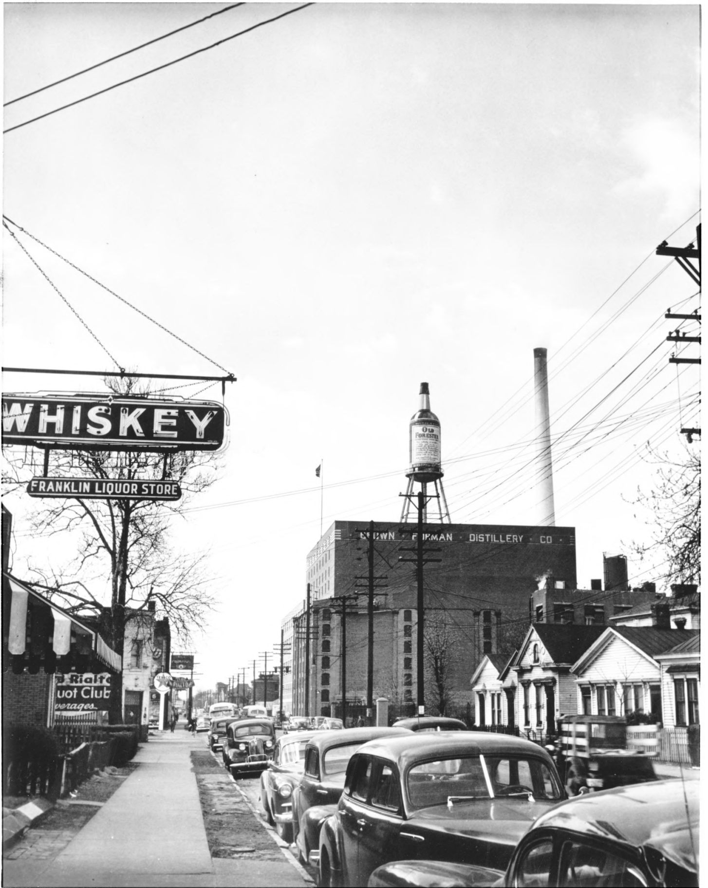
BROWN-FORMAN, WAREHOUSE 'A', LOUISVILLE, JEFFERSON COUNTY, KENTUCKY — PHOTO #4
