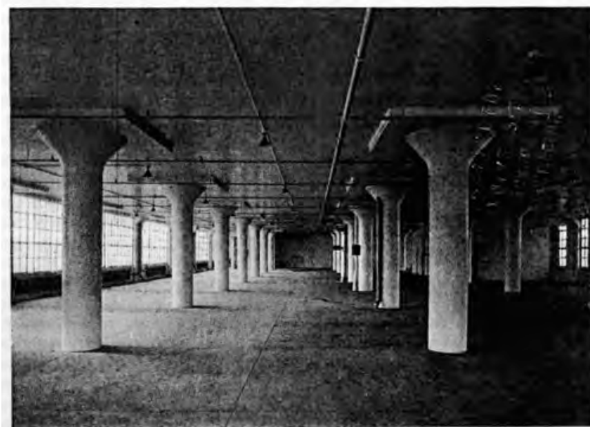
Interior of typical flat slab concrete building, showing use of gloss white paint to increase effective illumination. Tiffin Building, Long Island City, N. Y. The Ballinger Company, Architects and Engineers
