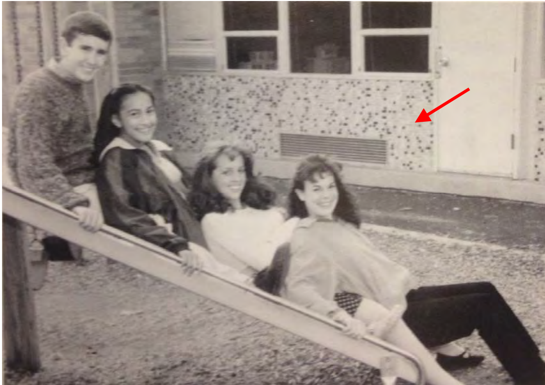
Figure 15: Marion Catholic Church School's original glazed tile under windows, now covered with aluminum panels (see Photo 26) Marion Catholic High School Yearbook (1997) Source: Marion Public Library
