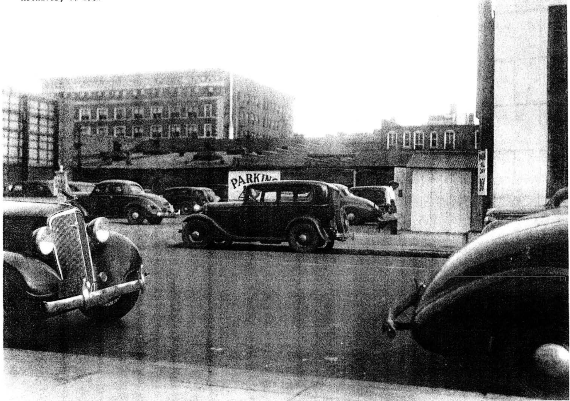
Site of 1958 addition: Tax Assessor's file, Birmingham Public Library Archives, c. 1938
