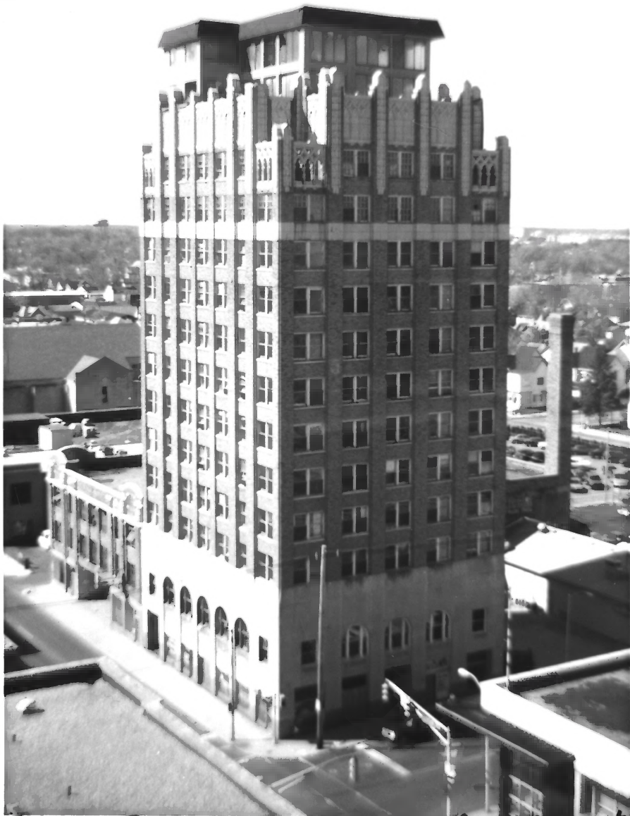
Tower Building Madison Co, IN #4
