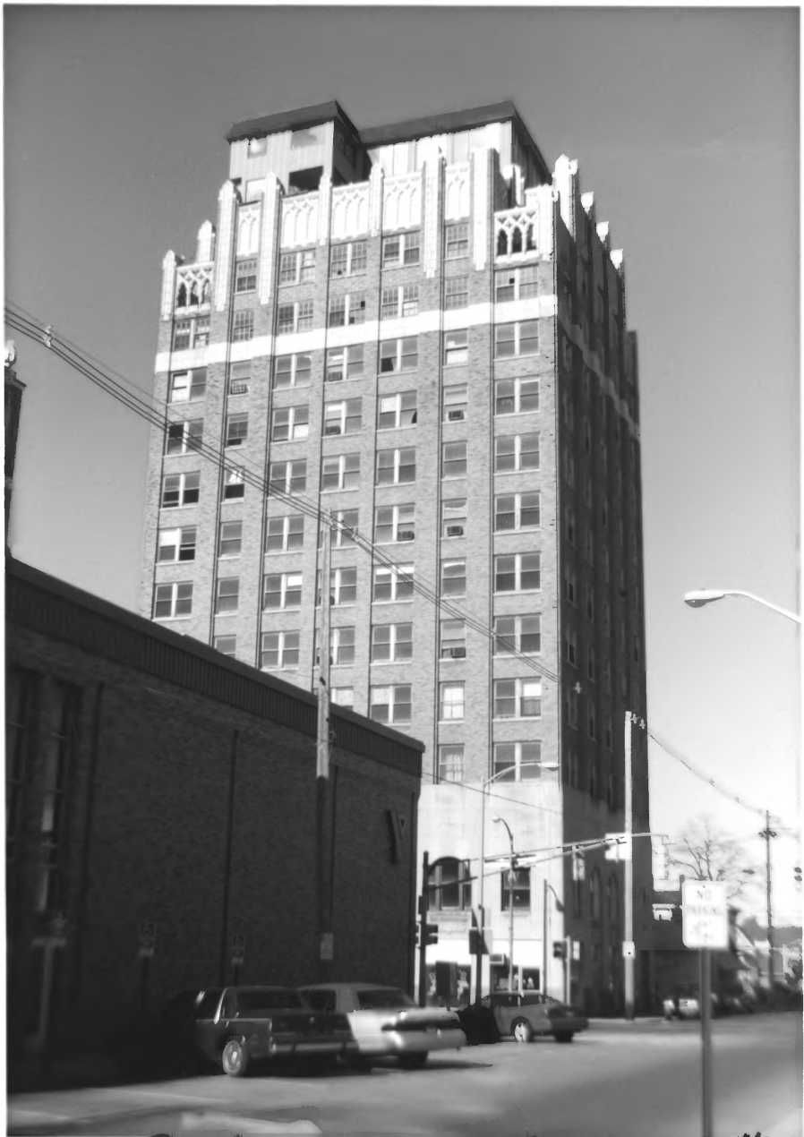
Tower Building, Madison Co., IN #1
