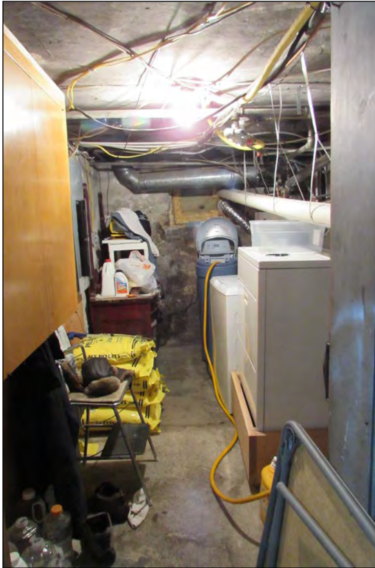
8 of 18. Clegg House—basement; view to the west
