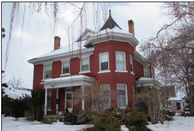
Figure 1. Clegg House; looking southwest
