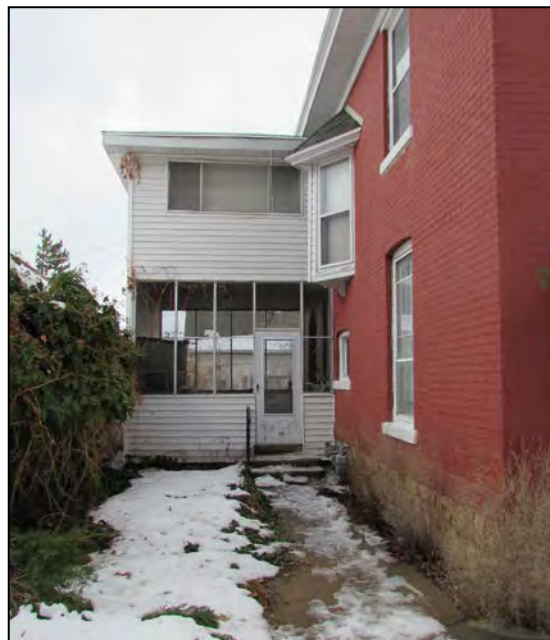
Figure 2. Clegg House addition; looking west
