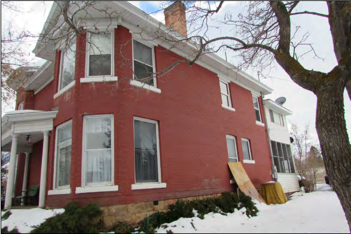
5 of 18. Clegg House—west elevation; camera facing southeast. Note addition at right.
