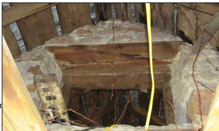
Figure 5. Attic opening in cold storage/workshop; looking west
