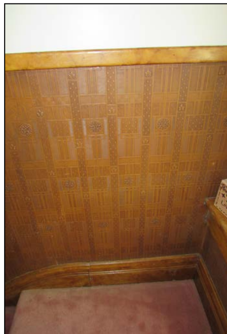
Figure 3. Wallpaper in stairwell
