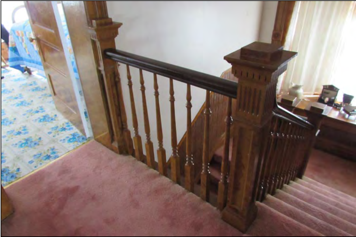
14 of 18. Clegg House—stairwell railing detail; camera facing southwest
