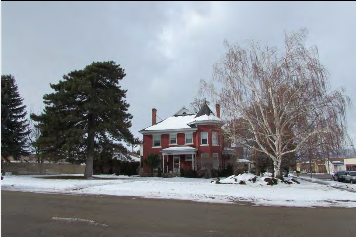
1 of 18. Overview of Clegg House property; camera facing west
