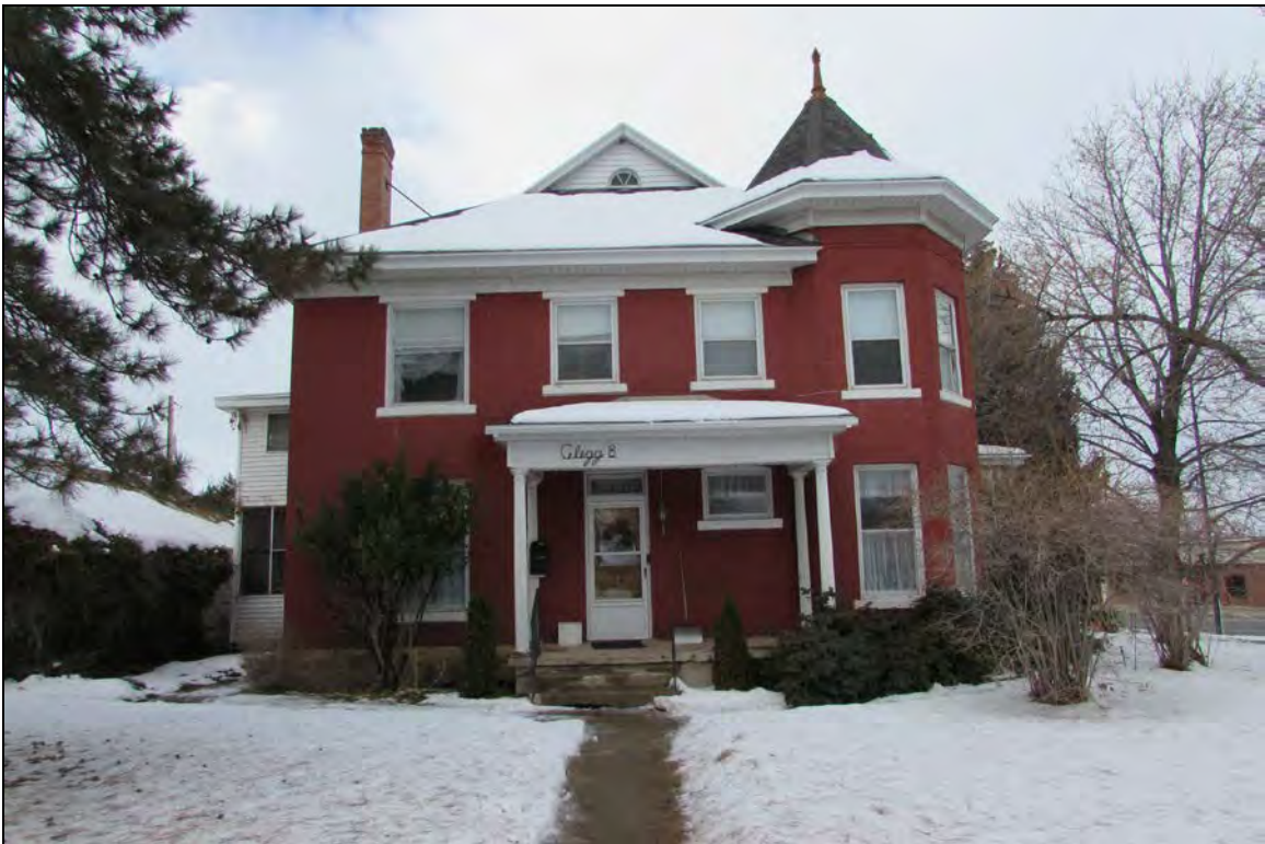
2 of 18. Clegg House—east elevation; camera facing west
