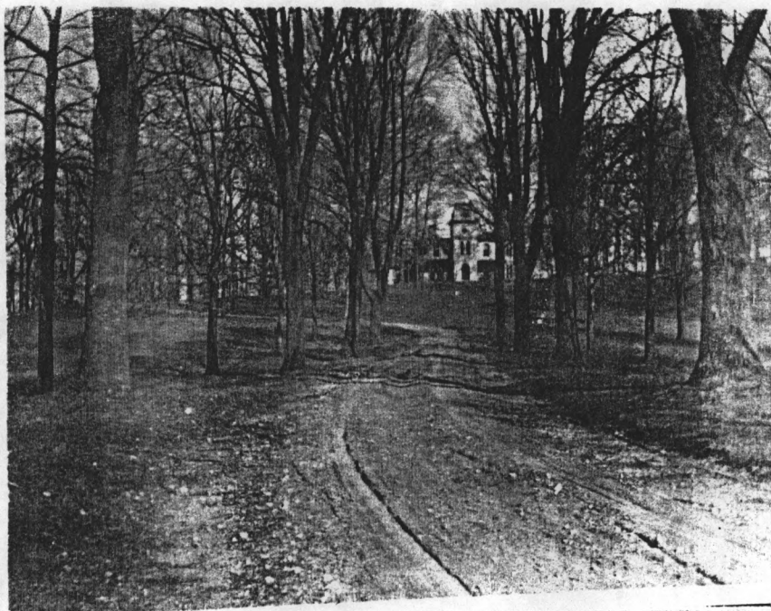
Figure 12: c. 1910. Clarksville, Tennessee. (Top) View of James Glenn house (1857) from southeast, with snow on ground. (Bottom) View of James Glenn house from south, looking up road from Madison Street. Original photo in possession of Frank Childers, Clarksville, Tennessee.
