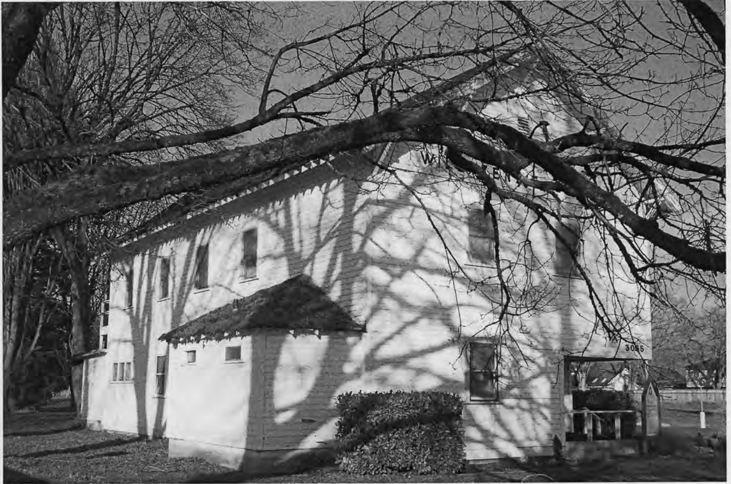
Photo 3 of 12: South and west elevations with bathroom addition, facing northeast.
