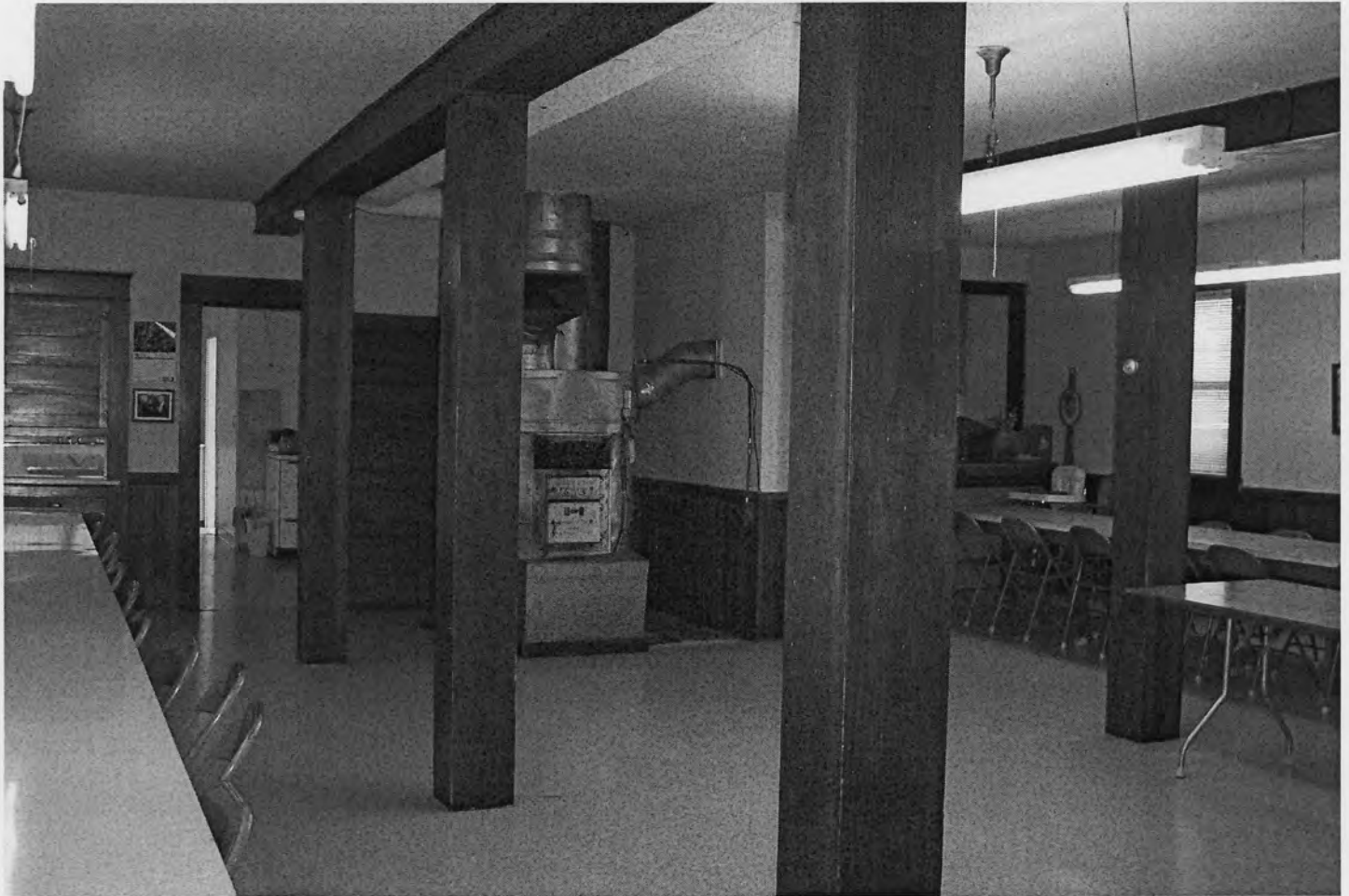
Photo 7 of 12: Ground floor dining hall, facing northeast.
