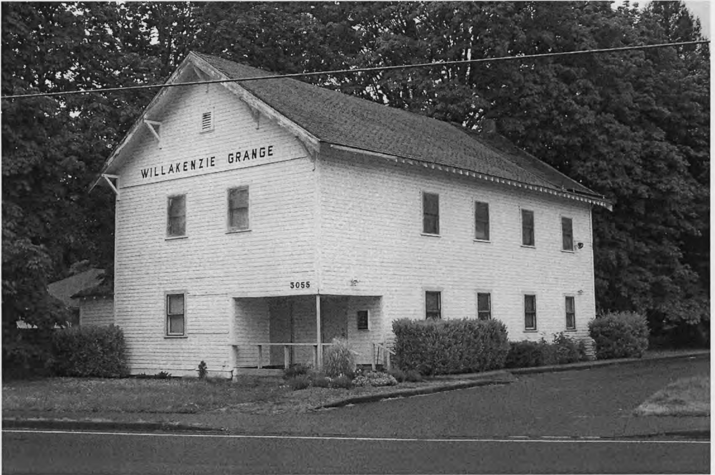
Photo 2 of 12: South and east elevations, facing northwest.
