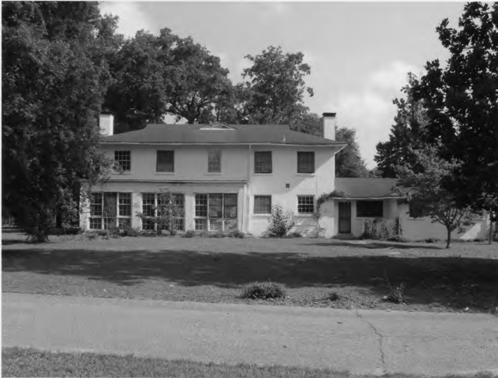
16. Charleston Naval Hospital Historic District North Charleston, Charleston County, South Carolina
