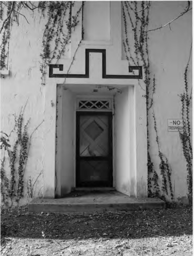
18. Charleston Naval Hospital Historic District North Charleston, Charleston County, South Carolina
