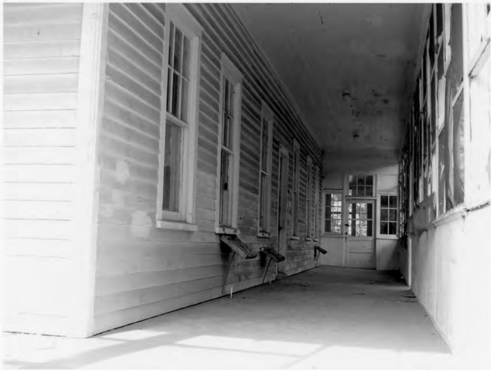
21. Charleston Naval Hospital Historic District North Charleston, Charleston County, South Carolina
