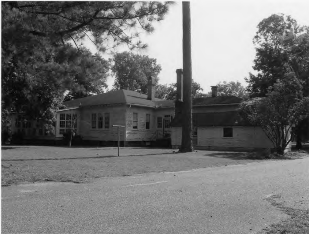
20. Charleston Naval Hospital Historic District North Charleston, Charleston County, South Carolina
