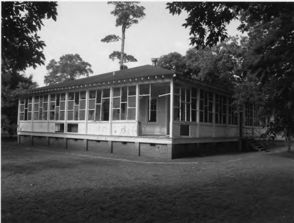
19. Charleston Naval Hospital Historic District North Charleston, Charleston County, South Carolina
