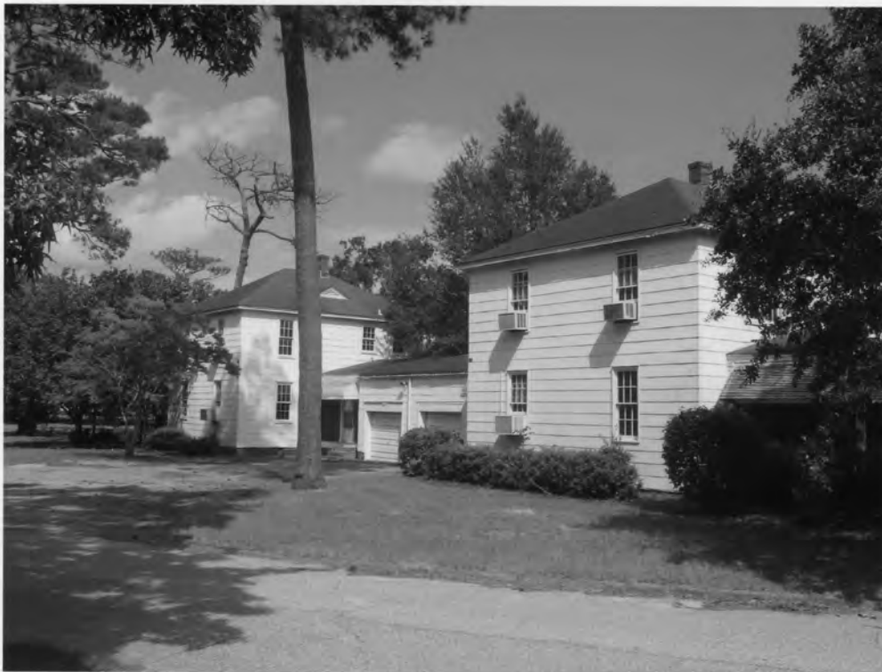
30. Charleston Naval Hospital Historic District North Charleston, Charleston County, South Carolina
