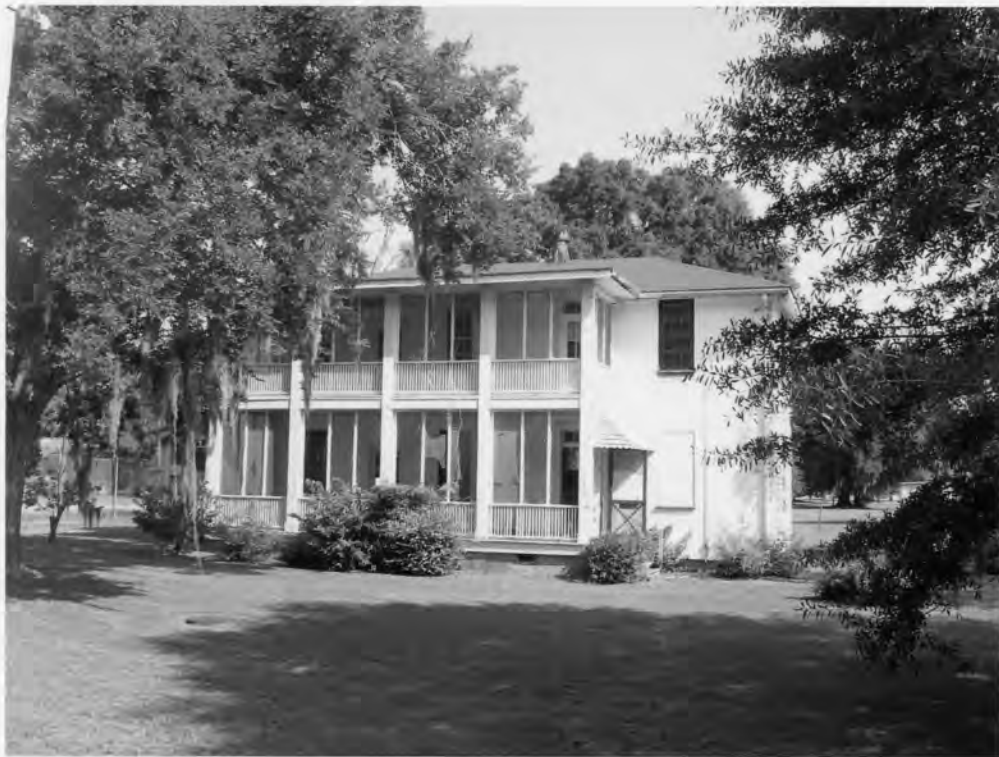
25. Charleston Naval Hospital Historic District North Charleston, Charleston County, South Carolina
