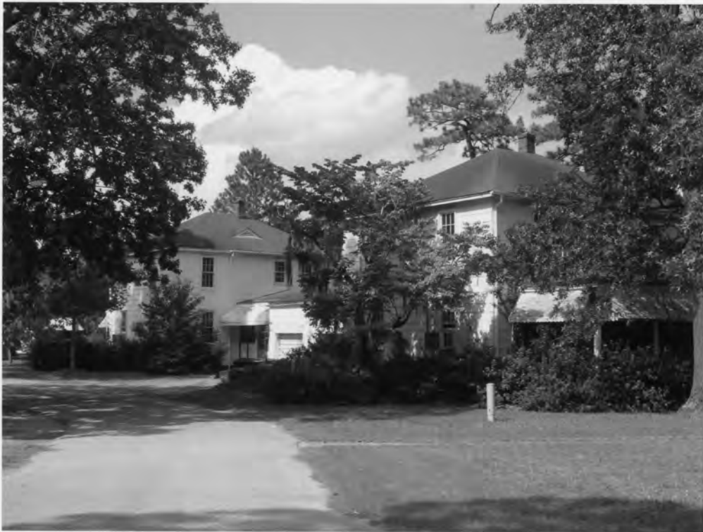
29. Charleston Naval Hospital Historic District North Charleston, Charleston County, South Carolina
