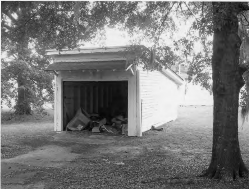
23. Charleston Naval Hospital Historic District North Charleston, Charleston County, South Carolina
