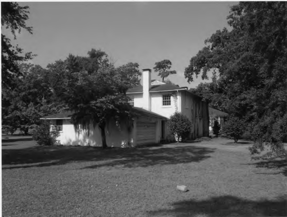
17. Charleston Naval Hospital Historic District North Charleston, Charleston County, South Carolina
