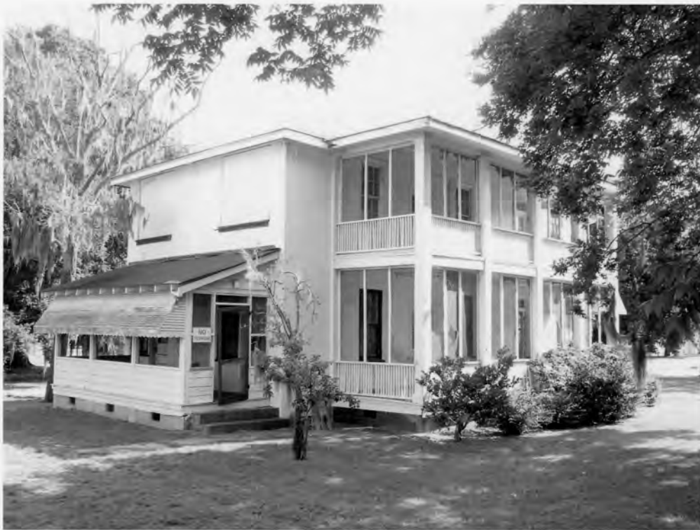
27. Charleston Naval Hospital Historic District North Charleston, Charleston County, South Carolina
