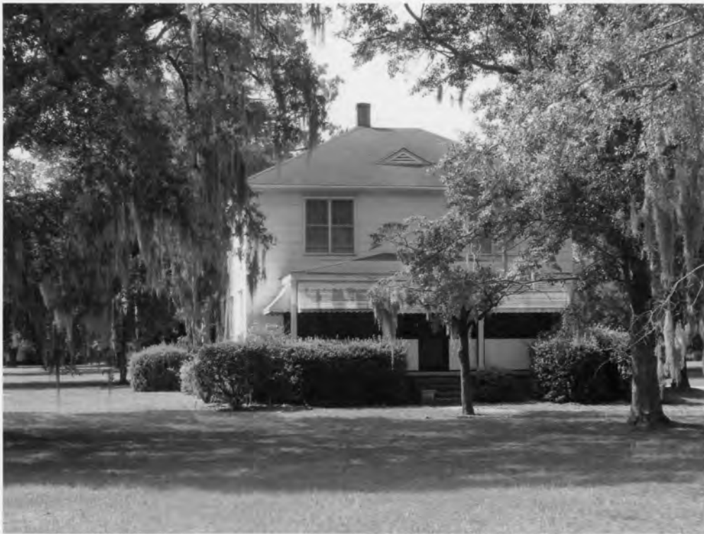
35. Charleston Naval Hospital Historic District North Charleston, Charleston County, South Carolina
