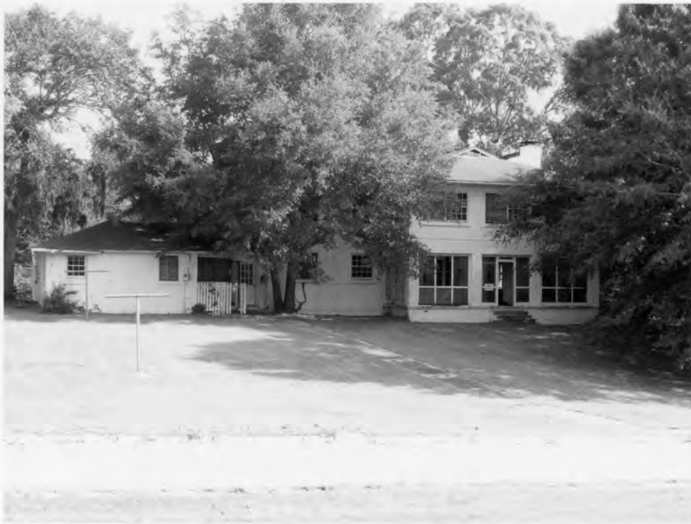
15. Charleston Naval Hospital Historic District North Charleston, Charleston County, South Carolina
