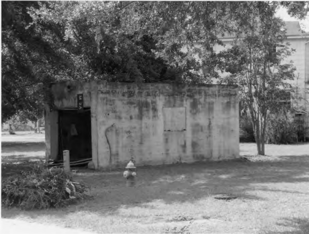
34. Charleston Naval Hospital Historic District North Charleston, Charleston County, South Carolina
