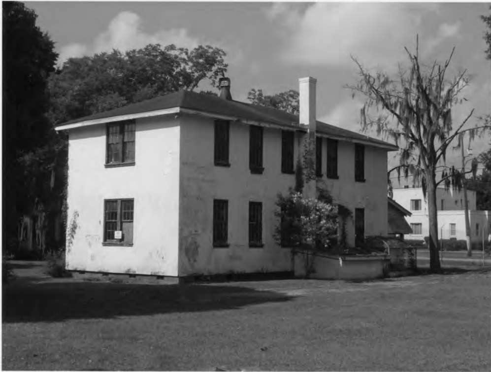
26. Charleston Naval Hospital Historic District North Charleston, Charleston County, South Carolina
