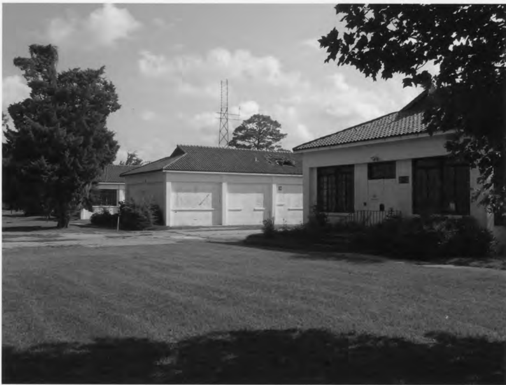
5. Charleston Naval Hospital Historic District North Charleston, Charleston County, South Carolina
