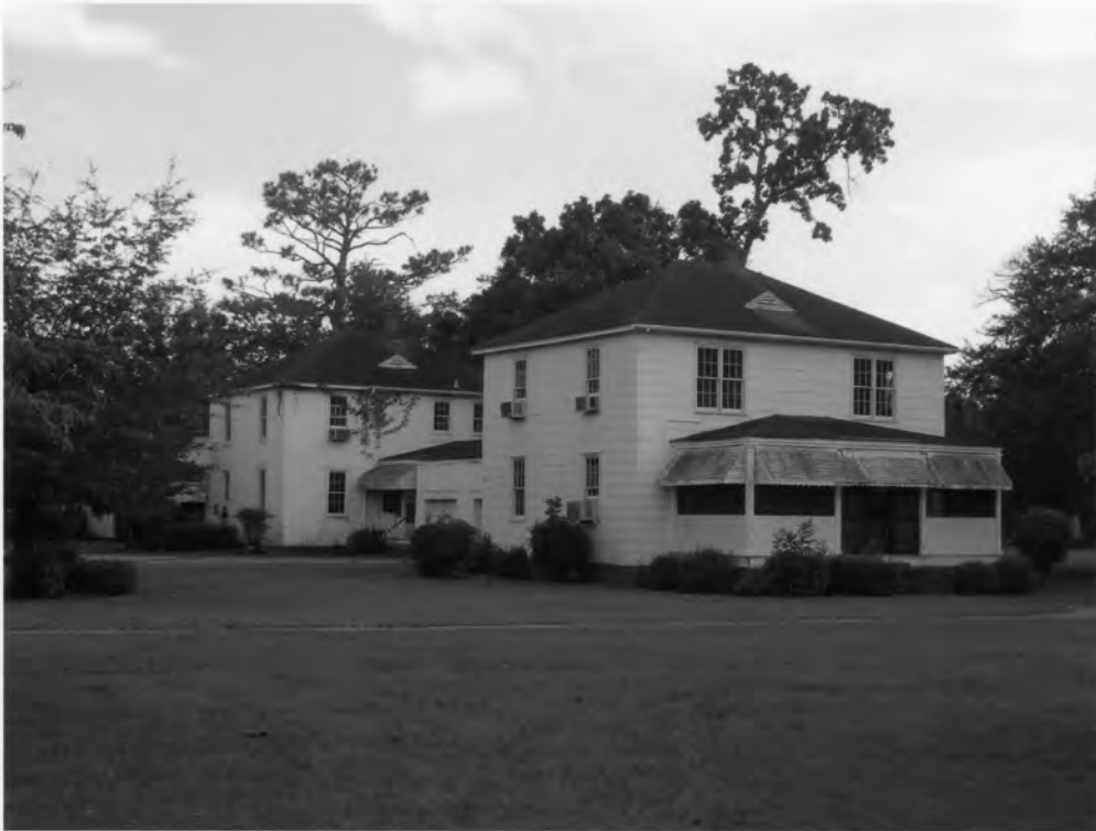
32. Charleston Naval Hospital Historic District North Charleston, Charleston County, South Carolina
