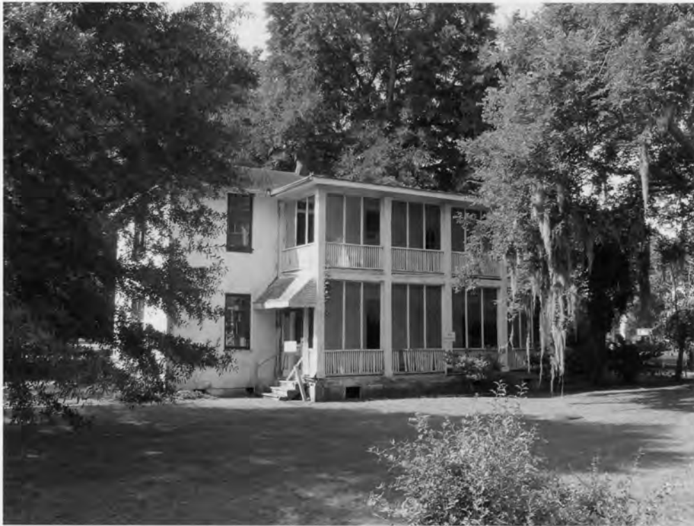
28. Charleston Naval Hospital Historic District North Charleston, Charleston County, South Carolina
