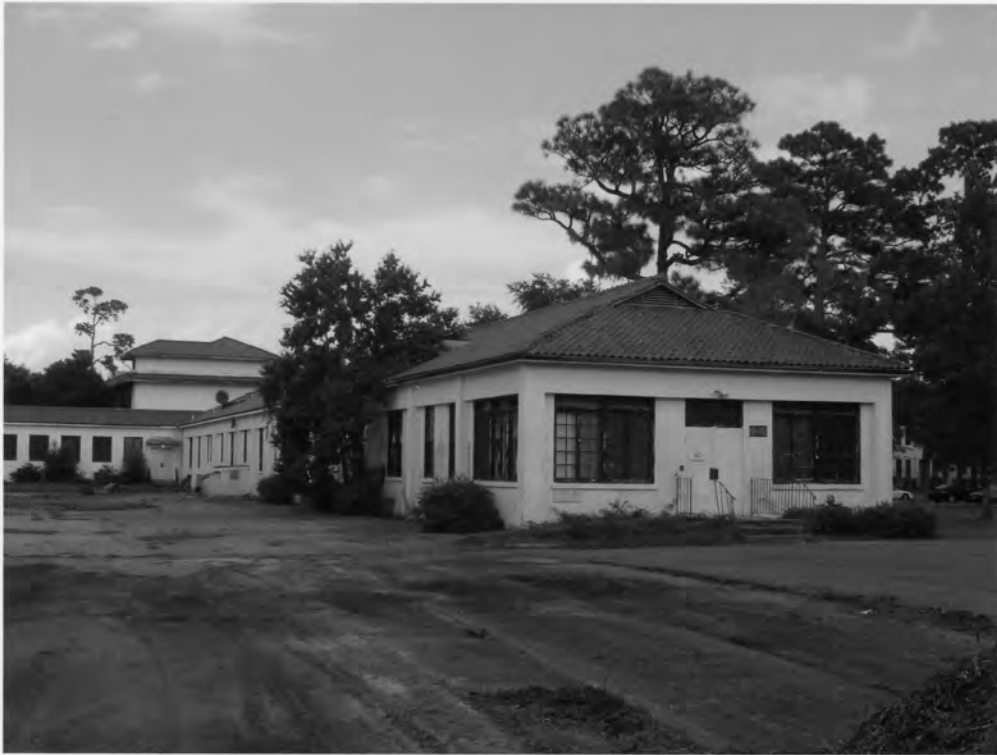
4. Charleston Naval Hospital Historic District North Charleston, Charleston County, South Carolina
