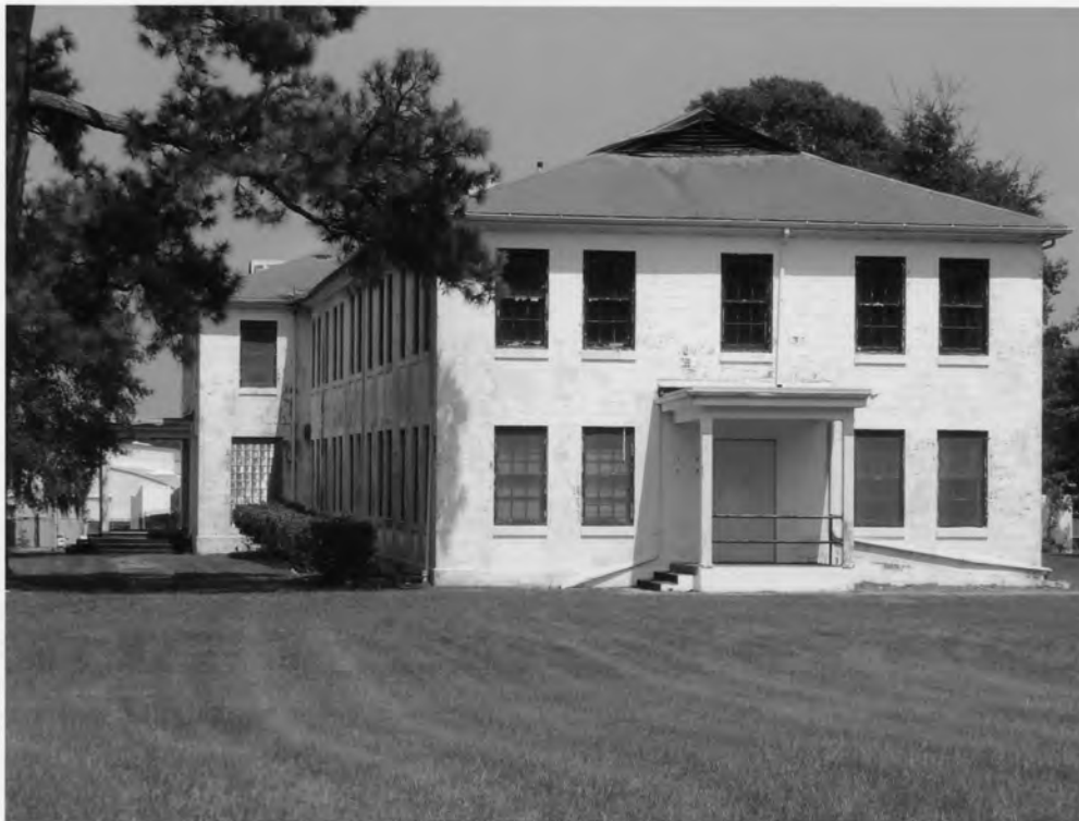
10. Charleston Naval Hospital Historic District North Charleston, Charleston County, South Carolina
