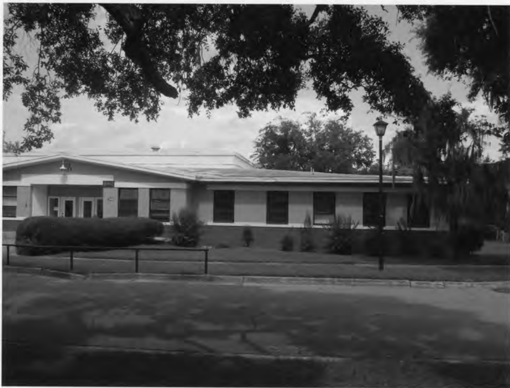
13. Charleston Naval Hospital Historic District North Charleston, Charleston County, South Carolina
