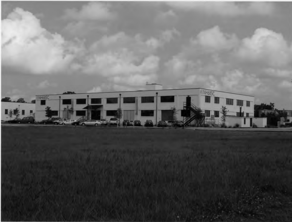
12. Charleston Naval Hospital Historic District North Charleston, Charleston County, South Carolina
