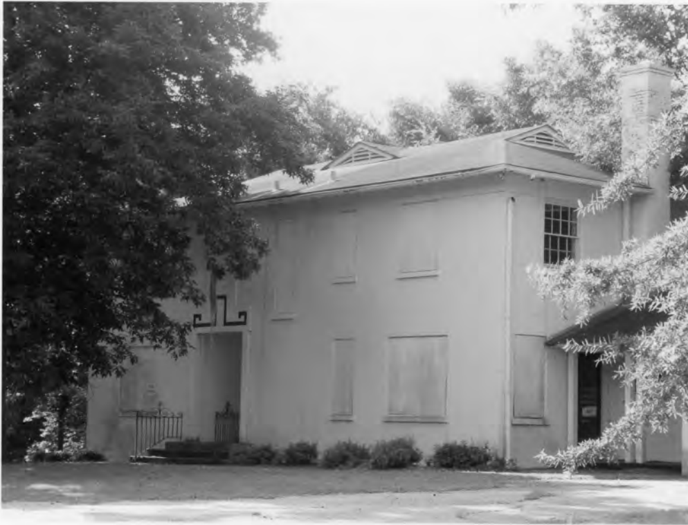
14. Charleston Naval Hospital Historic District North Charleston, Charleston County, South Carolina
