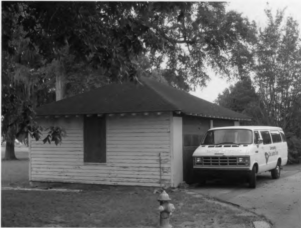
24. Charleston Naval Hospital Historic District North Charleston, Charleston County, South Carolina
