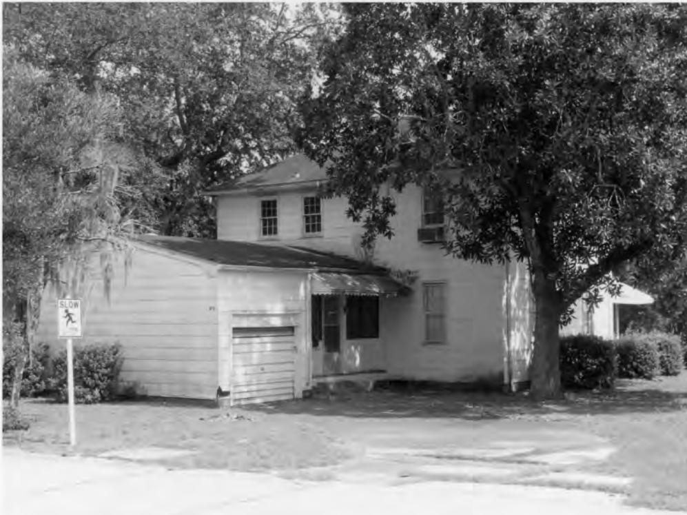
36. Charleston Naval Hospital Historic District North Charleston, Charleston County, South Carolina
