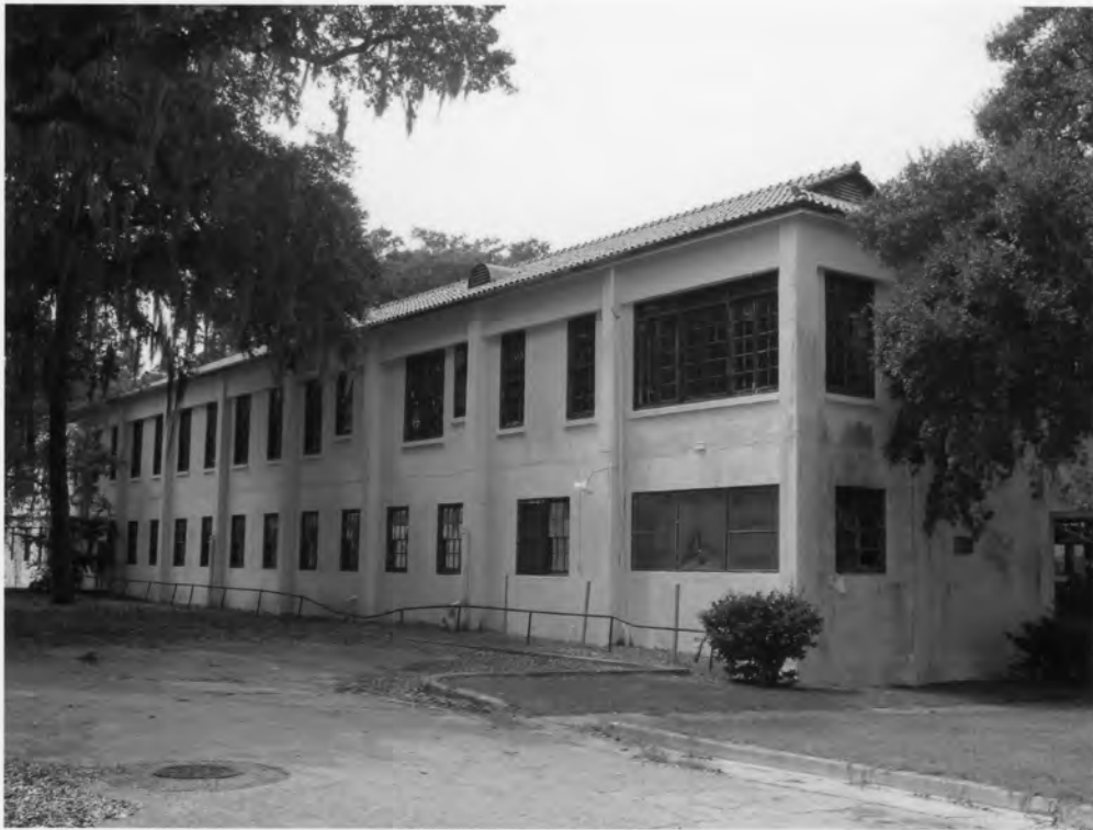
7. Charleston Naval Hospital Historic District North Charleston, Charleston County, South Carolina
