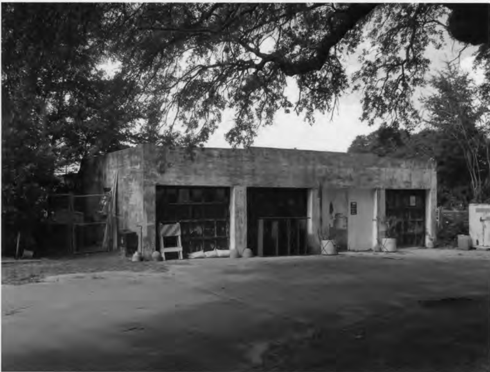
33. Charleston Naval Hospital Historic District North Charleston, Charleston County, South Carolina
