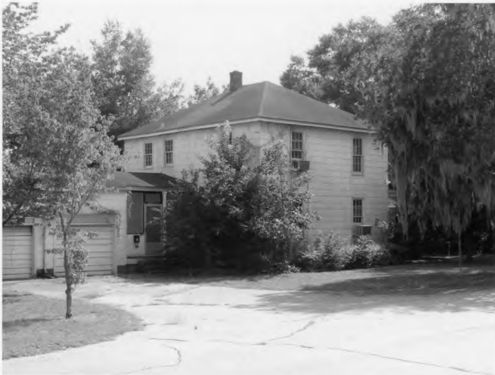
37. Charleston Naval Hospital Historic District North Charleston, Charleston County, South Carolina
