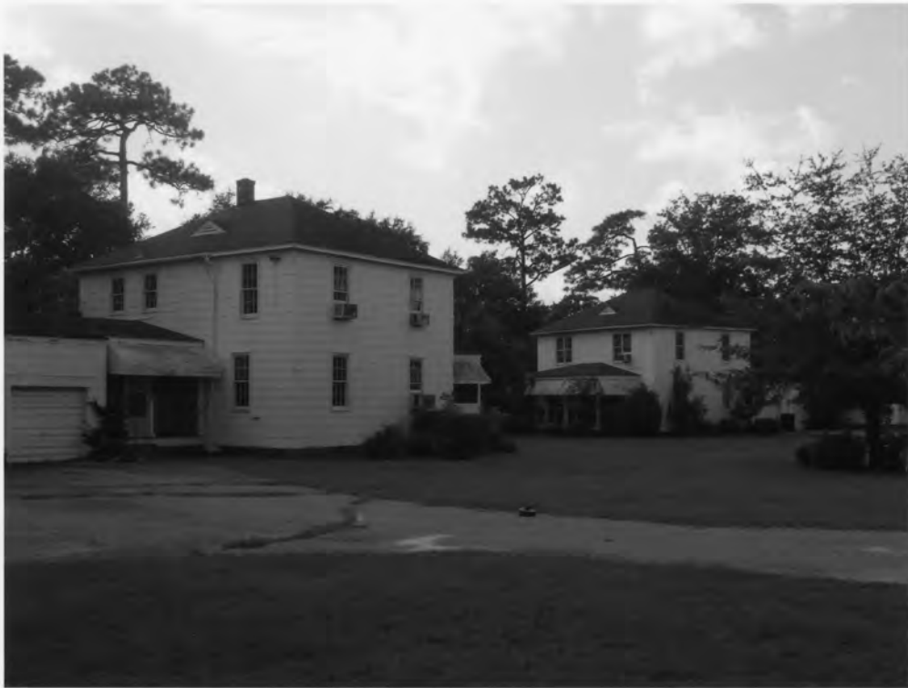
31. Charleston Naval Hospital Historic District North Charleston, Charleston County, South Carolina
