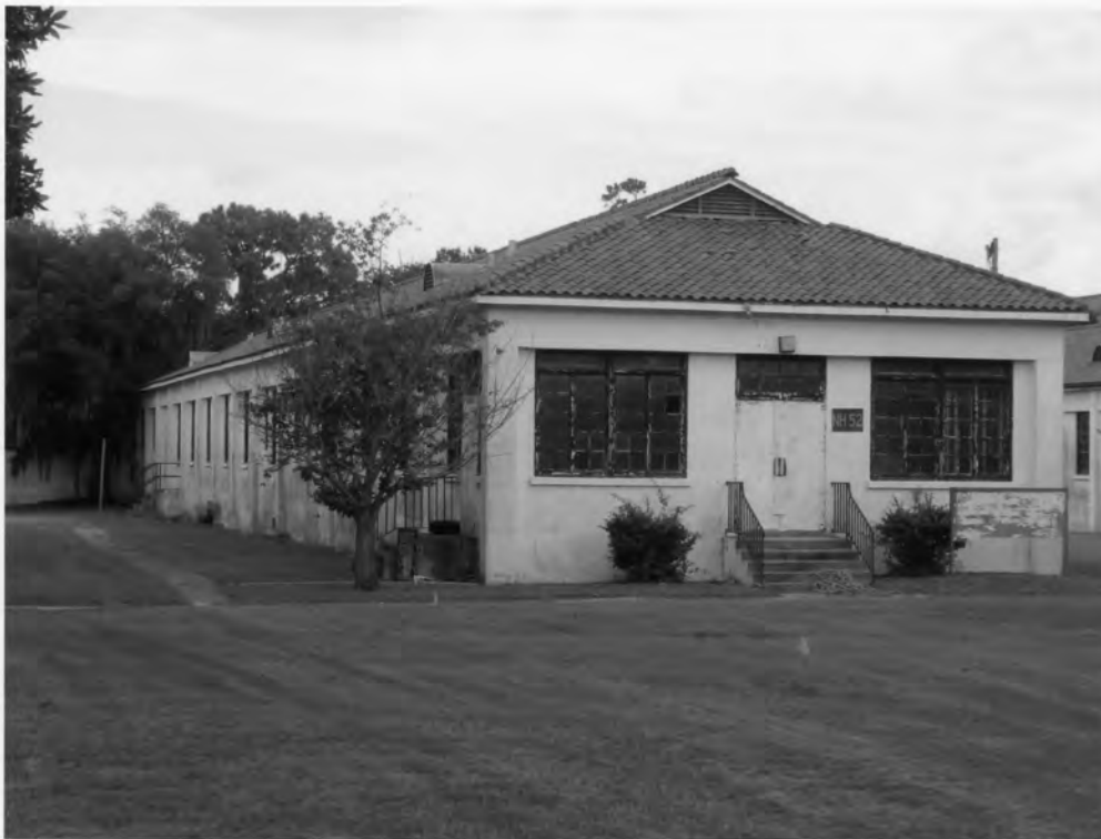
6. Charleston Naval Hospital Historic District North Charleston, Charleston County, South Carolina
