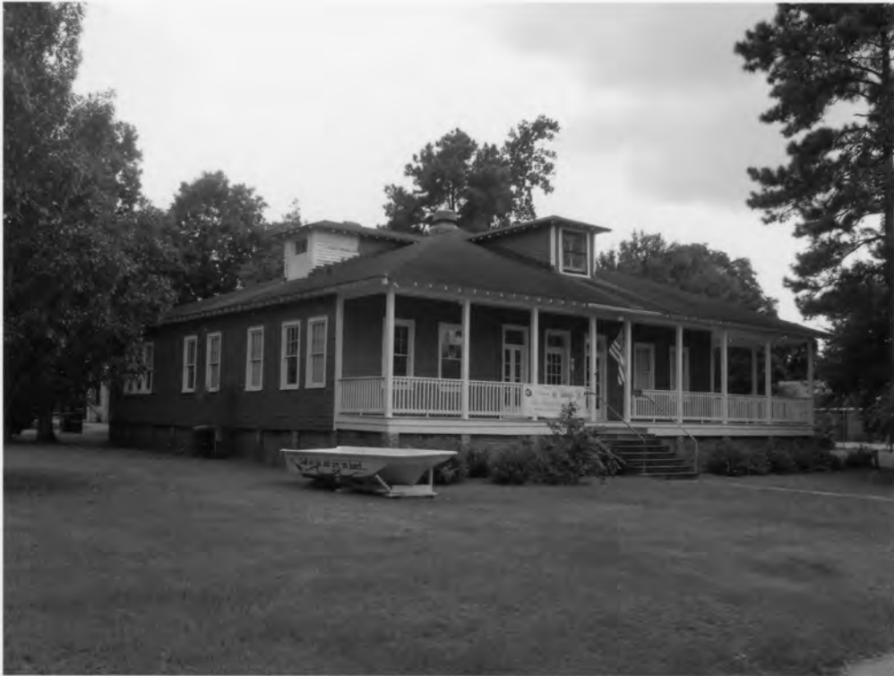
22. Charleston Naval Hospital Historic District North Charleston, Charleston County, South Carolina
