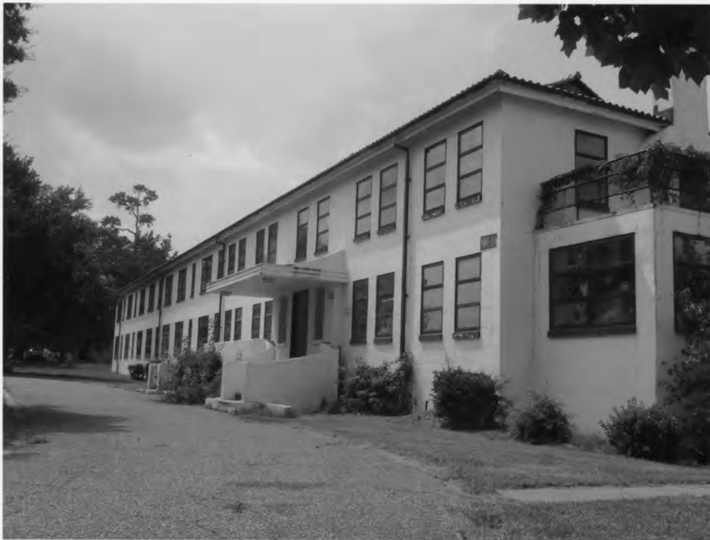
11. Charleston Naval Hospital Historic District North Charleston, Charleston County, South Carolina
