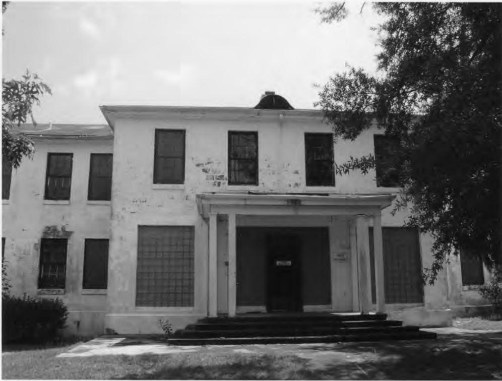
9. Charleston Naval Hospital Historic District North Charleston, Charleston County, South Carolina
