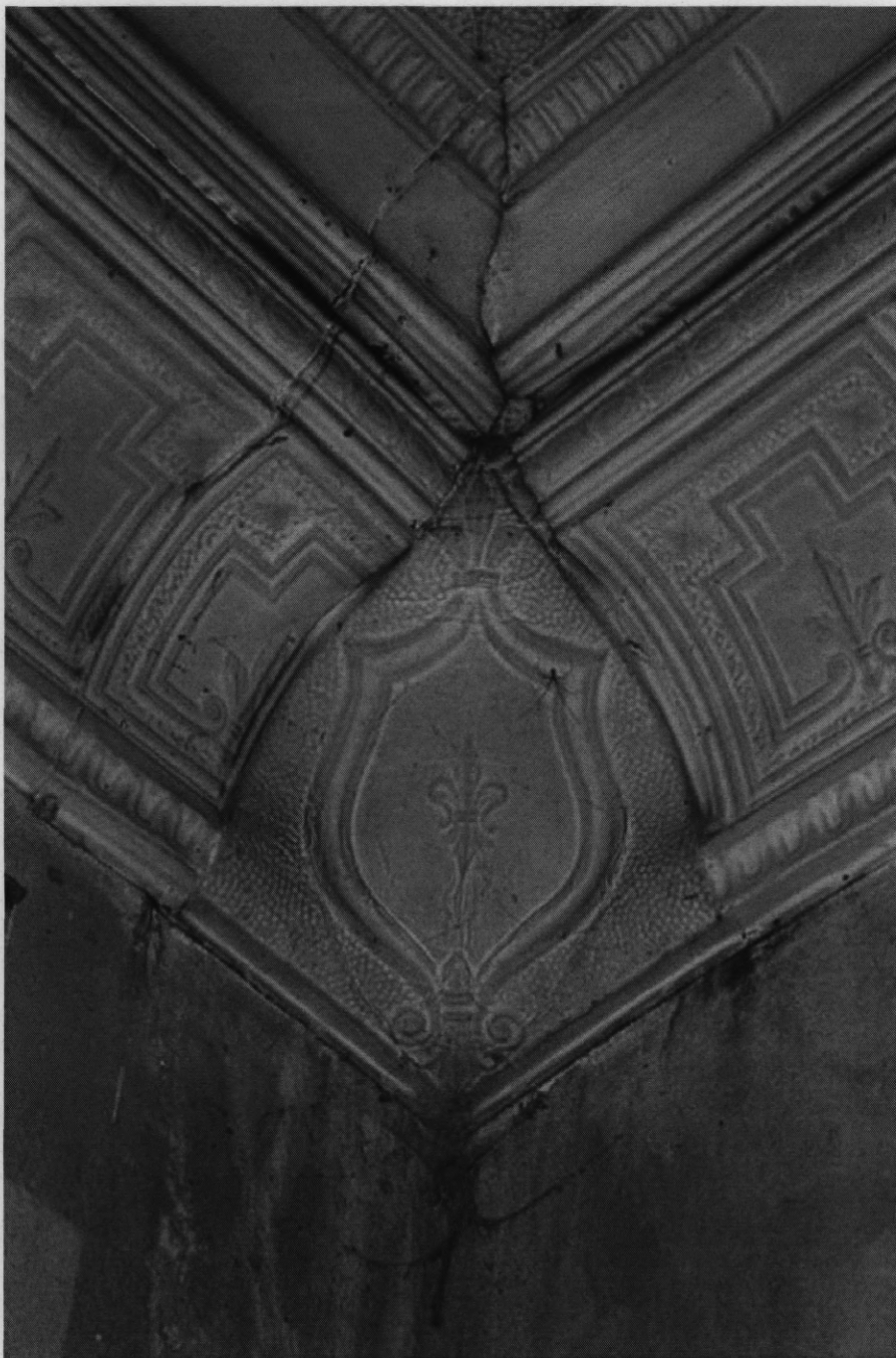
Detail view of ornamental pressed-tin ceiling.
