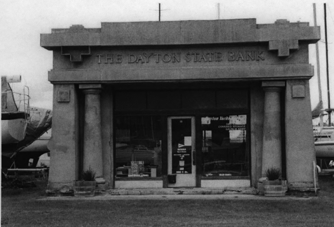
Photo 0001: Primary Elevation, West façade, View to the east.
