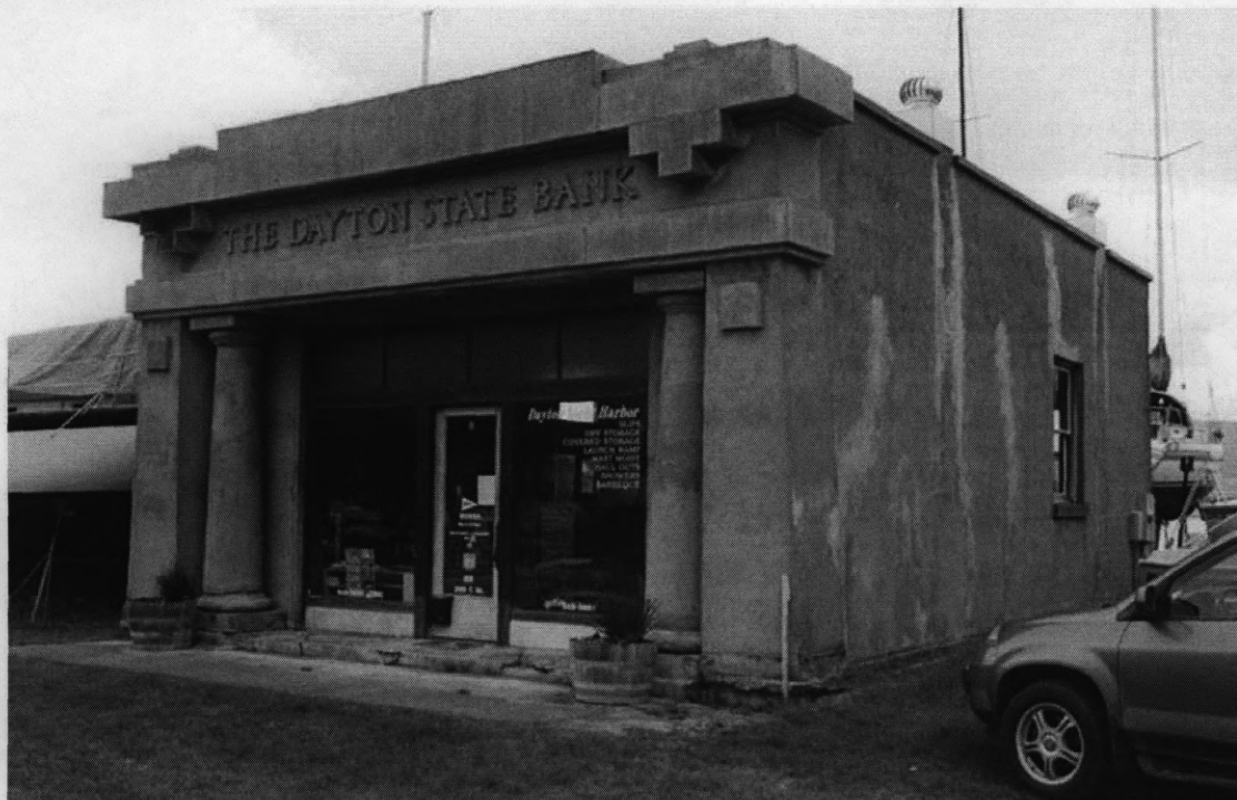
Photo 0002: Above: West and south facades, view to the northeast
