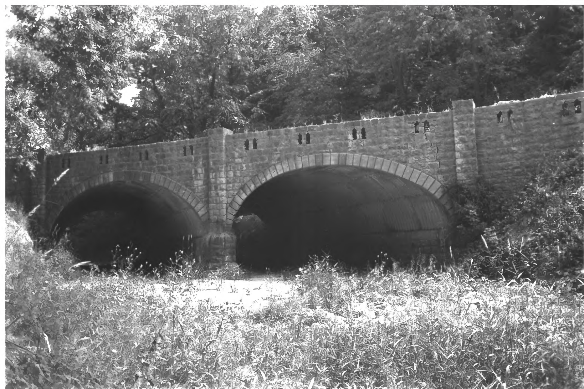
ZUMBRO PARKWAY BRIDGE (NO. 3219) WABASHA CO. MN PHOTO I.D. 09960 # 11
