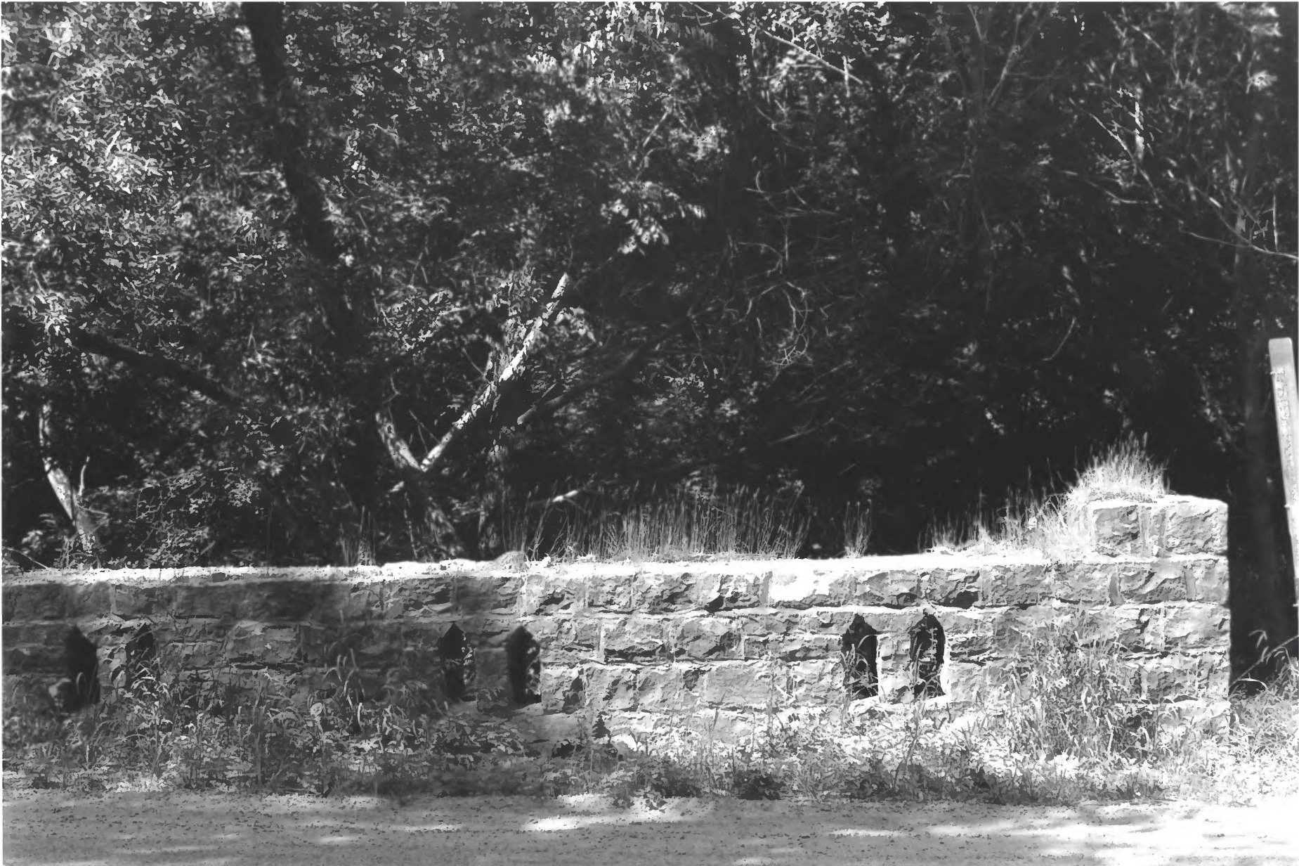
ZUMBRO PARKWAY BRIDGE (NO 3219) WABASHA CO., MN PHOTO I.D. 09660#5
