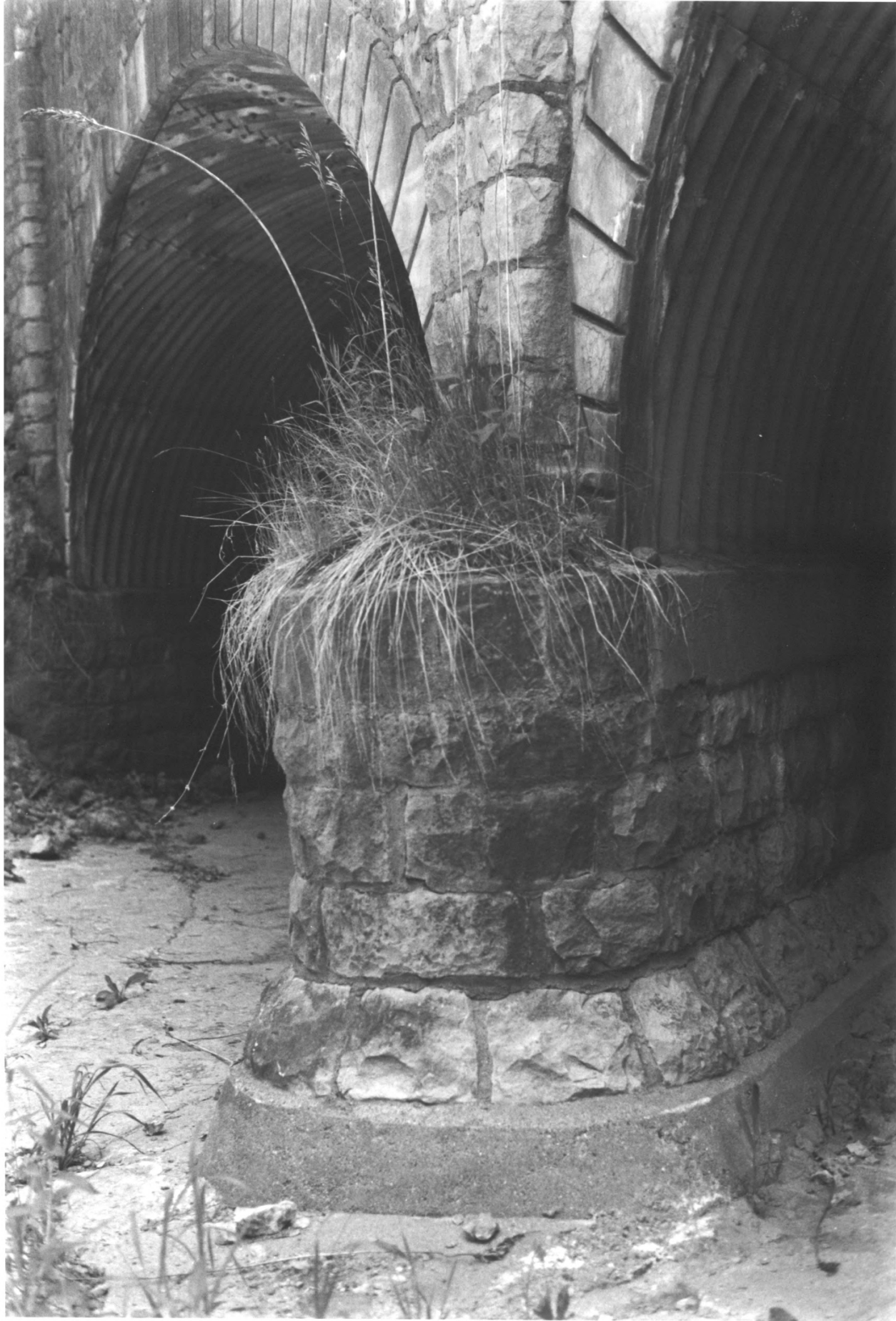
ZUMBERG PARKWAY BRIDGE (NO 3219) WABASHA CO. MN PHOTO I.D. 09660 #14
