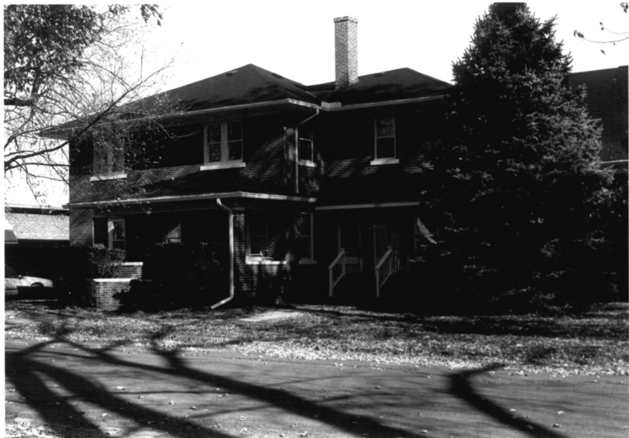
HILLCREST COMMUNITY CENTER - CLINTON, VERMILLION CO., IN. PHOTO NO. 6
