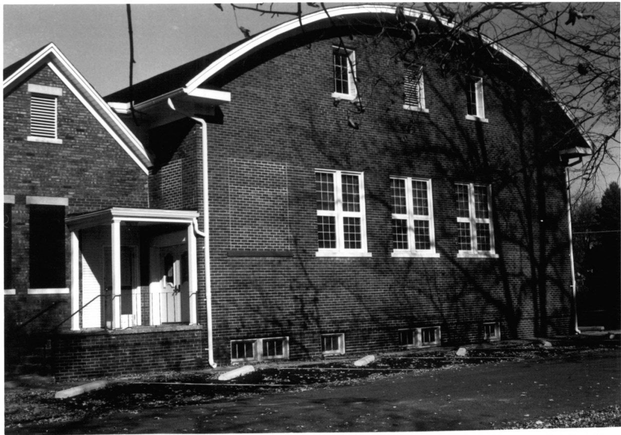
HILLCREST COMMUNITY CENTER, CLINTON, VERMILION CO., INDIANA PHOTO. 3
