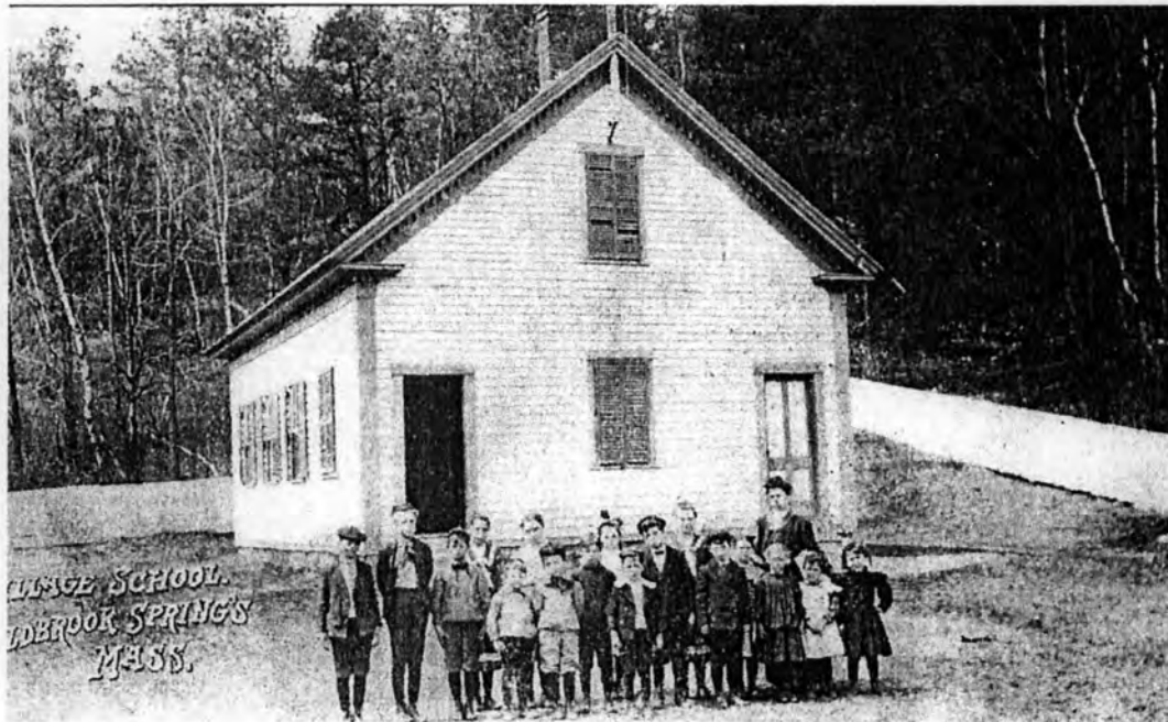
Illustration # 3 Coldbrook School, Oakham, built c. 1850(?)
