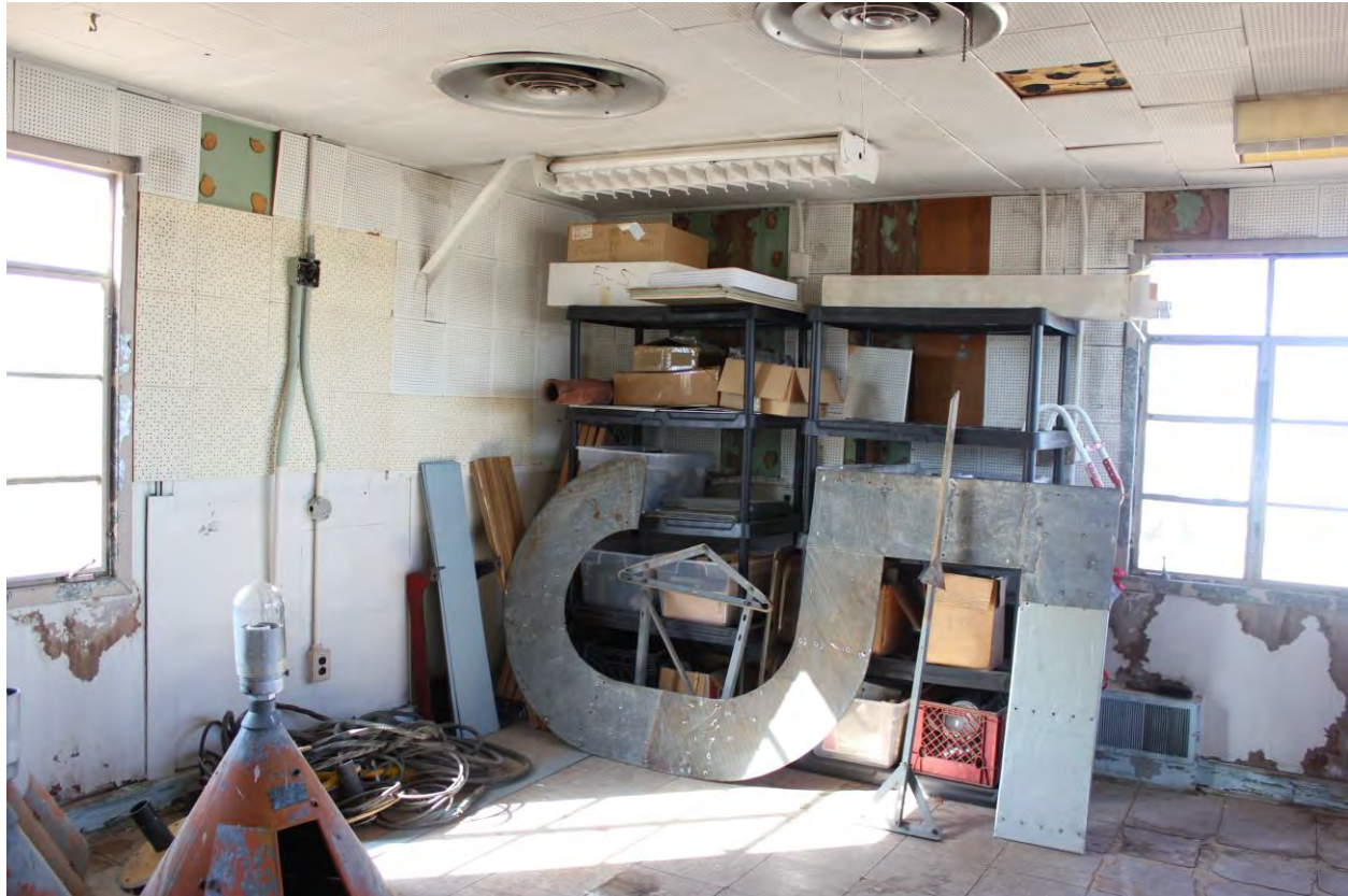
11 of 15. FSS Building, interior, Operations Room, photographer facing southwest.
