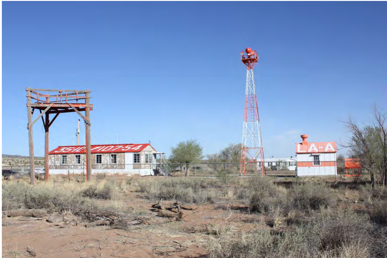
2 of 15. Flight Service Station, with (left to right) delta antenna platform, FSS building, beacon tower, and generator shed, photographer facing northwest.
