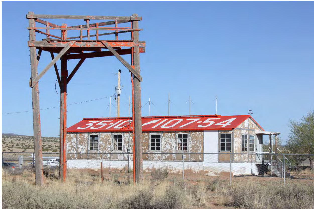
7 of 15. Delta antenna platform and FSS building, south and east sides, photographer facing northwest.
