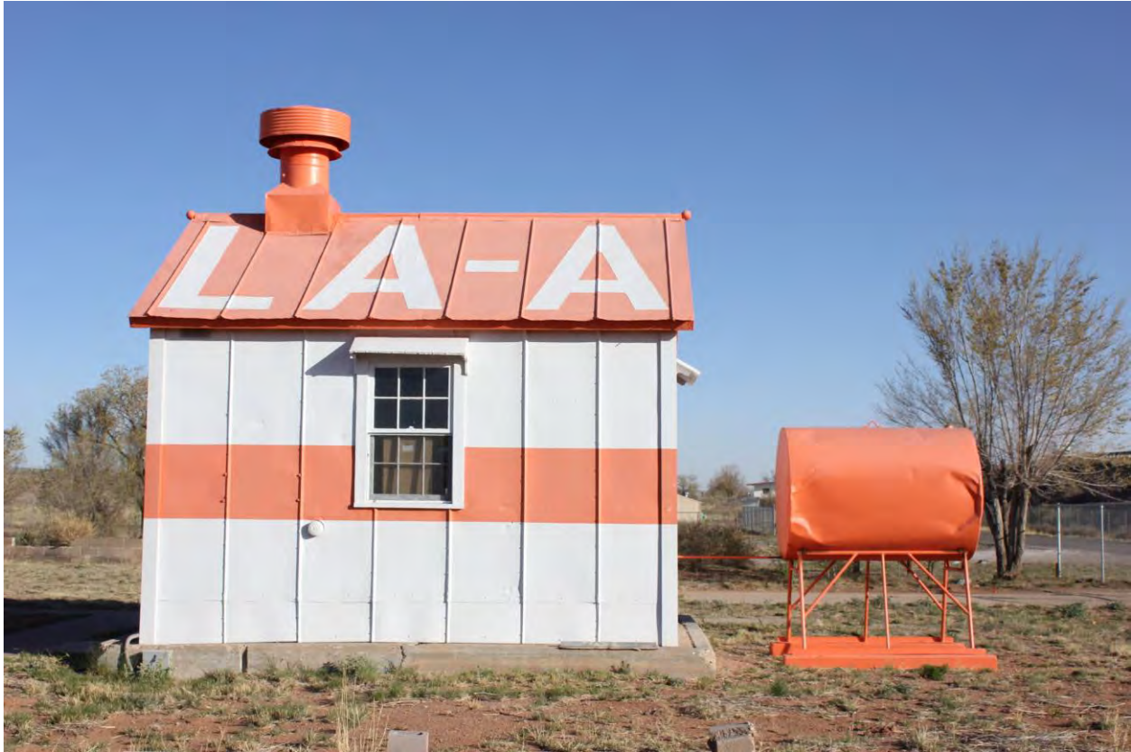
15 of 15. Generator shed, photographer facing north.
