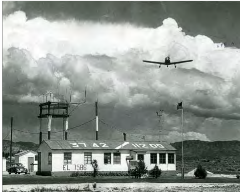
Figure 9. Flight service station, Bryce Canyon, Utah, with Type “S” modular design and delta antenna platform.
