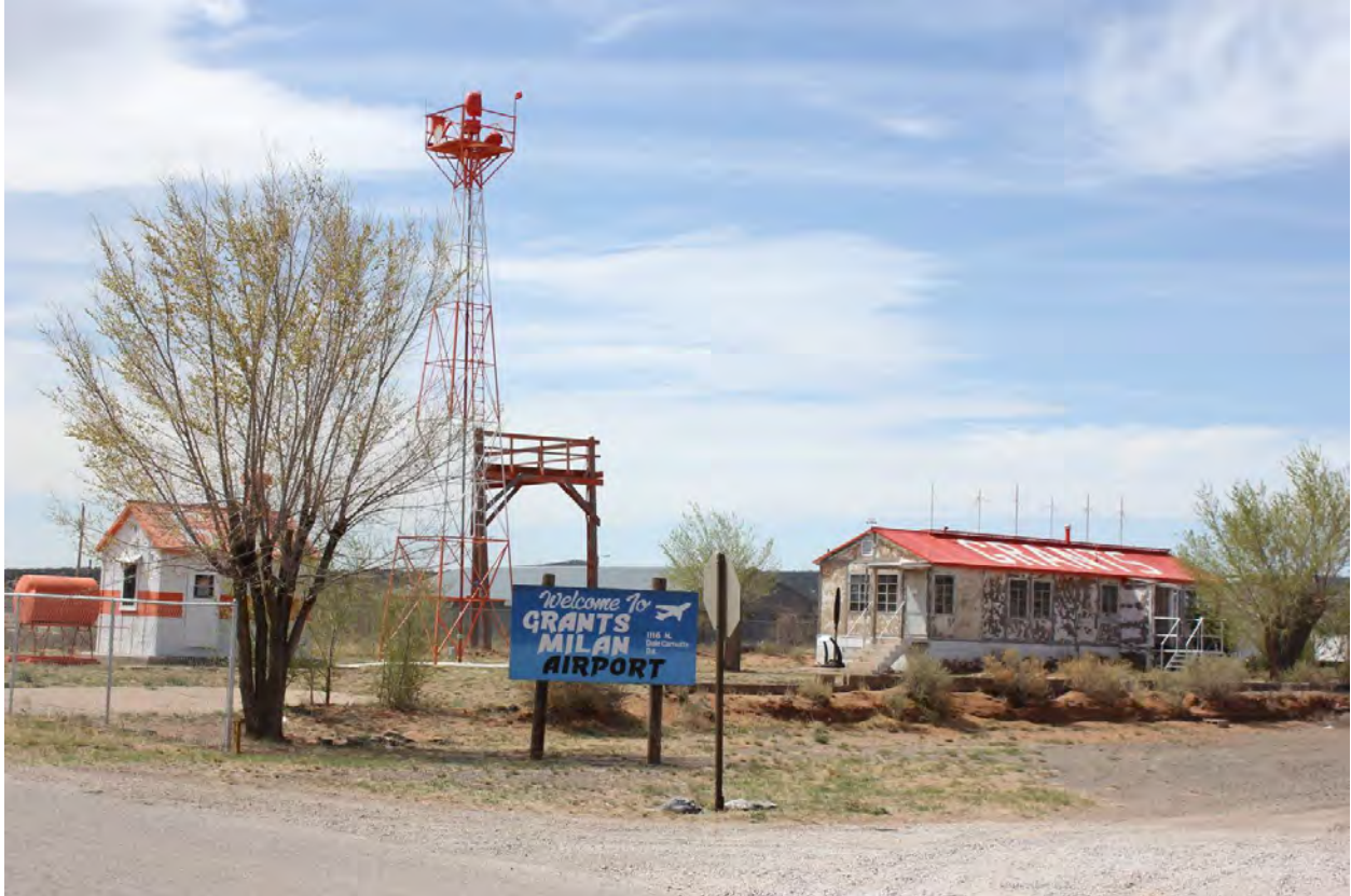
1 of 15. Flight Service Station, with (left to right) generator shed, beacon tower, delta antenna platform, FSS building, photographer facing south.
