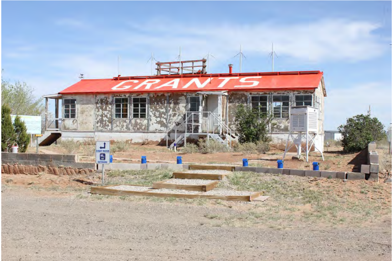
3 of 15. FSS building, north (main) facade, with retaining walls and Stevenson screen enclosure, photographer facing southeast.
