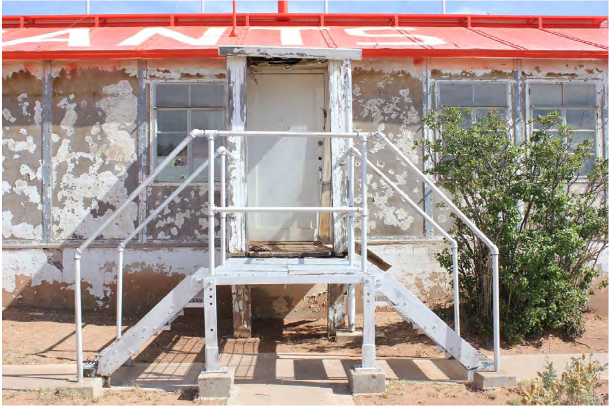
5 of 15. FSS building, main entrance, photographer facing southeast.
