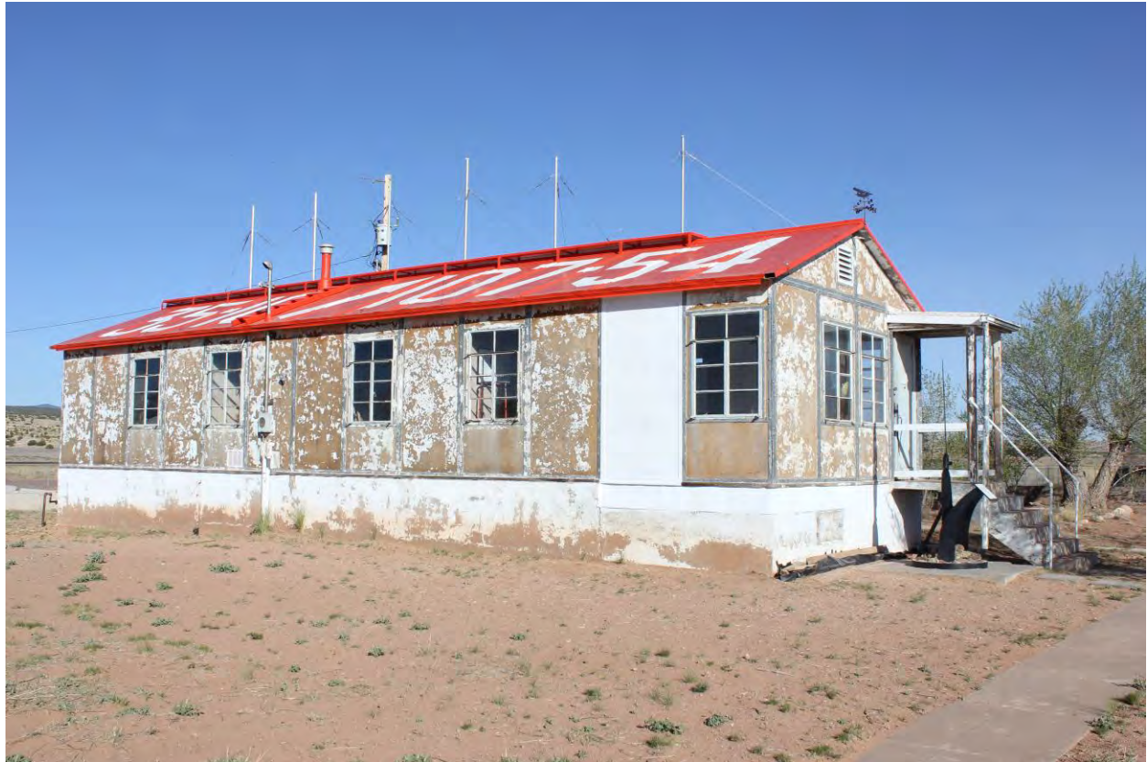
8 of 15. FSS building, south and east sides, photographer facing northwest.
