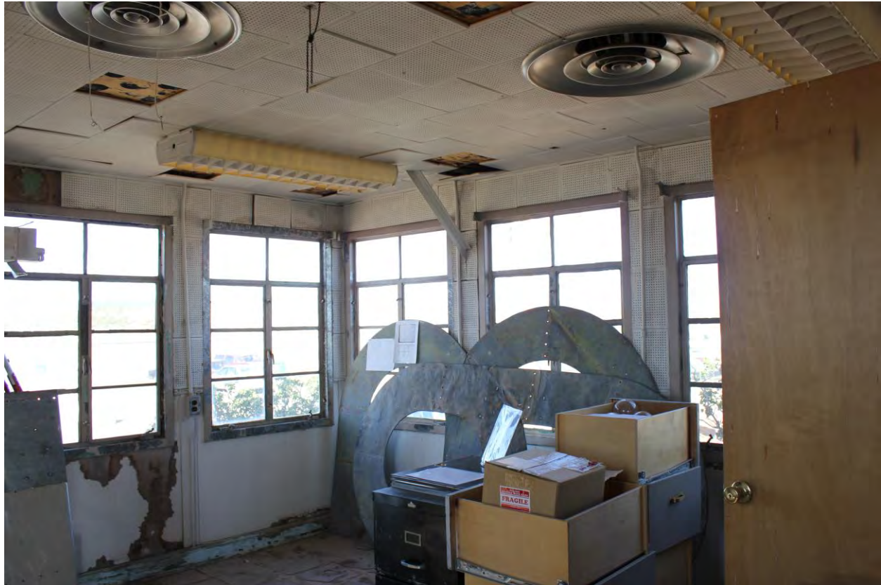
10 of 15. FSS Building, interior, Operations Room, photographer facing northwest.
