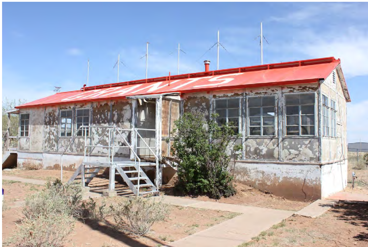
4 of 15. FSS building north and west sides, photographer facing east.
