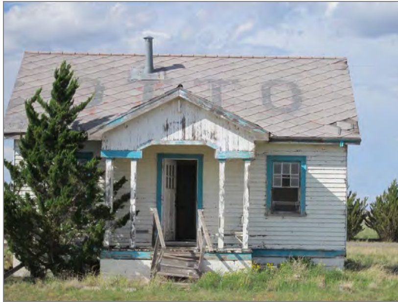
Figure 11. A typical wood-framed Type "K" building
