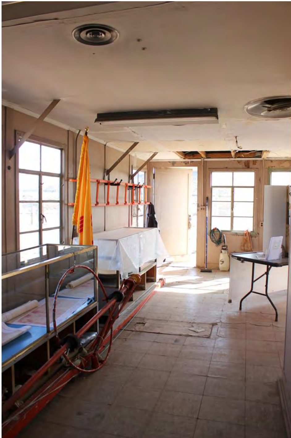
14 of 15. FSS Building, interior, SES office and workshop, photographer facing northeast.
