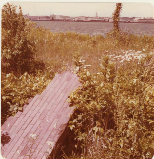
FIG. 14 - CISTERN FRAGMENT: VIEW TO E.
