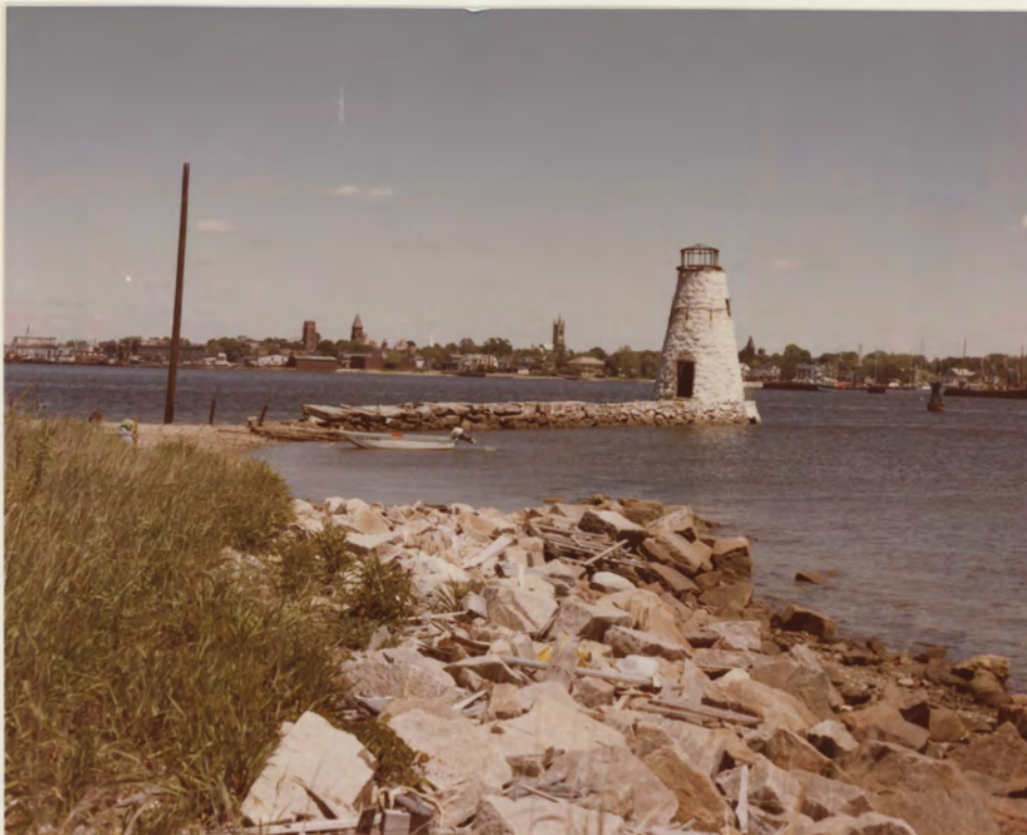
FIG. 9 - EASTERN BEACH, LOOKING N. TOWARD LIGHTHOUSE: SHOWING RIPRAP
