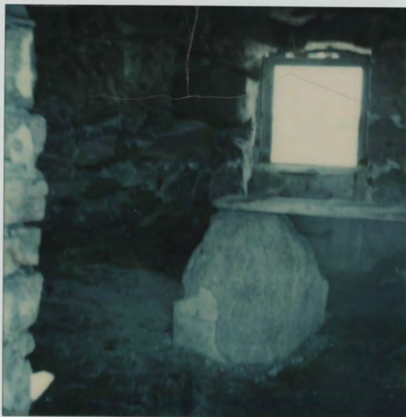
Palmer's Island Light, Station New Bedford, MA. Photog. - Robert Batt, 12 Jun 79 View of lighthouse interior from east doorway.
