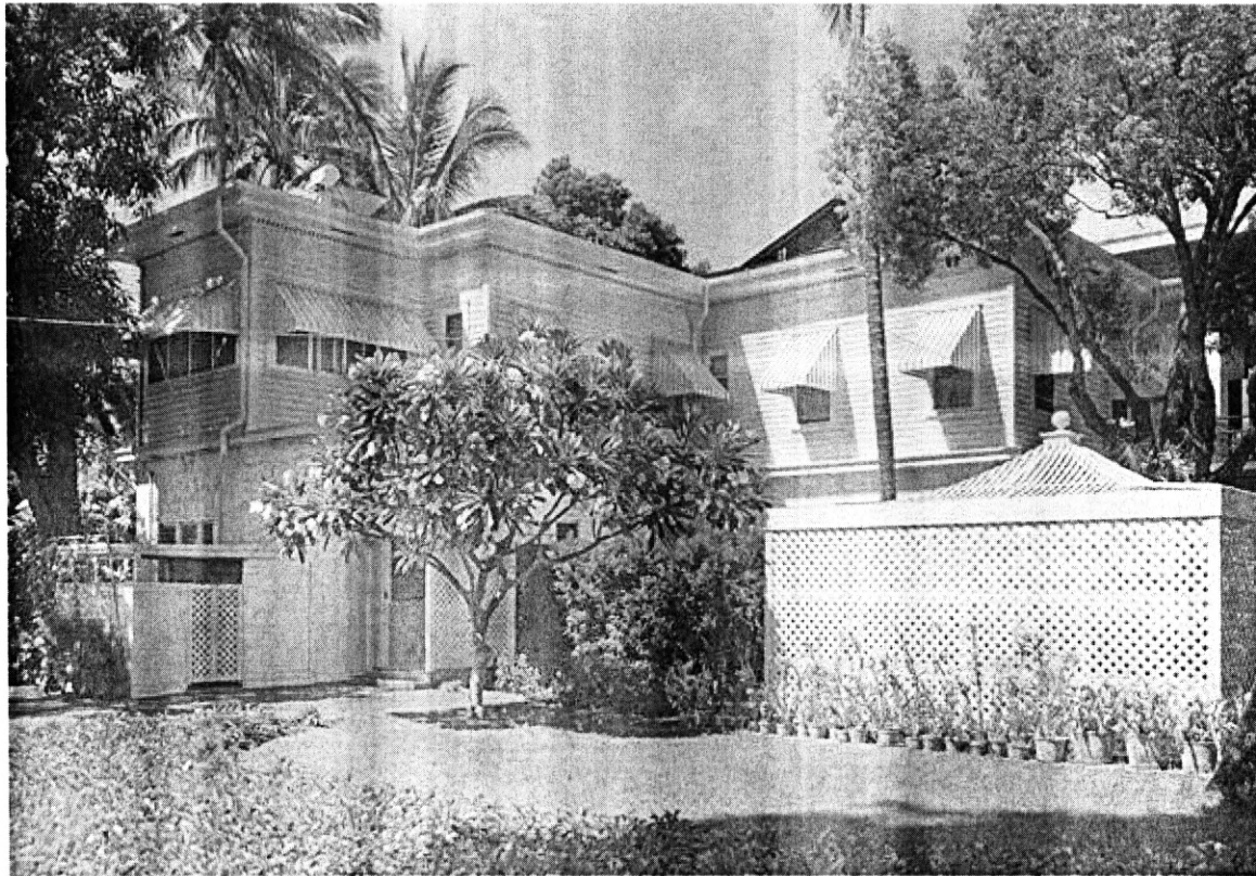
Washington Place, HI. Northeast (rear) Elevation, HABS 1966.
