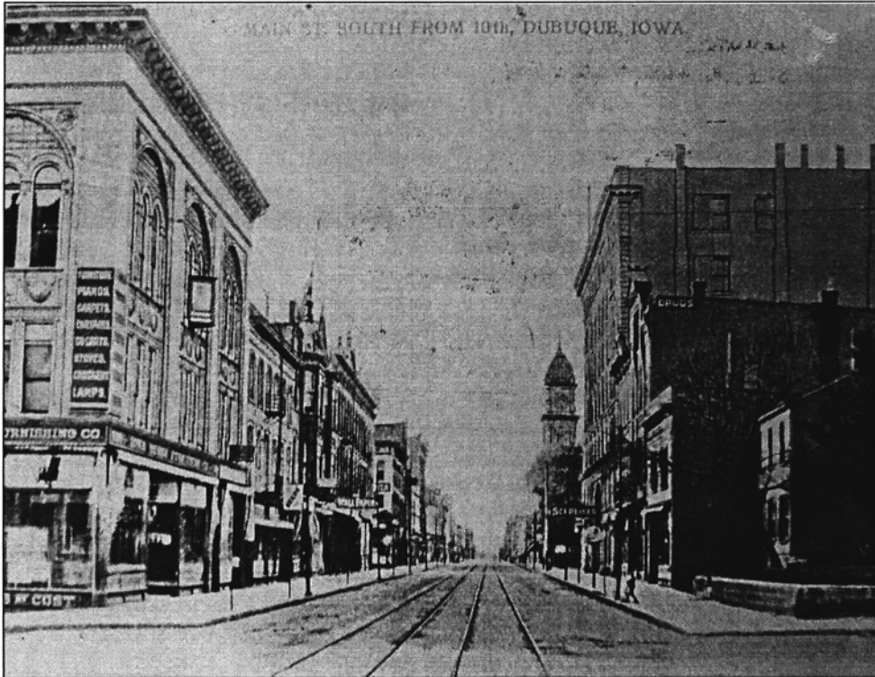
Figure 22: View south along Main from 10 th Street, c.1905 (Loras College, Center For Dubuque History)
