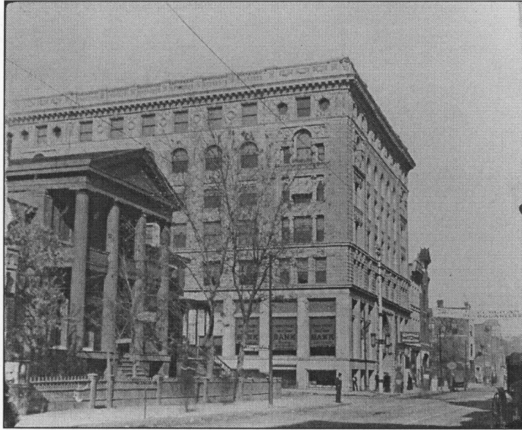
Figure 17: Bank and Insurance Building, view northwest, c.1896 (Dubuque County Historical Society)
