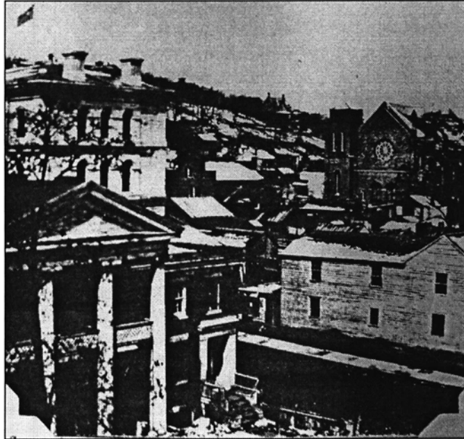
Figure 5: Future Bank and Insurance Building site, view northwest, ca.1890 (Loras College, Center For Dubuque History)
