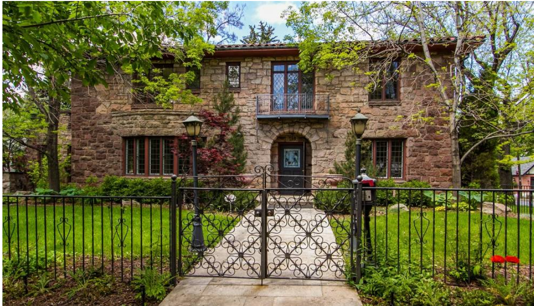
Figure 26: Osmer House, 789 Gaylord Street, Denver, ca. 2018. Tulia.com
