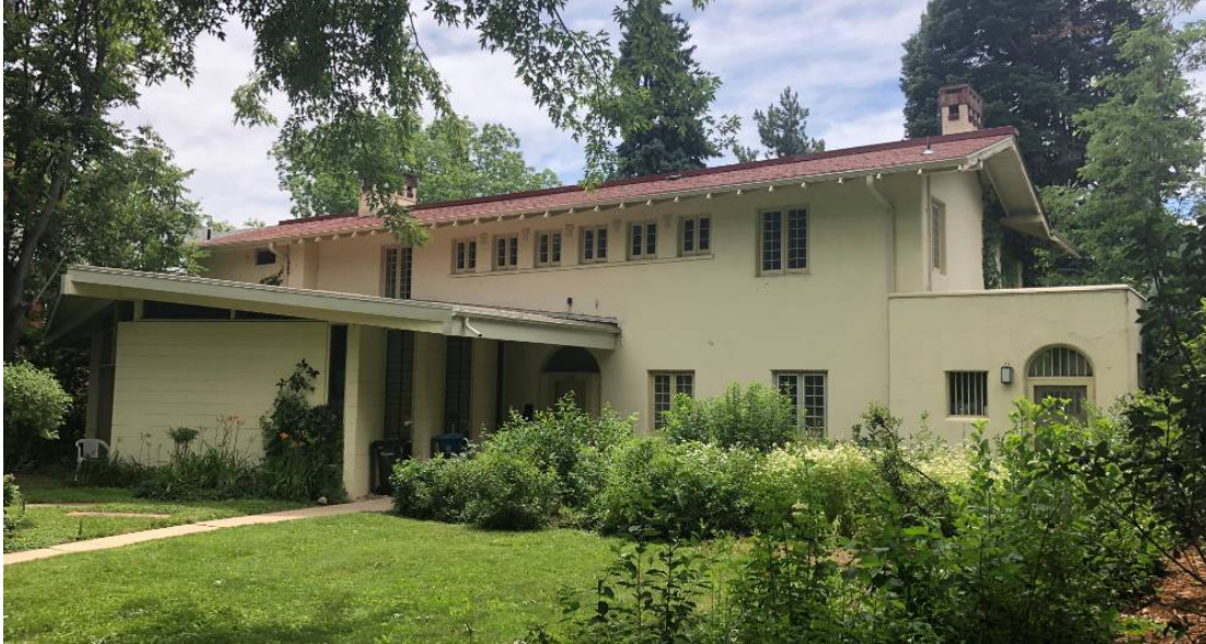
Figure 28: 570 Highland Avenue, Boulder. Photo by Amy Unger.
