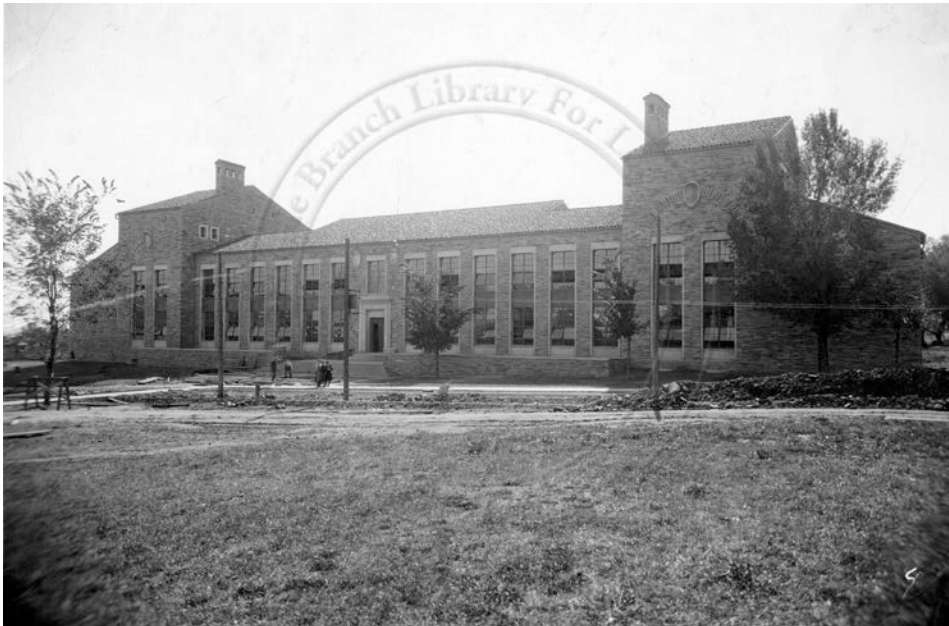
Figure 2: The 1921 Helms Arts and Sciences Building was the first University of Colorado building designed by Charles Klauder in the "Colorado Style" after adoption of Klauder's campus master plan in 1918. Photograph dated May 1922. Boulder Historical Society Collection, Carnegie Library for Local History, BHS 240-2-30.
