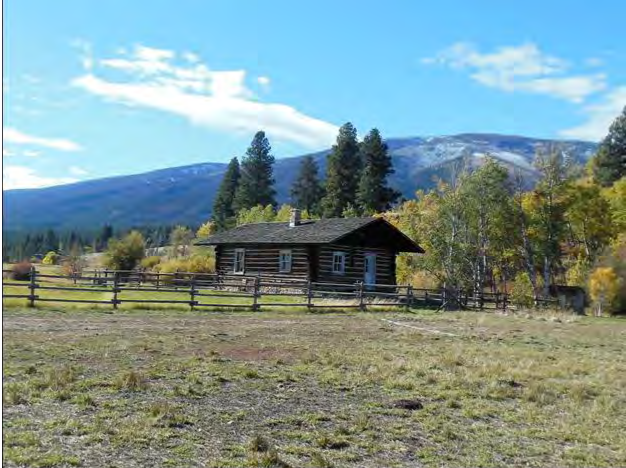
East and north elevations. Looking west. Ward Mountain in background. MT_RavalliCounty_JamesMcCrossinCabin_Photo 0002.
