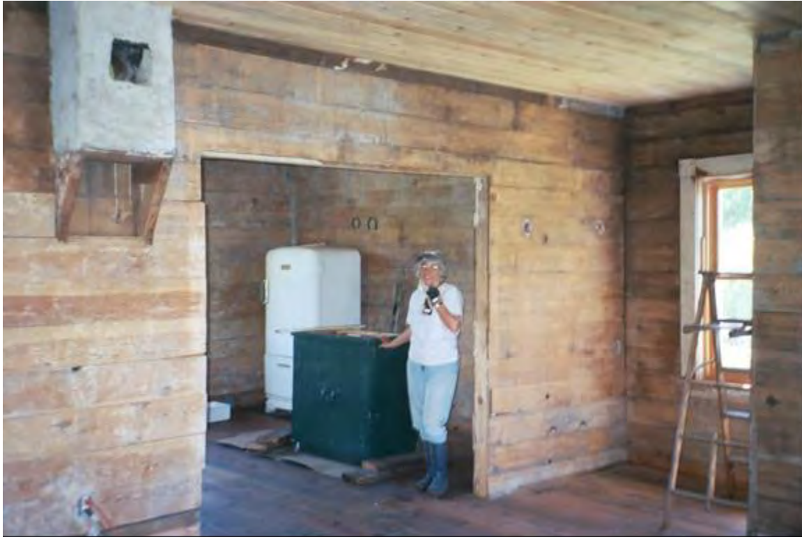
Interior of the James McCrossin Cabin during restoration.
