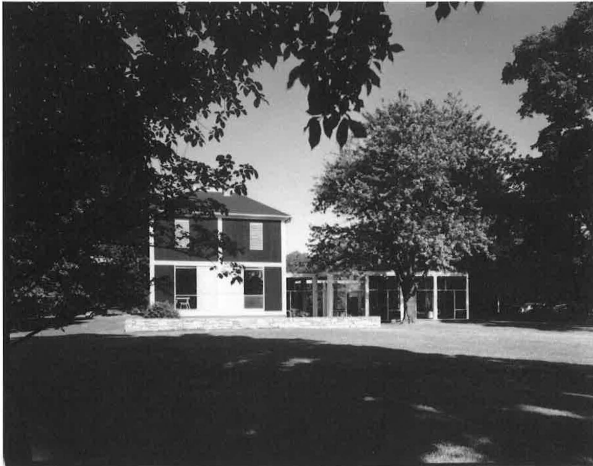
1 of 11: The Charles M. Goodman House, ca. 1954, showing the eastern façade. The original farmhouse (left) was constructed between 1873 and 1879. Goodman remodeled the house and added a glass pavilion (right) to the house between 1953 and 1954. From the Robert C. Lautman Photography Collection, box 33, courtesy of the National Building Museum, Washington, D.C.
