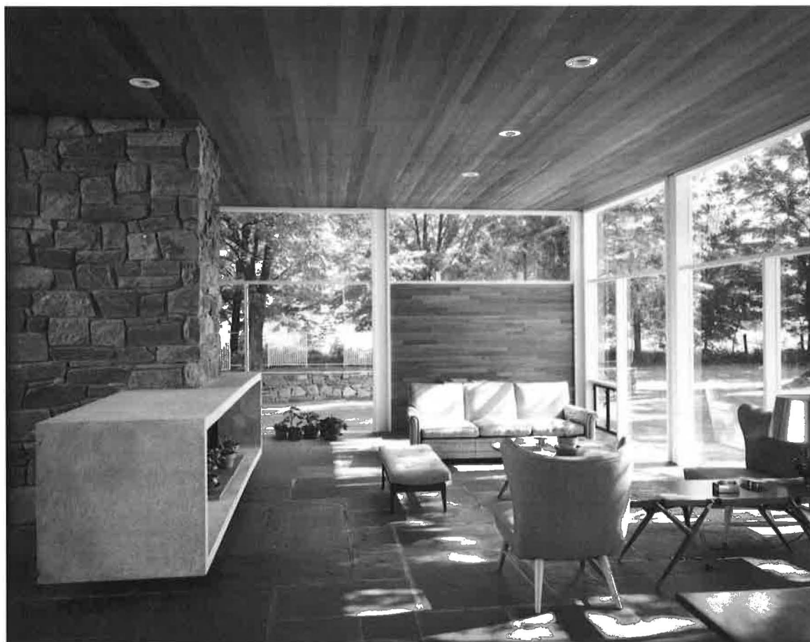
9 of 11: The glass enclosed living room of the Goodman addition, ca. 1954. Visible here are the cantilevered concrete fireplace, stone chimney, wood paneled ceiling, and flagstone floors with radiant heating. While most of the prefabricated panels were filled with plate glass, some like the panel above were filled with wood paneling. The bench is a Jens Risom piece. From the Robert C. Lautman Photography Collection, box 35, courtesy of the National Building Museum, Washington, D.C.
