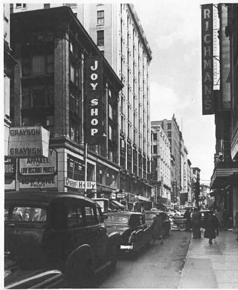
Figure 3: Blake and Amory Building, Looking East along Washington Street c. 1955
