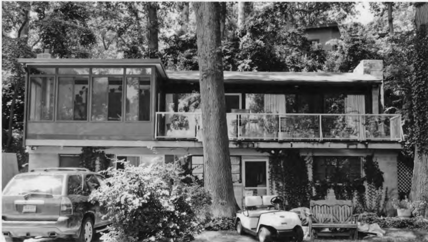
Photo 17. 28 Dock Road. Norwalk, Fairfield County, Connecticut View west, July 14, 2009, Tod Bryant
