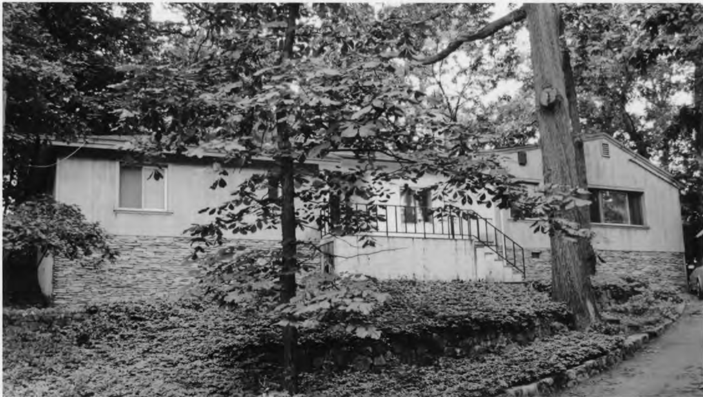
Photo 6. 9 Dock Road. Norwalk, Fairfield County, Connecticut View northeast, July 14, 2009, Tod Bryant
