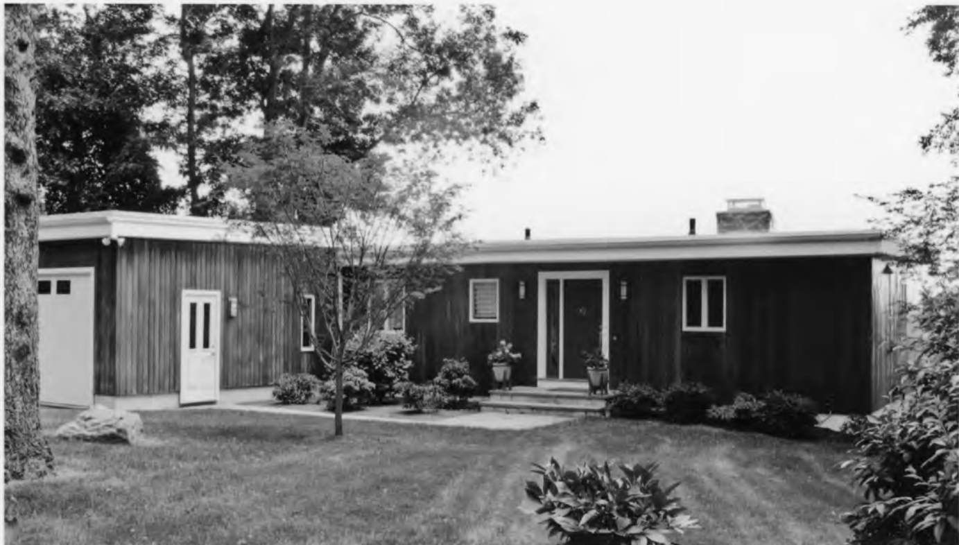
Photo 11. 17 Dock Road. Norwalk, Fairfield County, Connecticut View northeast, July 14, 2009, Tod Bryant
