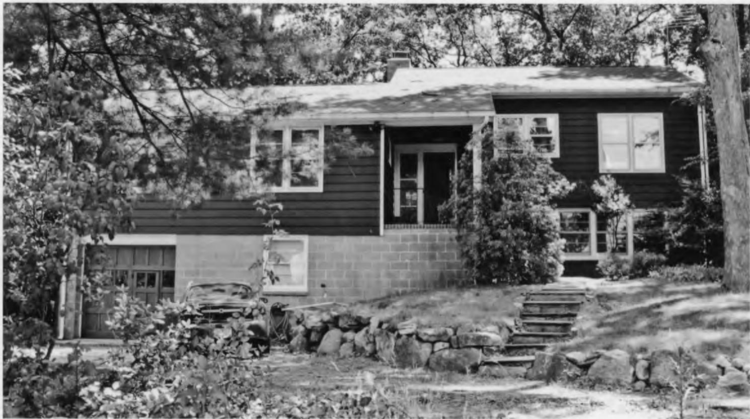
Photo 1. 1 Dock Road. Norwalk, Fairfield County, Connecticut View east, July 14, 2009, Tod Bryant
