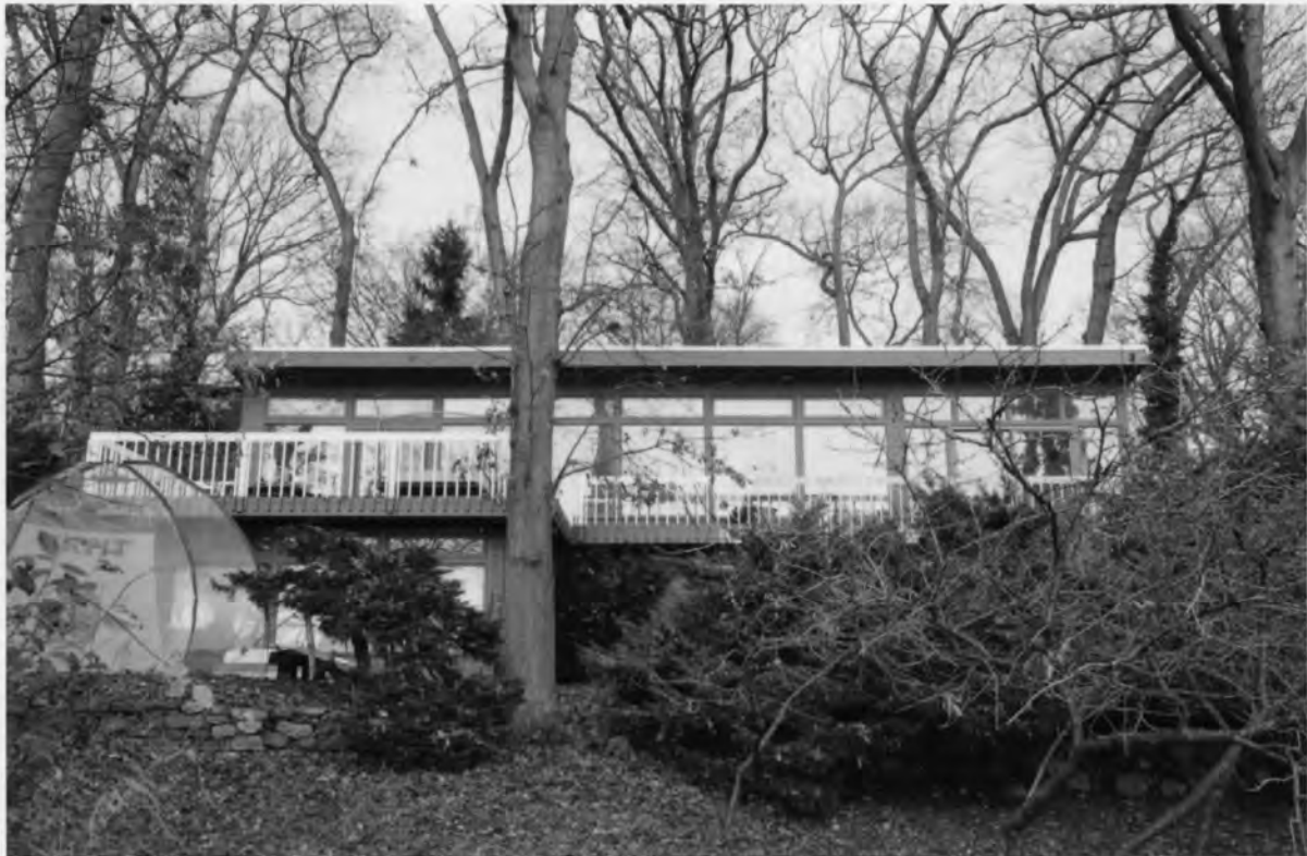
Photo 19. 32 Dock Road. Norwalk, Fairfield County, Connecticut View west, July 14, 2009, Tod Bryant
