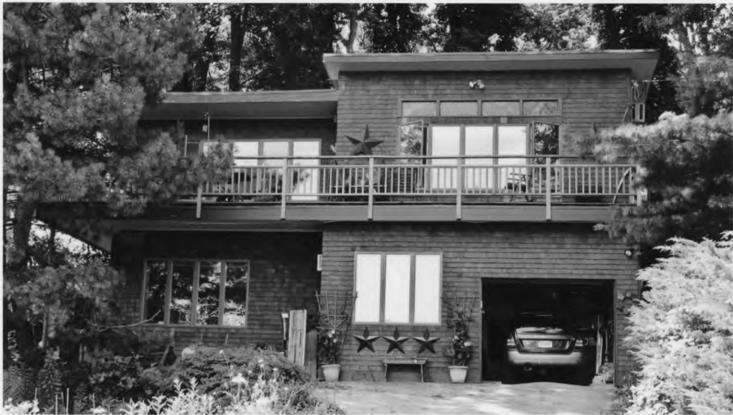
Photo 15. 24 Dock Road. Norwalk, Fairfield County, Connecticut View west, July 14, 2009, Tod Bryant
