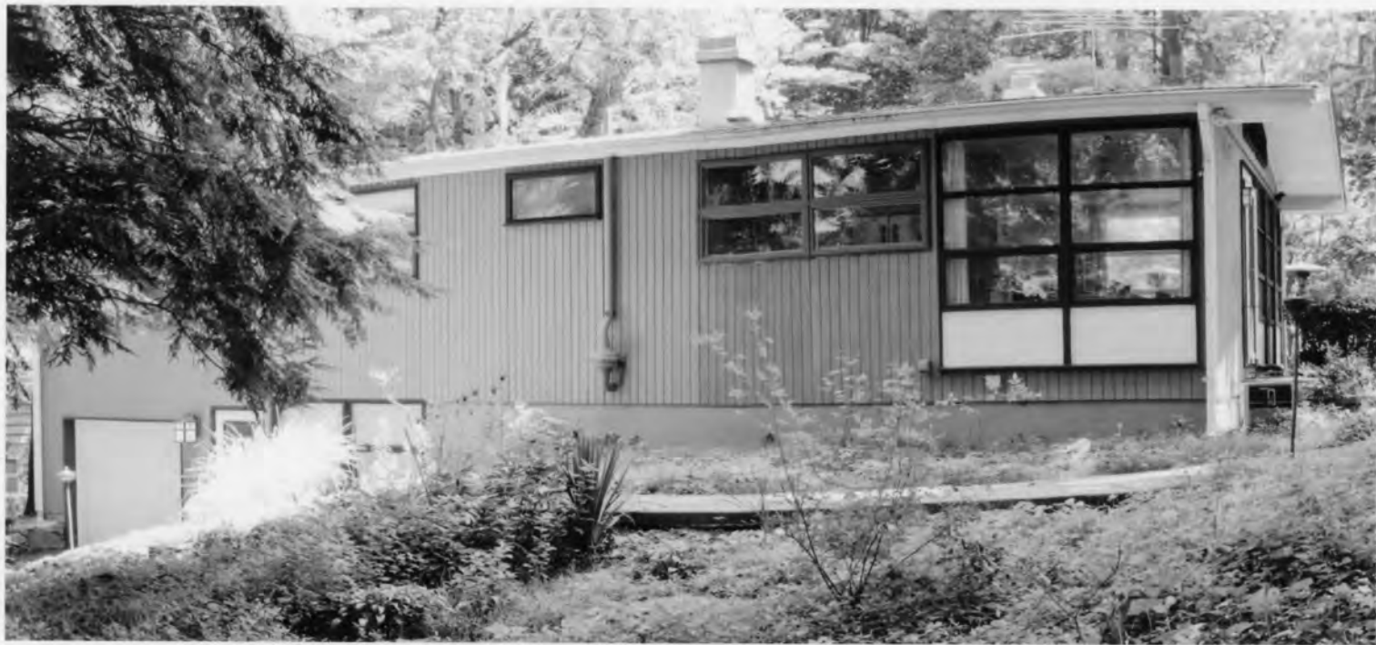
Photo 39. 17 Split Rock Road, Norwalk, Fairfield County, Connecticut View northeast, July 14, 2009, Tod Bryant
