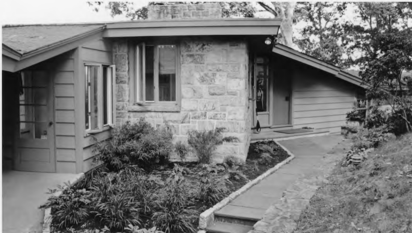
Photo 24. 9 Outer Road. Norwalk, Fairfield County, Connecticut View east, July 14, 2009, Tod Bryant
