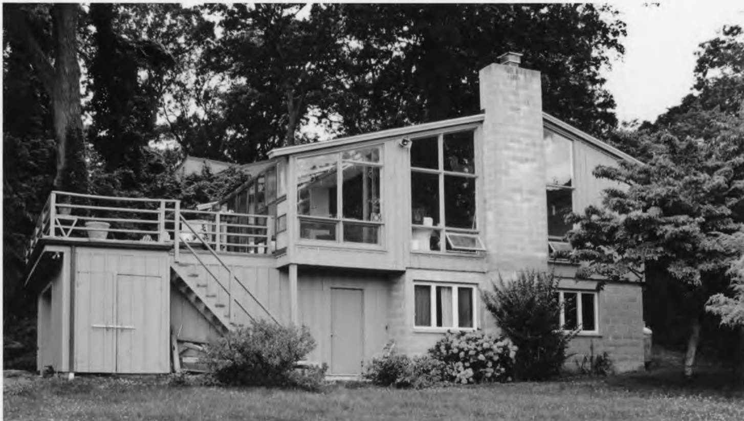
Photo 14. 22 Dock Road. Norwalk, Fairfield County, Connecticut View northeast, July 14, 2009, Tod Bryant
