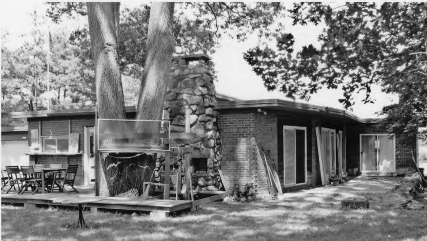
Photo 22. 3 Outer Road. Norwalk, Fairfield County, Connecticut View northeast, July 14, 2009, Tod Bryant
