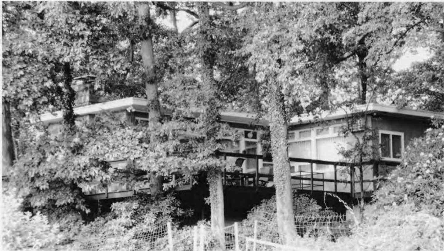
Photo 27. 10 Outer Road. Norwalk, Fairfield County, Connecticut View northeast, July 14, 2009, Tod Bryant
