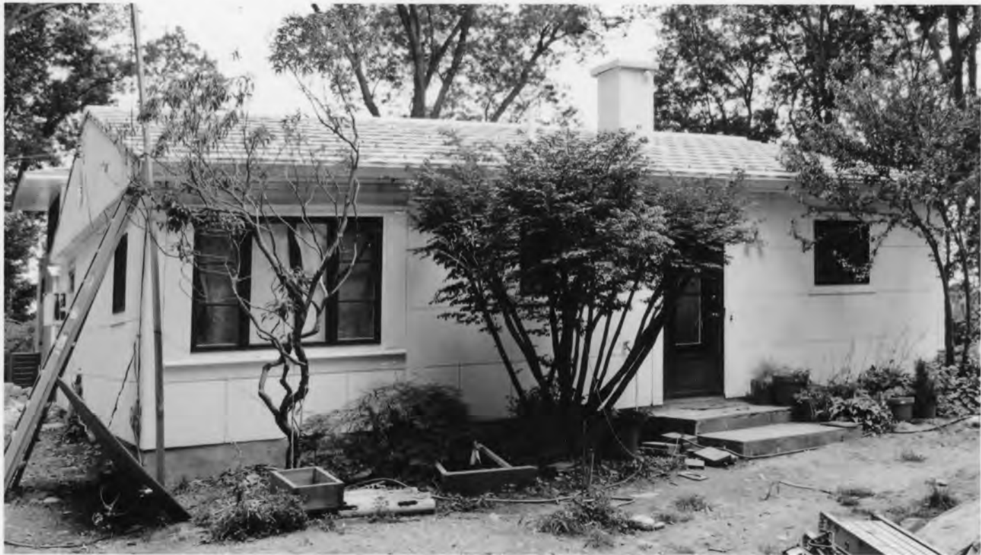
Photo 9. 13 Dock Road. Norwalk, Fairfield County, Connecticut View east, July 14, 2009, Tod Bryant
