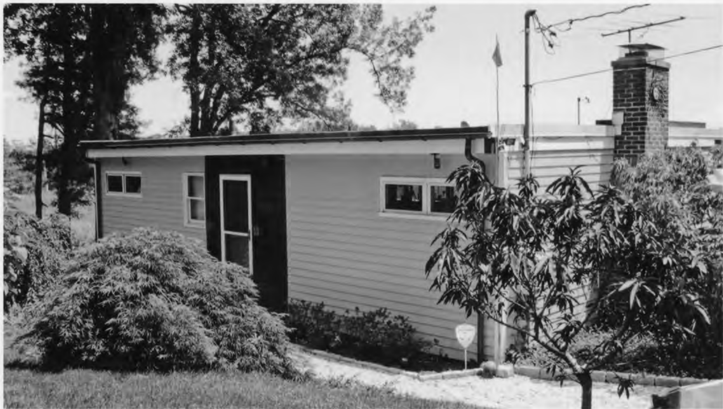
Photo 10. 15 Dock Road. Norwalk, Fairfield County, Connecticut View northeast, July 14, 2009, Tod Bryant
