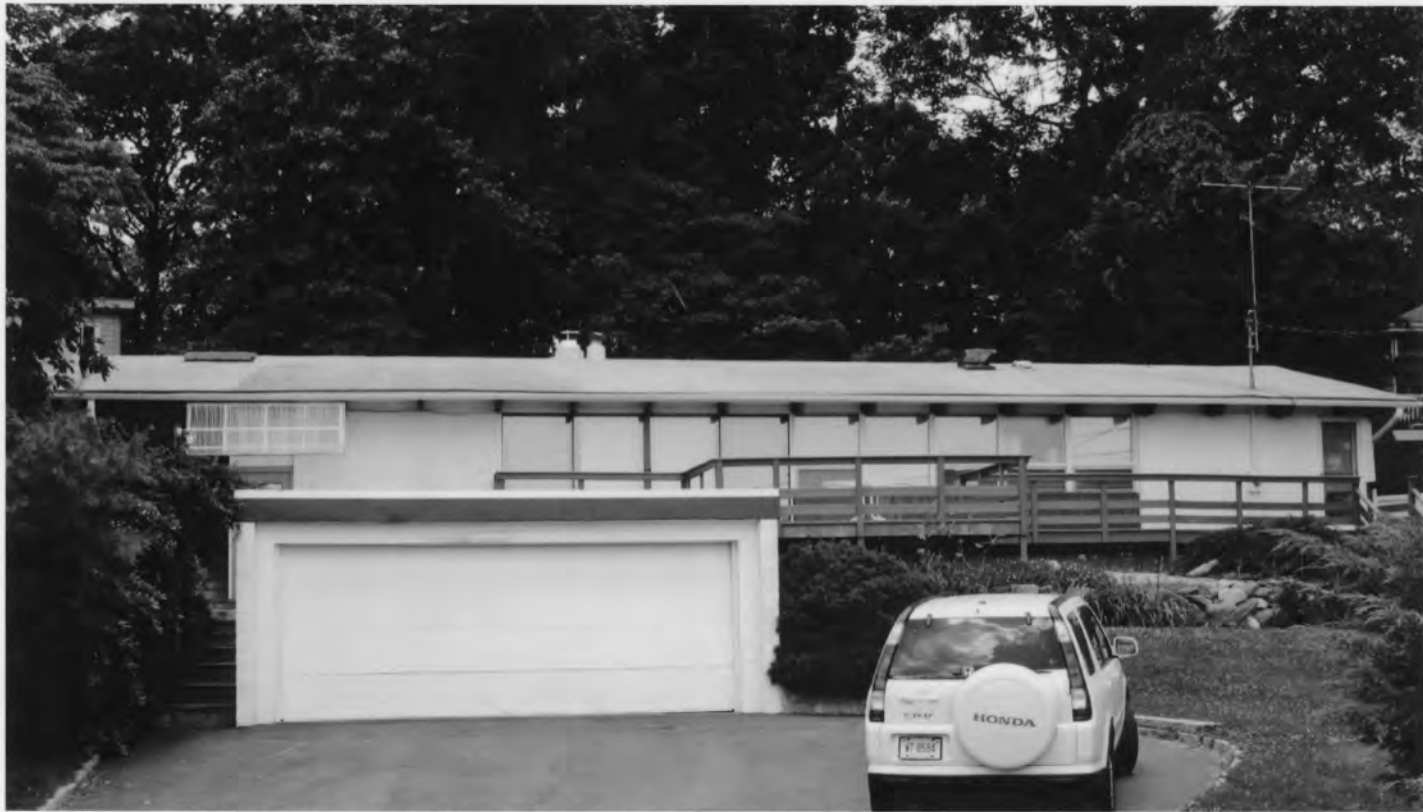
Photo 13. 20 Dock Road. Norwalk, Fairfield County, Connecticut View west July 14, 2009, Tod Bryant
