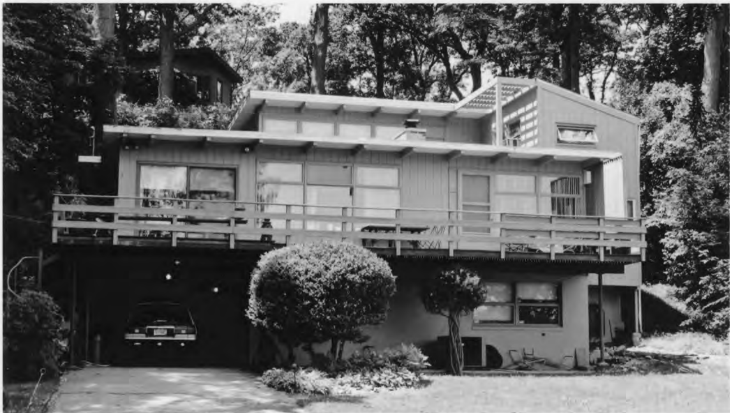
Photo 16. 26 Dock Road. Norwalk, Fairfield County, Connecticut View west, July 14, 2009, Tod Bryant
