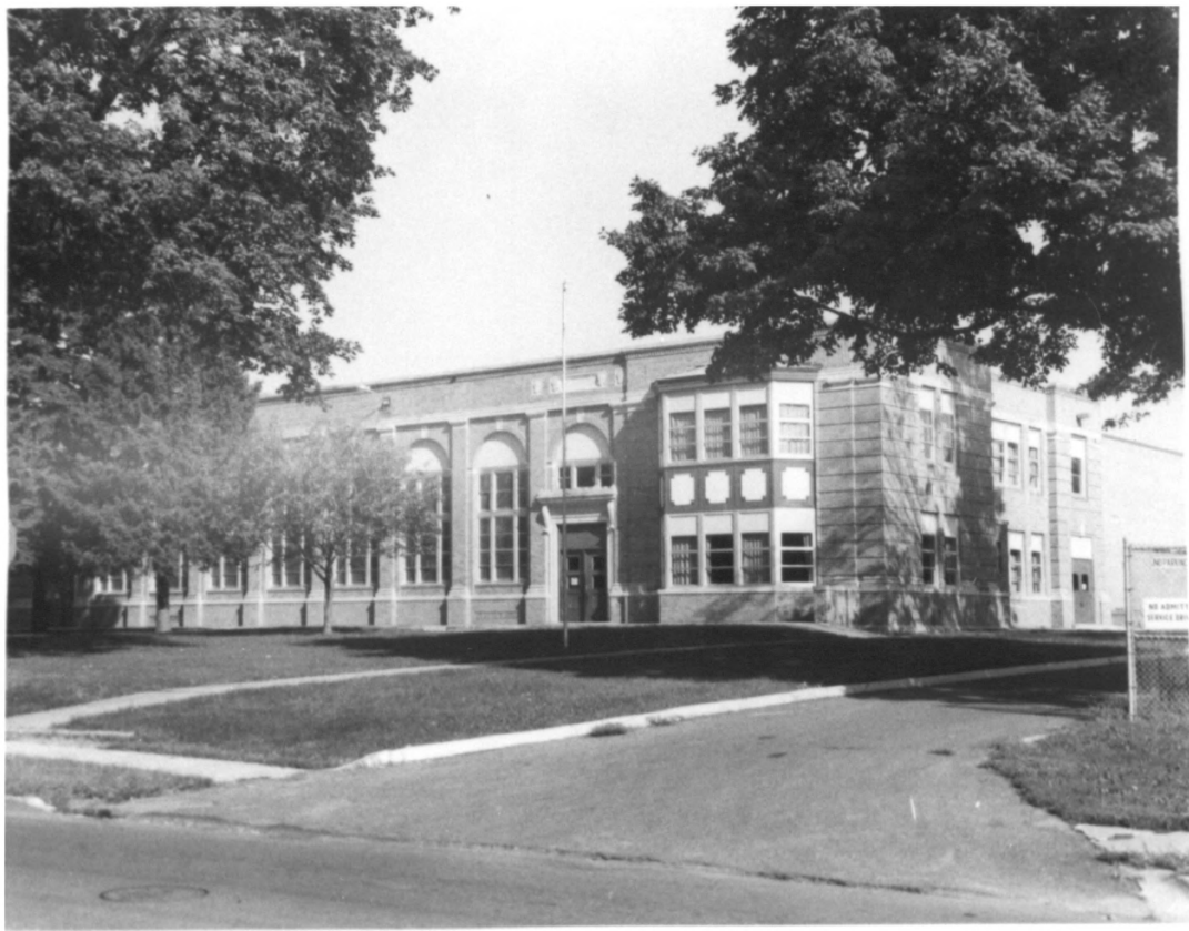
5. EMERSON HOUGH ELEMENTARY SCHOOL : NEWTON, MA
