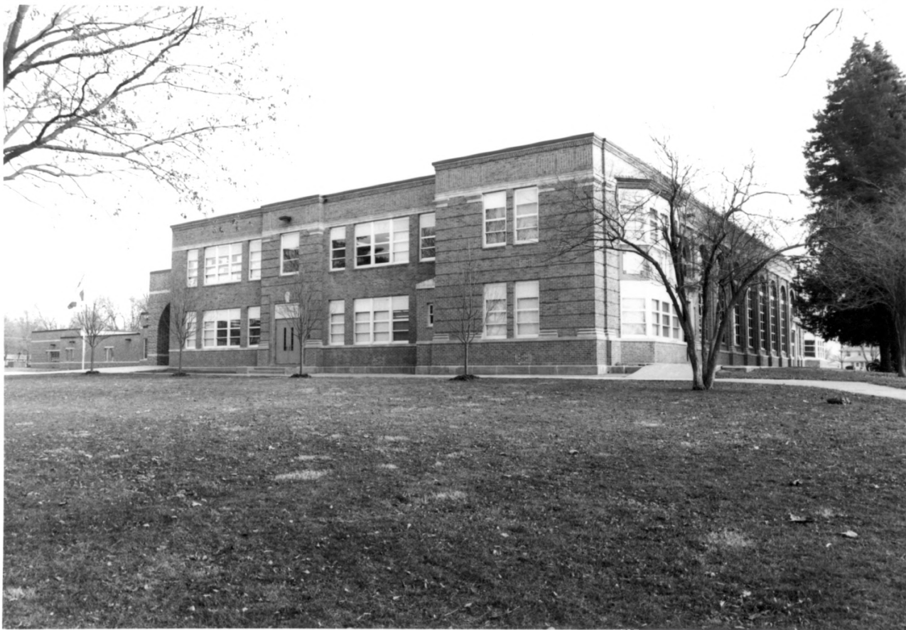
Z. EMERSON HOUGH ELEMENTARY SCHOOL : NEWTON, IA
