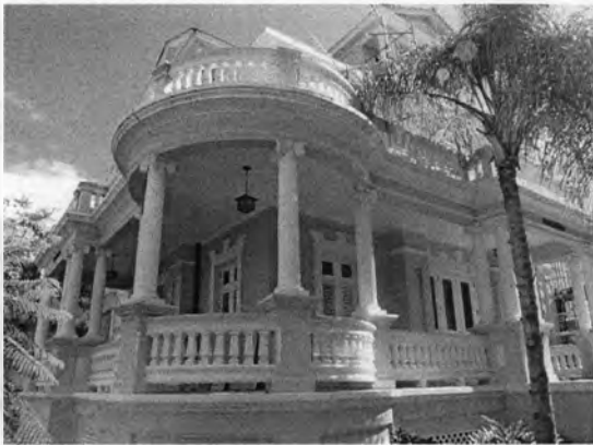
Fig. 5. Partial view of balcony
