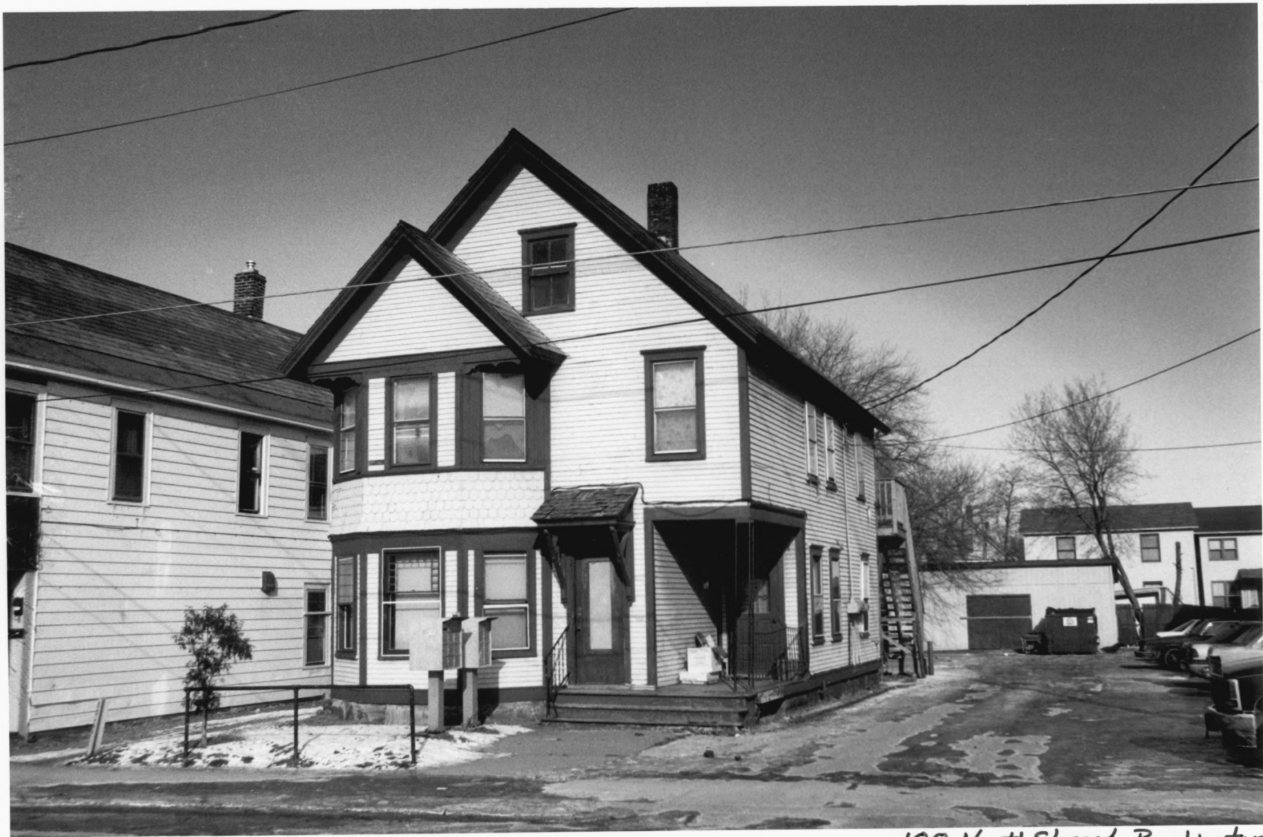
188 North Street, Burlington North Street Historic District Chittenden, Vermont #64 County
