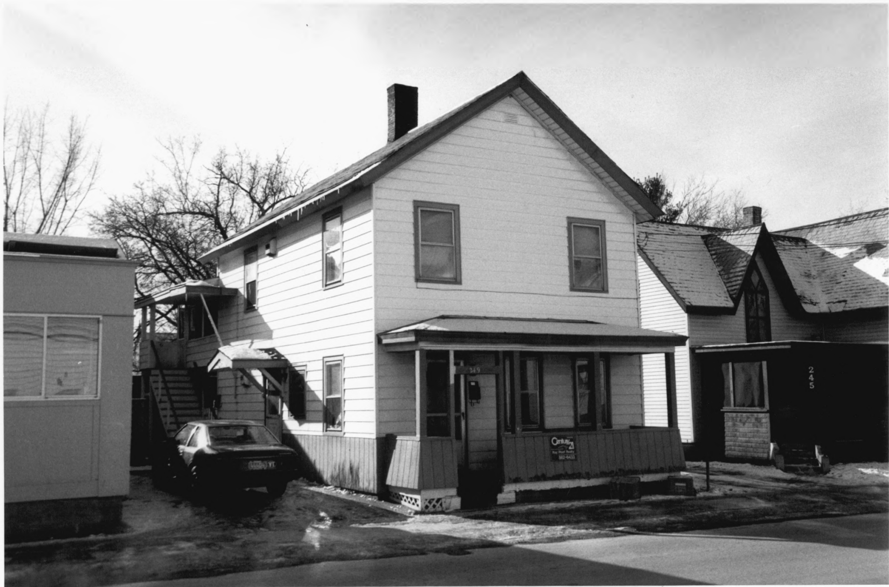
249 North Street, Burlington North Street Historic District Chittenden, Vermont #85 COUNTY
