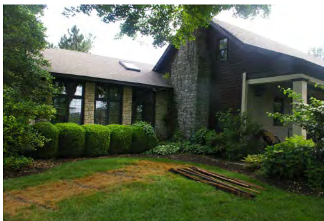
Looking east at west side. Historic portion at Right.
