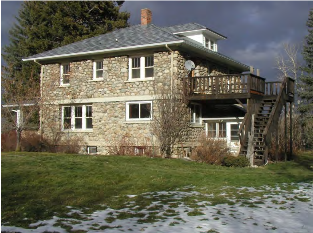
Description and view of camera: South and East elevation, view to northwest Photograph: MT_StillwaterCounty_CharlesGladysPeltonHouse_0005
