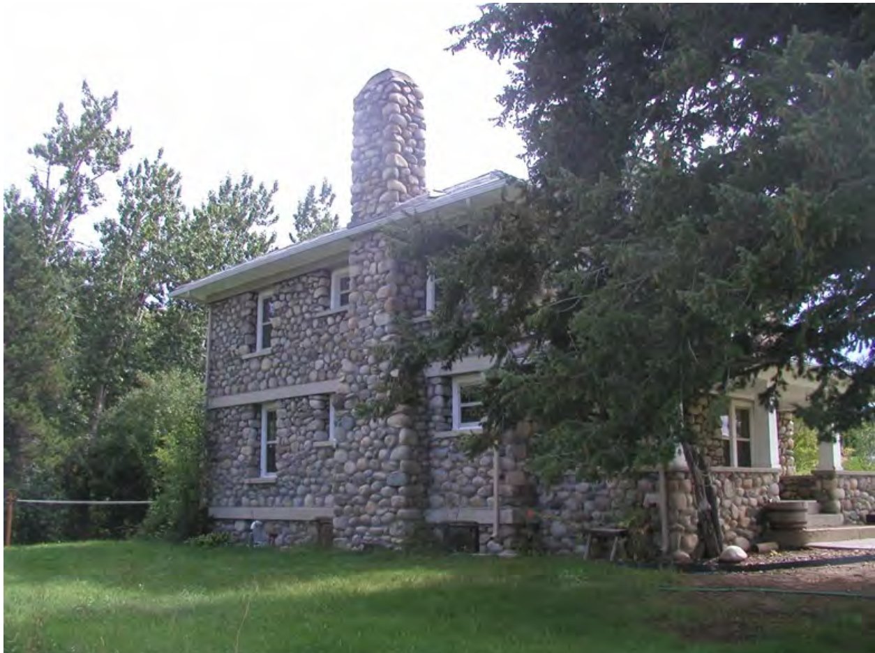
Description and view of camera: North and West elevation, view to southeast Photograph: MT_StillwaterCounty_CharlesGladysPeltonHouse_0003
