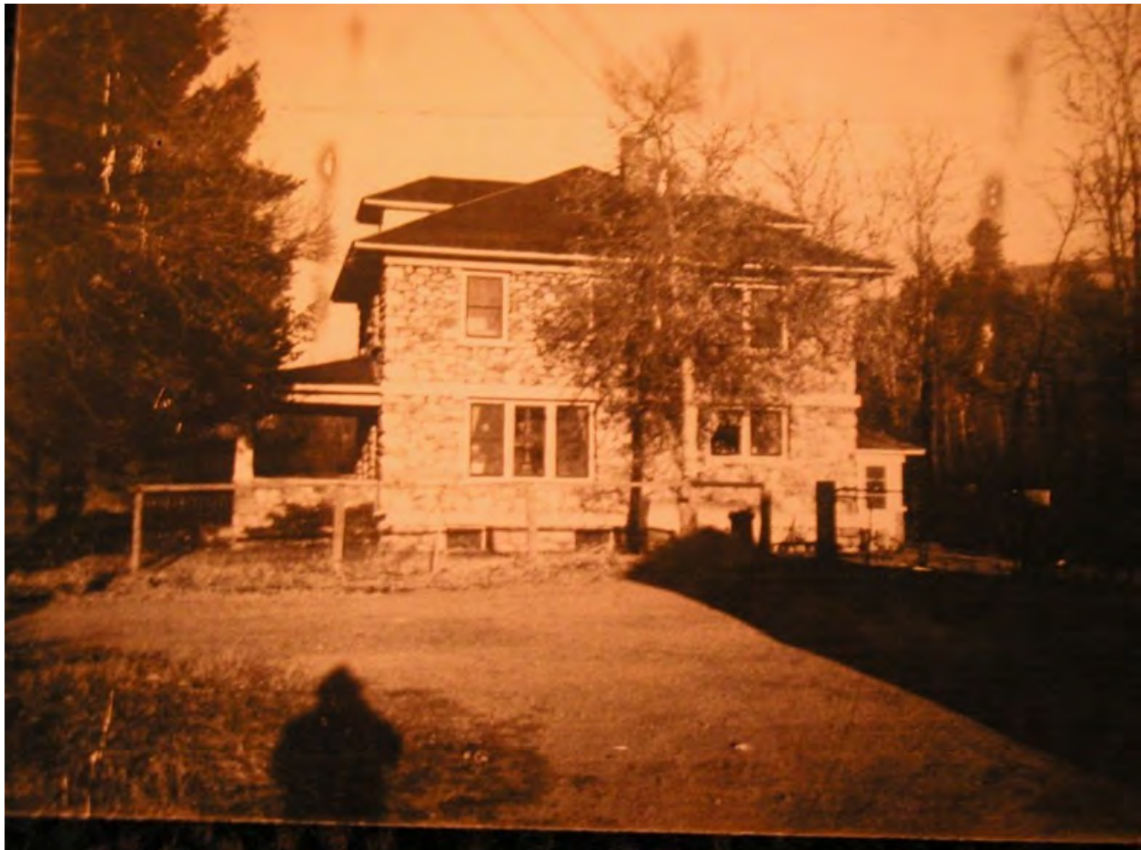
South Side of Pelton House, view to north, 1976 Photograph: MT_StillwaterCounty_CharlesGladysPeltonHouse_0012
