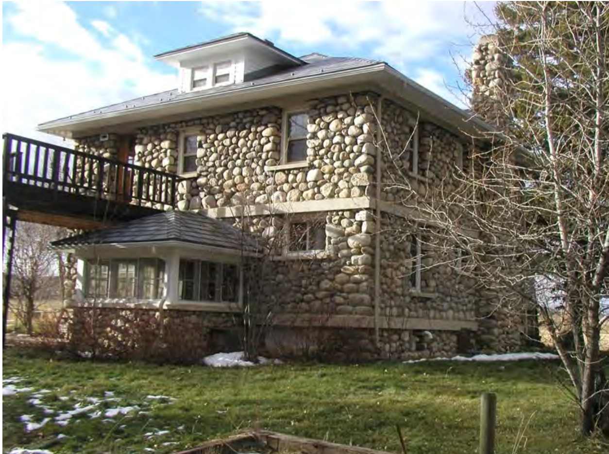
Description and view of camera: North and East elevations, view to southwest Photograph: MT_StillwaterCounty_CharlesGladysPeltonHouse_0004
