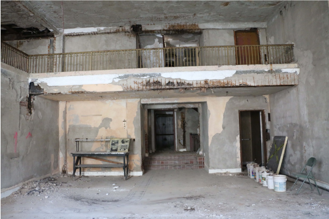
Hotel lobby looking south, 2015
