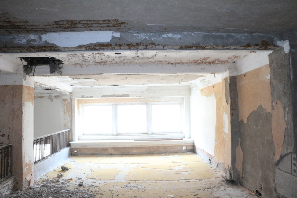
Mezzanine looking north, 2015
