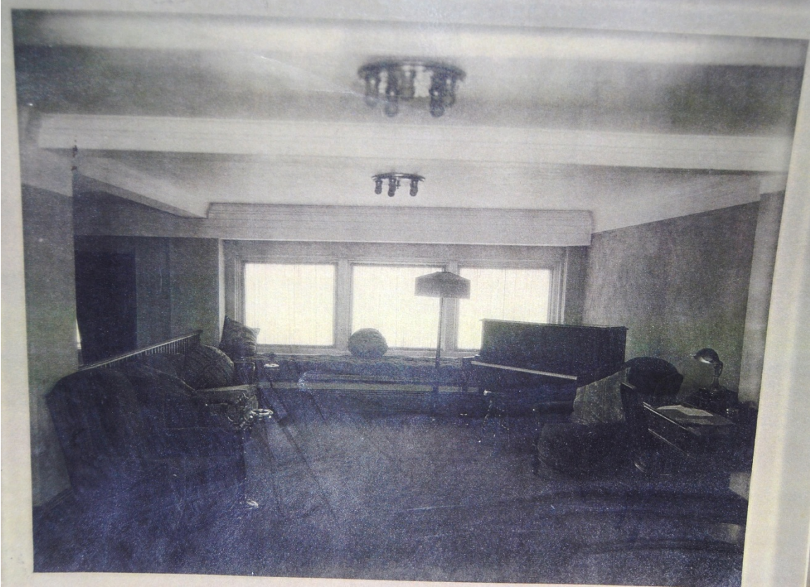
Figure 3.4 Mezzanine looking north, ca. 1926
