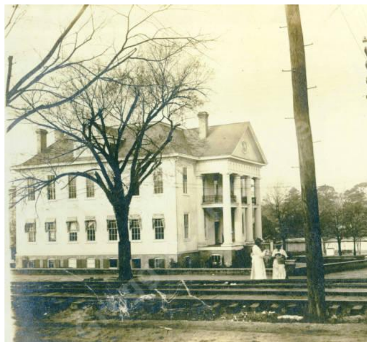
Figure 4: Hickman Memorial Hall, c. 1910 (Gregg-Graniteville Photographic Archive, Gregg-Graniteville Library, Univ. of South Carolina, Aiken)
