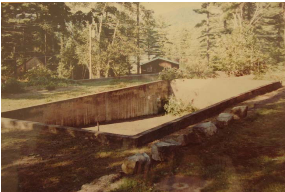
View of unused swimming pool, ca. 1950, in collection of Daniel Slovak
