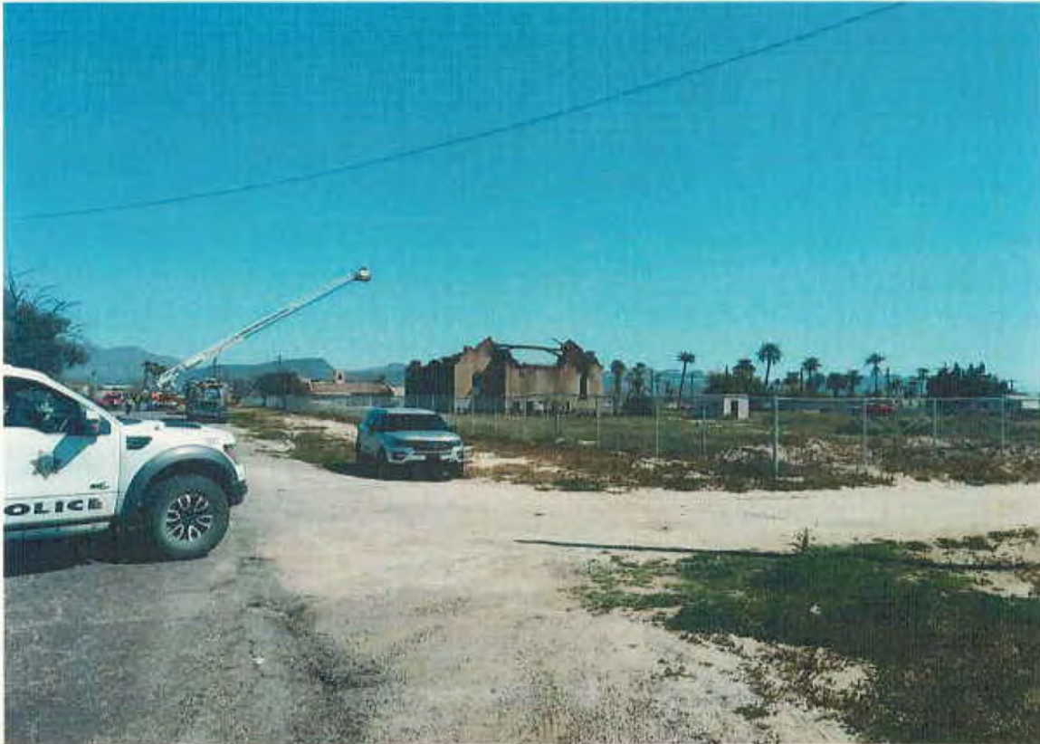
Figure 3. C.H. Cook Memorial Church after the front roof vault has collapsed March 25, 2019.
