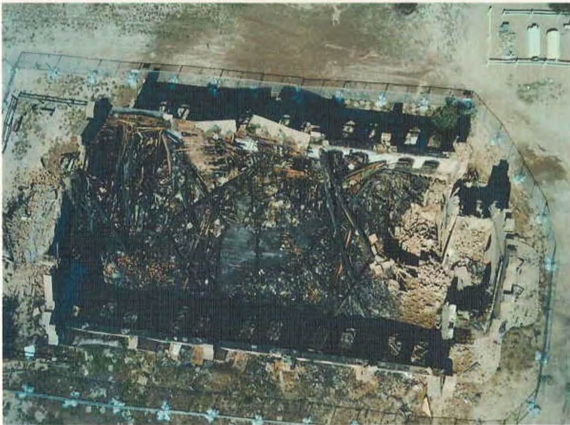
Figure 6. Overhead View of C.H. Cook Memorial Church Drone Photo March 28, 2019.
