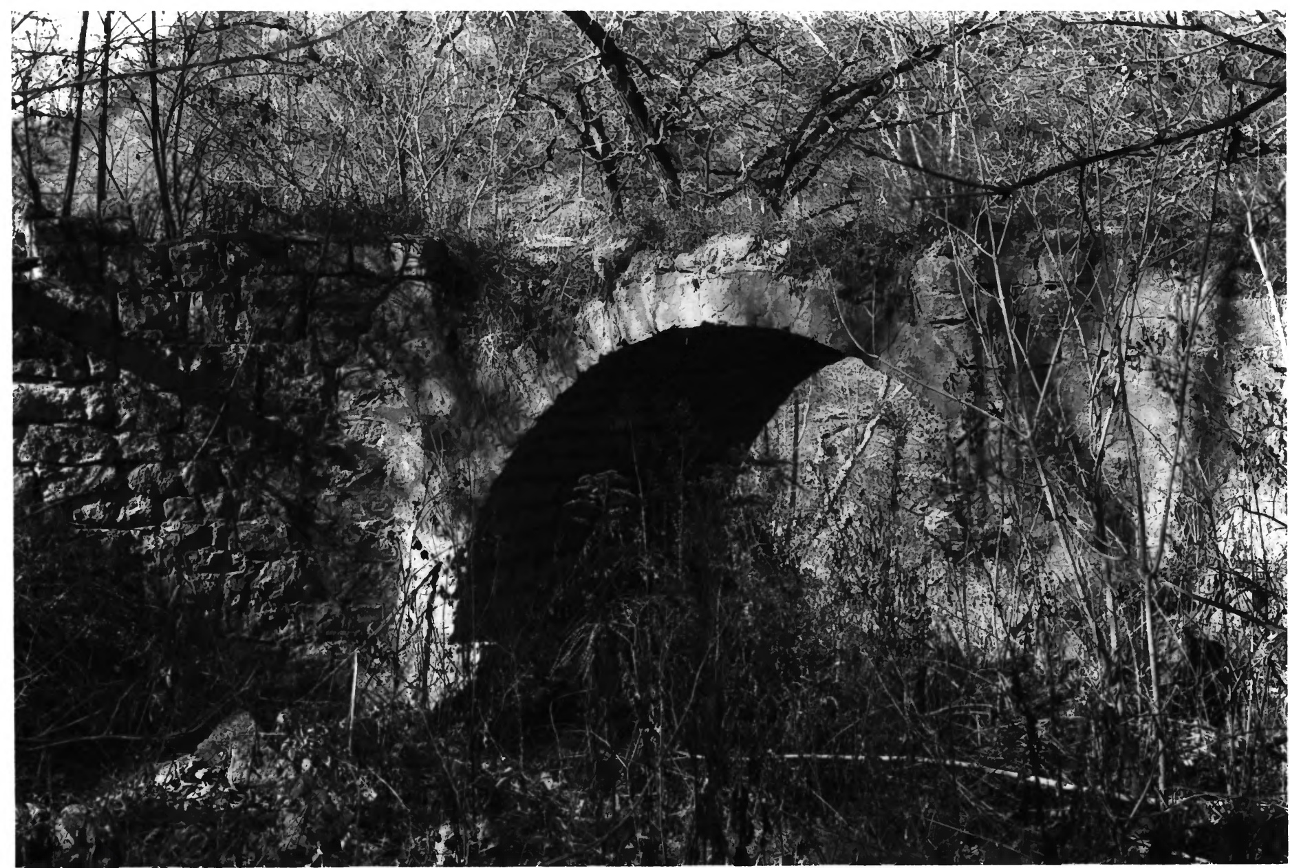
BRIDGE NO. L 4013 HOUSTON CO., MN PHOTO I.D. 09369#16
