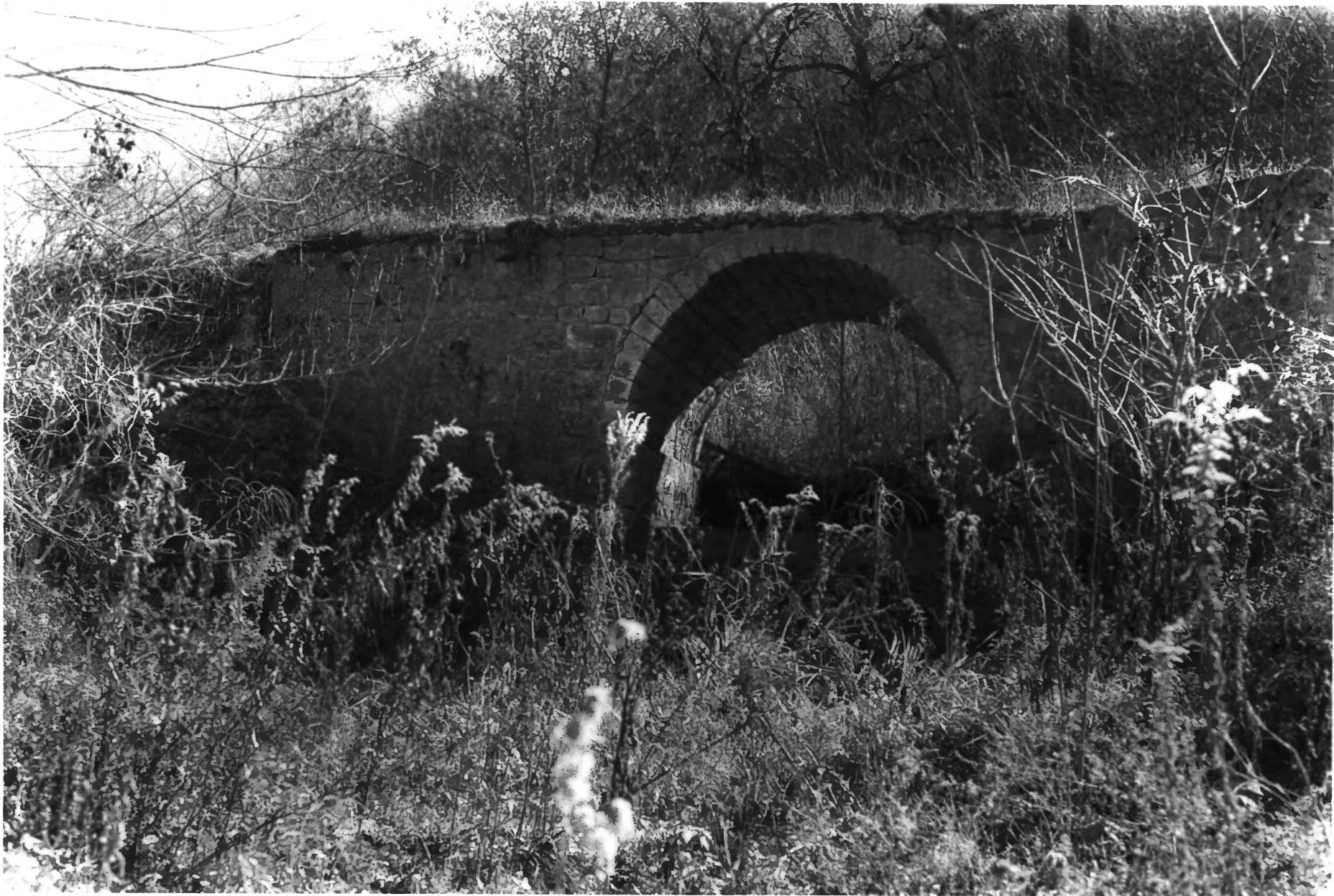
BRIDGE NO. L4013 HOUSTON CO., MN PHOTO I.D. 09369 #10
