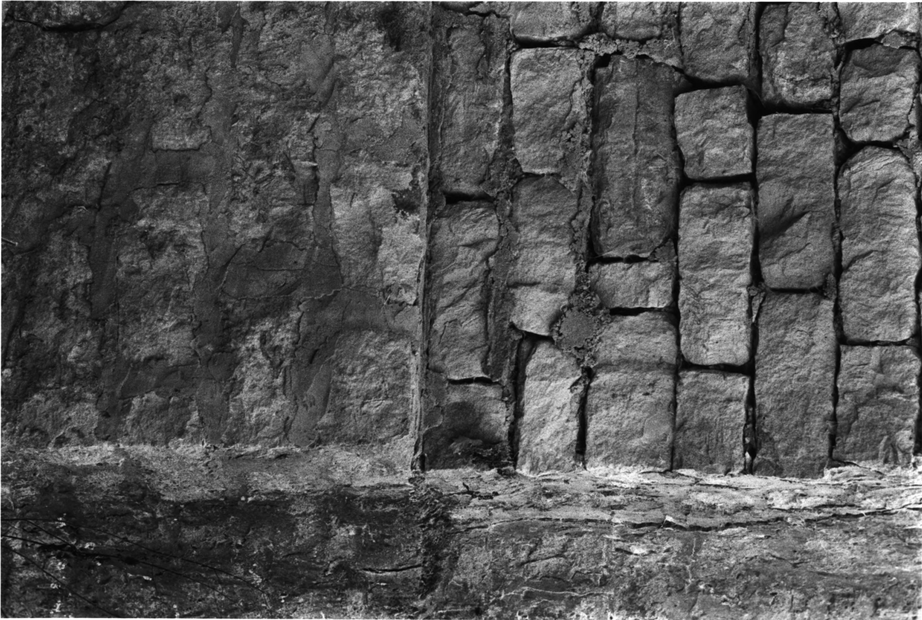
BRIDGE NO. L4013 HOUSTON CO., MN. PHOTO I. D. '09369 #12
