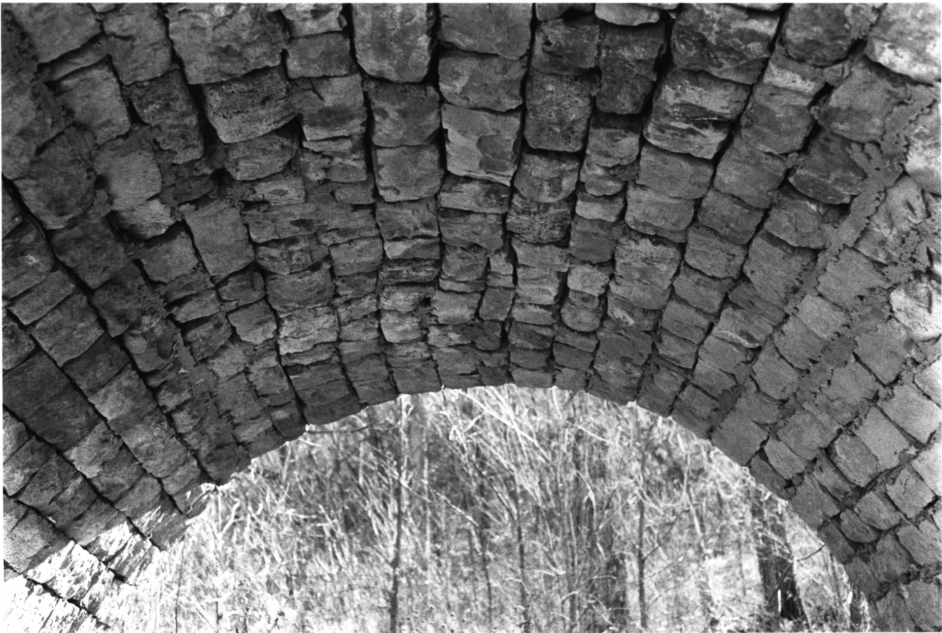
BRIDGE NO. L 4013 HOUSTON CO., MN PHOTO I.D. A9369 #13
