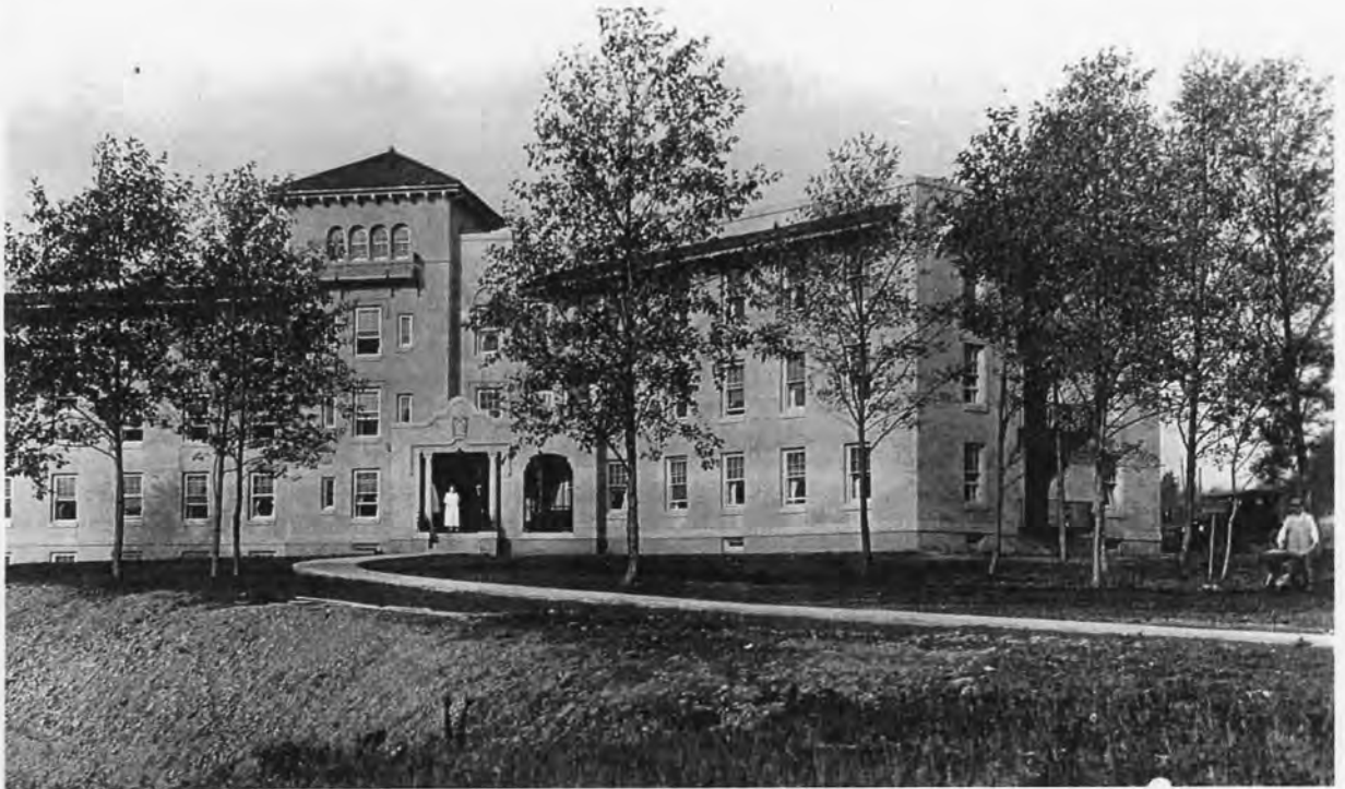
1920s-30s VIEW OF THE FRONT, SOUTHEAST FACADE OF NURSES' HALL No. 1.
