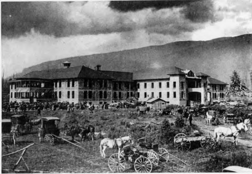
CA. 1911 VIEW SHOWING THE SIDE FACADES OF THE ADMINISTRATION BUILDING DURING CONSTRUCTION.
