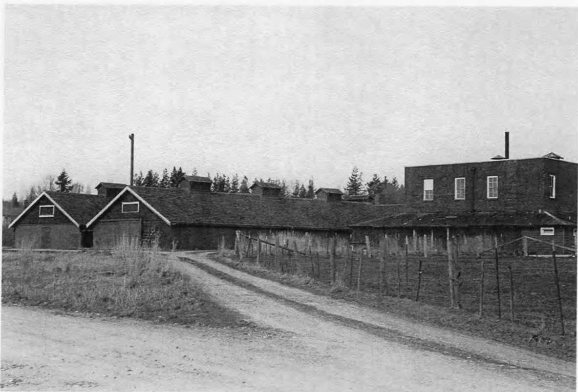
1950s-60s VIEW OF THE ROOT HOUSES AND CANNERY BUILDING.
