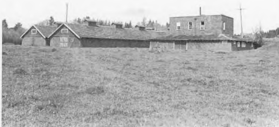
1940s-50s VIEW LOOKING NORTHWEST AT THE CANNERY AND ROOT HOUSE BUILDINGS.
