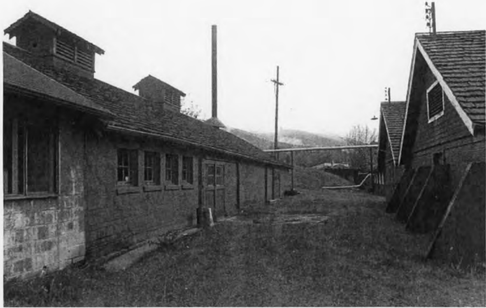
1940s-50s view looking east between the boiler house (left) and root houses (right).
