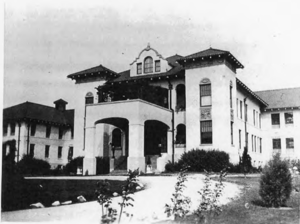
1920s VIEW OF THE FRONT, SOUTH FACADE OF THE ADMINISTRATION BUILDING.
