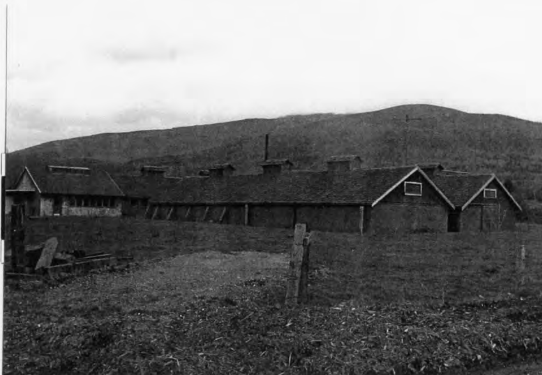
1950s-60s VIEW LOOKING NORTHEAST AT THE BOILER HOUSE AND TWO ROOT HOUSES.
