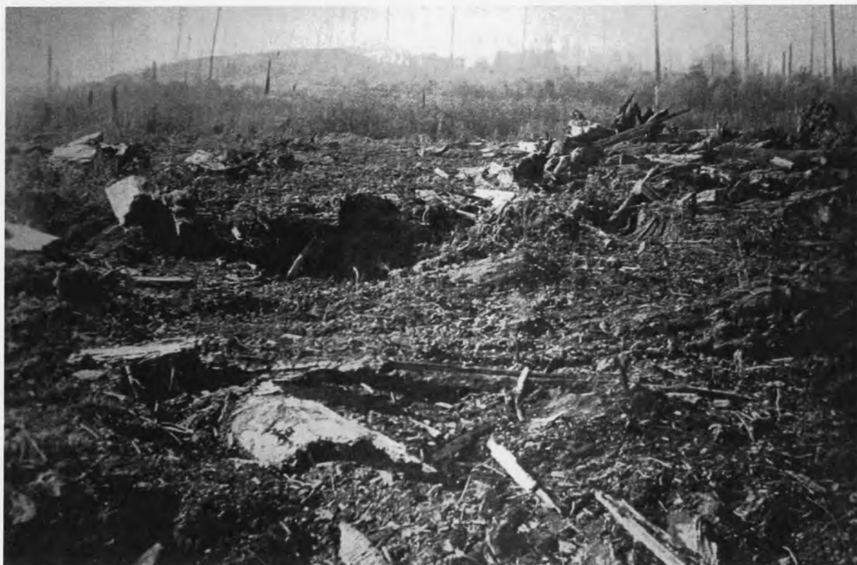
CA. 1914 VIEW OF GRADING ONGOING AT THE NSH SITE.
