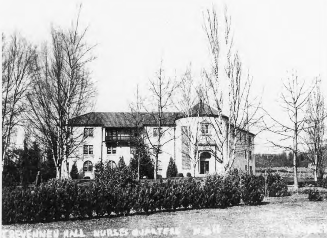
1940s VIEW OF THE FRONT EAST FACADE OF NURSES' HALL No. 2.
