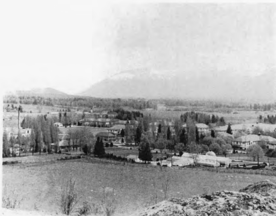
1940s-50s VIEW LOOKING SOUTHWEST OVER NSH GROUNDS AND BUILDINGS.
