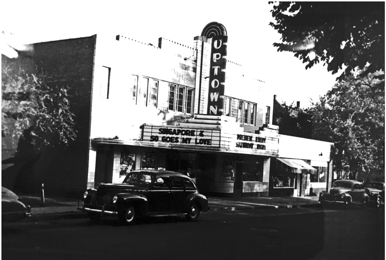
Fig. 1. Historic circa 1947 photograph of 1212 (left, theater) and 1210 (right, with awning) North Hudson.
