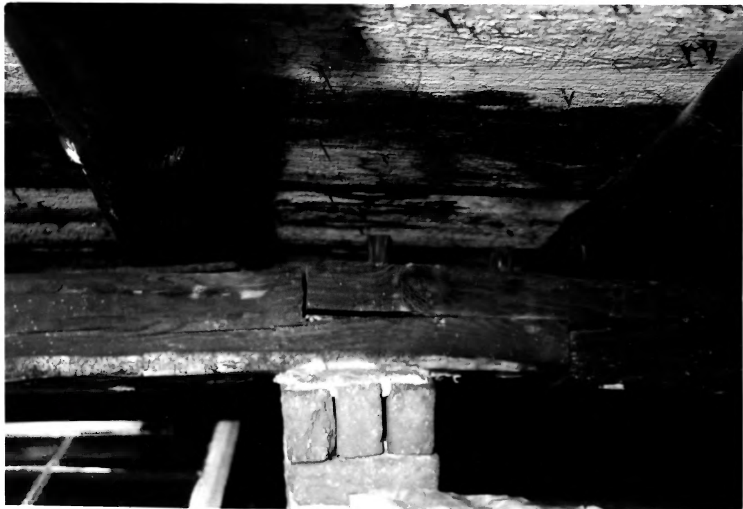
Kellett. Bolling. Stewart Place. Hickory Tavern Rd, Fountain Inn, S. C. 12
