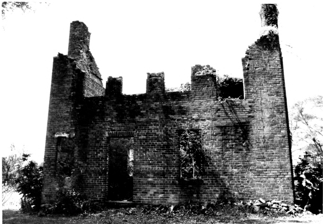
Kellett Bolling Stewart Place Hickory Tavern Rd. FOUNTAIN INN, S.C 15
