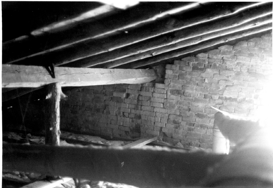
Kellett Bolling Stewart Place Hickory Tavern Rd. FOUNTAIN INN, S.C. 28
