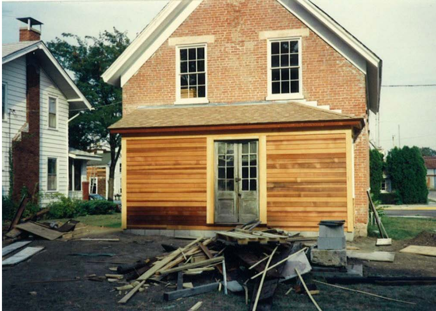
Dr. Burns House in 1990, rear elevation before restoration
