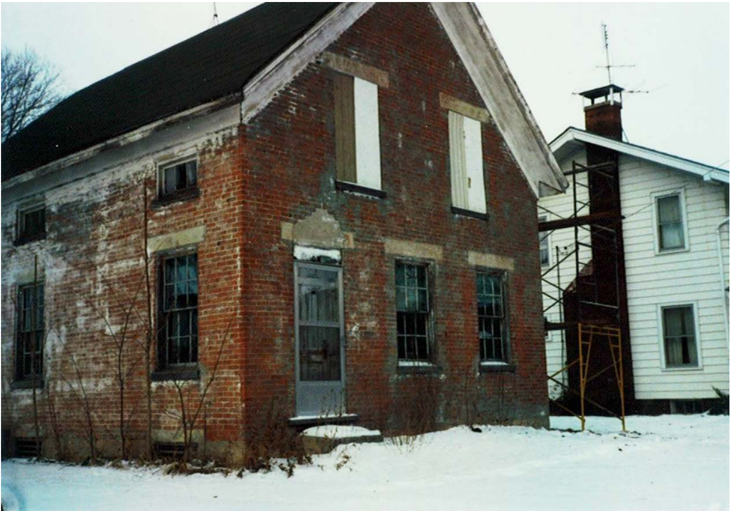
Dr. Burns House in 1990, front elevation before restoration
