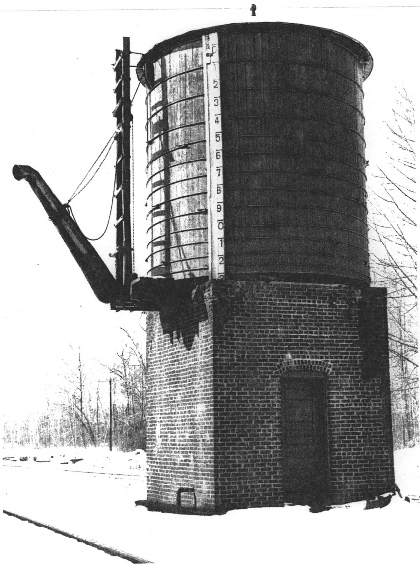
5 of 11 MORRISTOWN & ERIE RAILROAD WHIPPANY, NJ WATER TANK Photo Date: Early-1960's Whippany Railway Museum Collection
