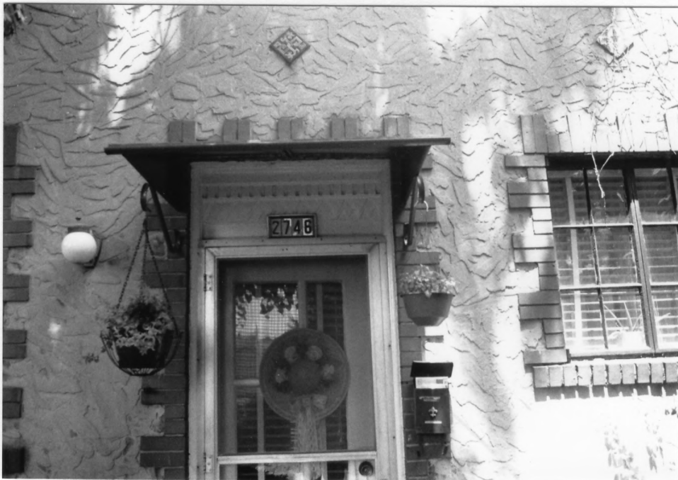
DRAFTING ROOM ADDITION ENTRANCE
