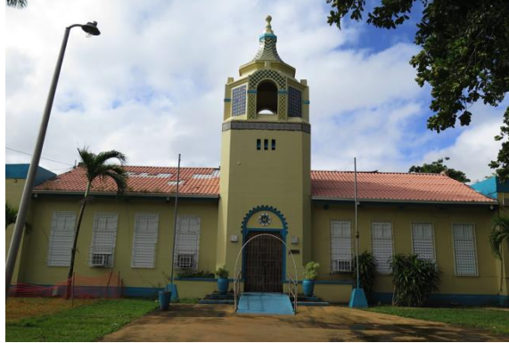
Figure 27. Principal Façade Main Building, 1925-1928, Joseph O'Kelly, Instituto Loaiza Cordero para Niños Ciegos Historic District, APC, 2018.
