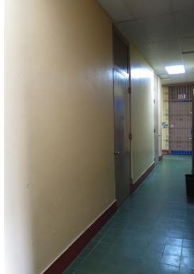
Figure 32. Interior view of the corridor, principal building, 1925-1928, Joseph O'Kelly, Instituto Loaiza Cordero para Niños Ciegos Historic District, APC, 2018.
