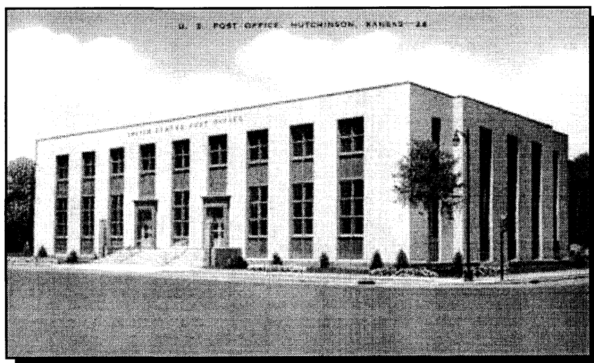
The Post Office: one of the many WPA projects during the 1930s
