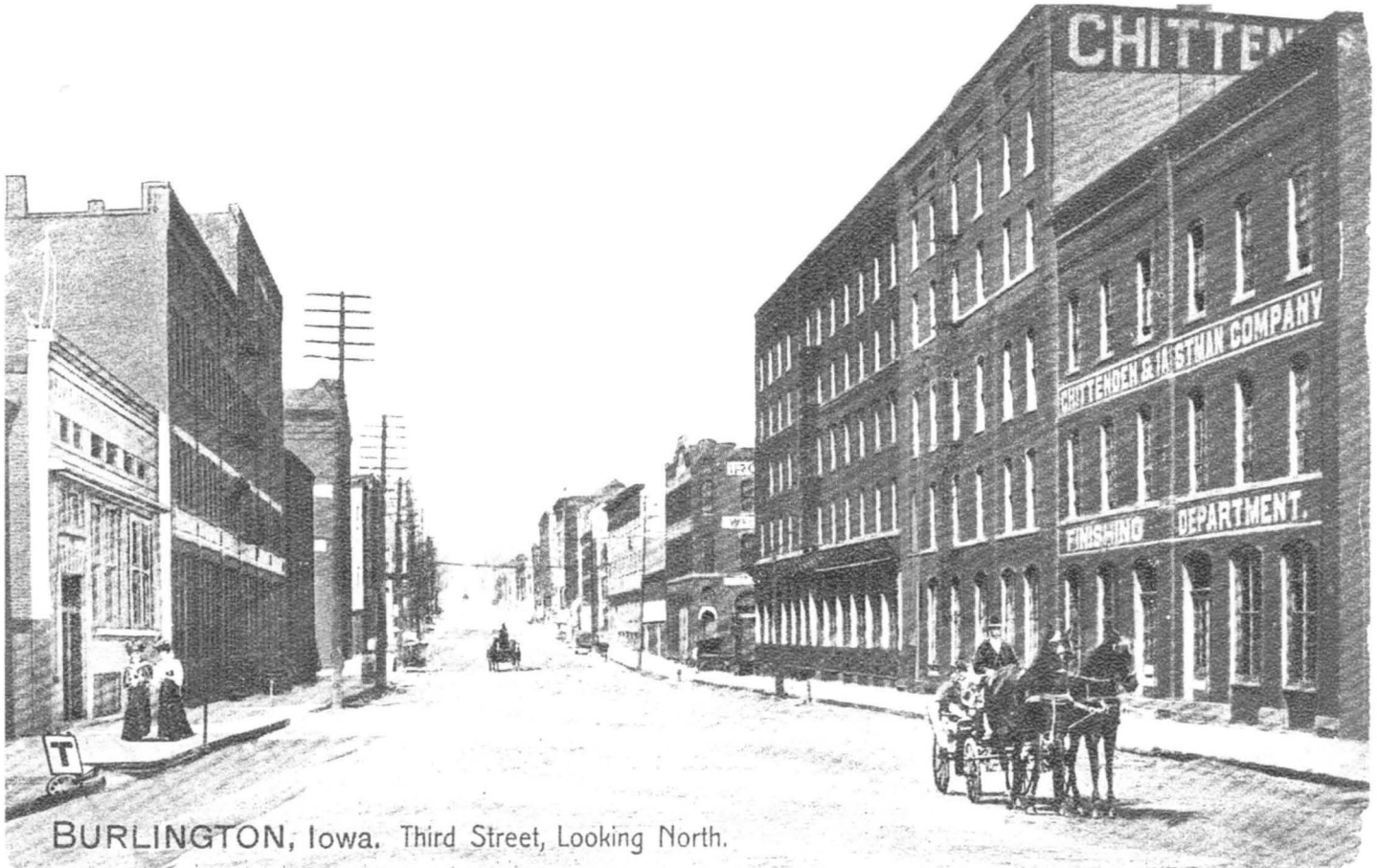
Figure 24. Postcard view of actual Chittenden and Eastman buildings on S. 3 rd Street (1910 postmark), looking north – left: office (Map #22), factory buildings (Map #21-20), and older small building (site of Map #19) - right: original five story buildings (Map #12-13), three-story building enlarged to five stories (Map #14), and two-story Burlington Vinegar and Pickle Works building enlarged to three stories (Map #15) (BPL postcards: streets 010).
