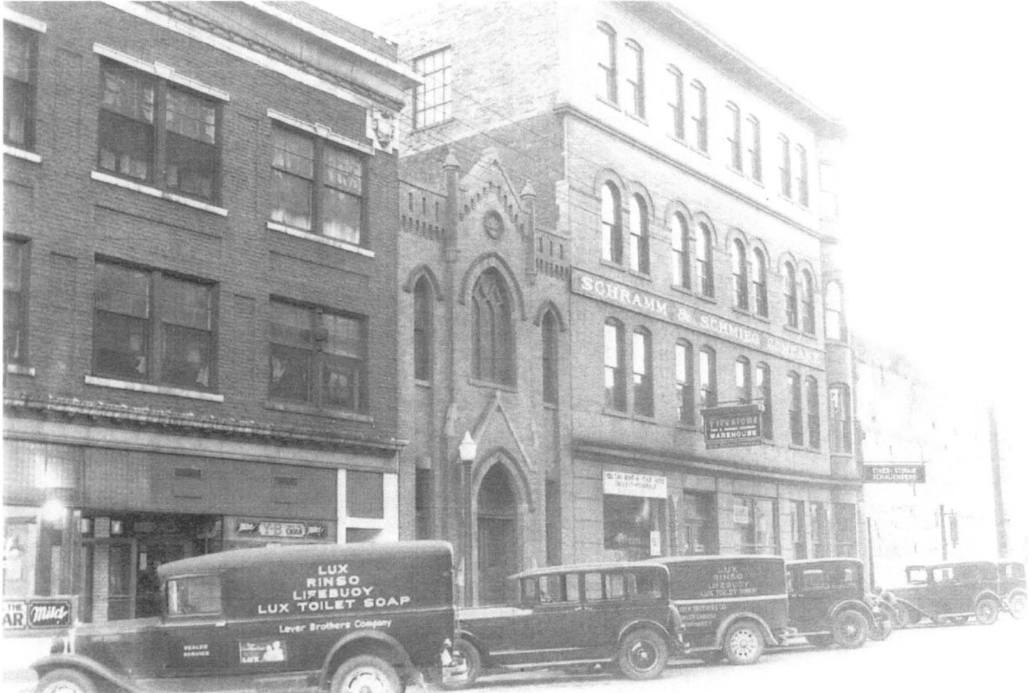
Figure 32. Unterkircher building expanded for Schramm & Schmieg factory at right, looking southwest (DMCHS image file).
