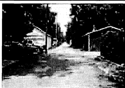
Alley Between Rhode Island and New Hampshire Streets, Looking North from 14 th Street (Photo #33)
