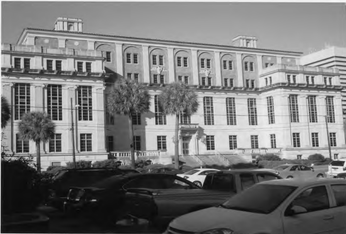
1. John C. Calhoun State Office Building 1015 Sumter Street, Columbia Richland County, South Carolina
