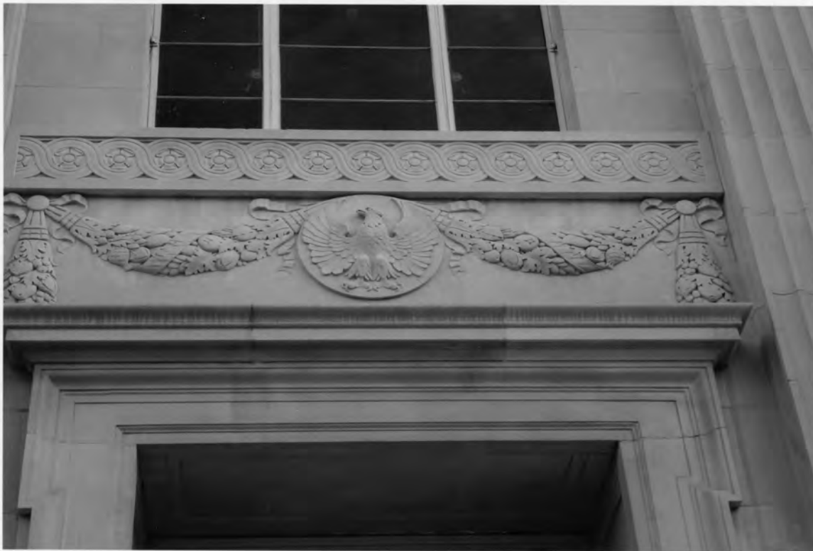
19. John C. Calhoun State Office Building 1015 Sumter Street, Columbia Richland County, South Carolina
