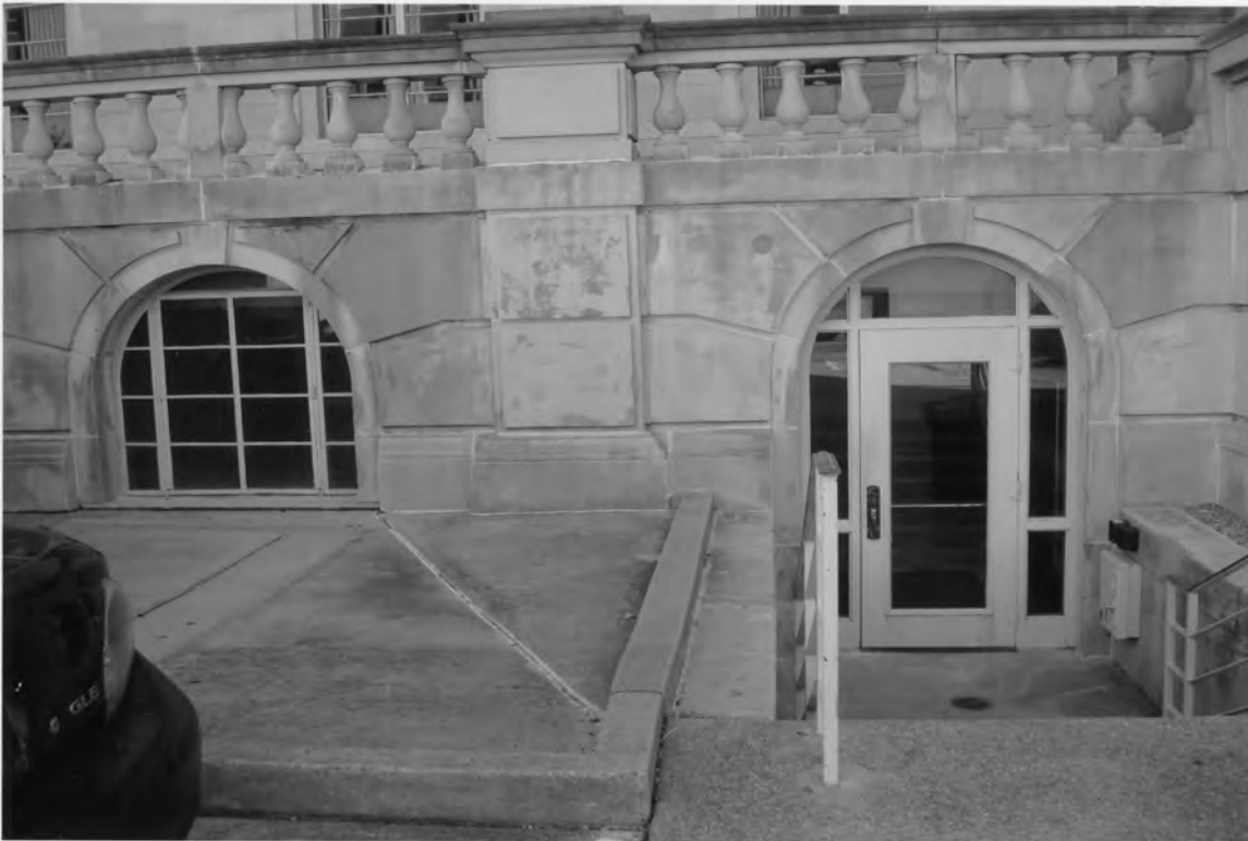
23. John C. Calhoun State Office Building 1015 Sumter Street, Columbia Richland County, South Carolina
