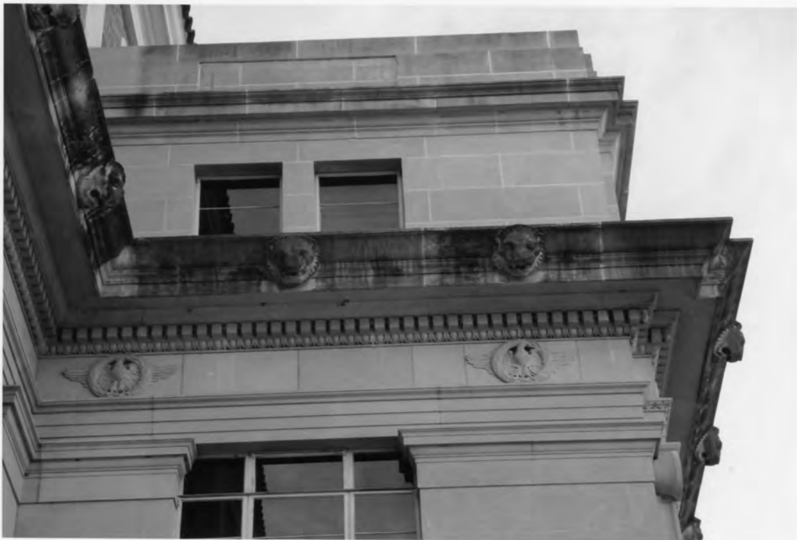
18. John C. Calhoun State Office Building 1015 Sumter Street, Columbia Richland County, South Carolina
