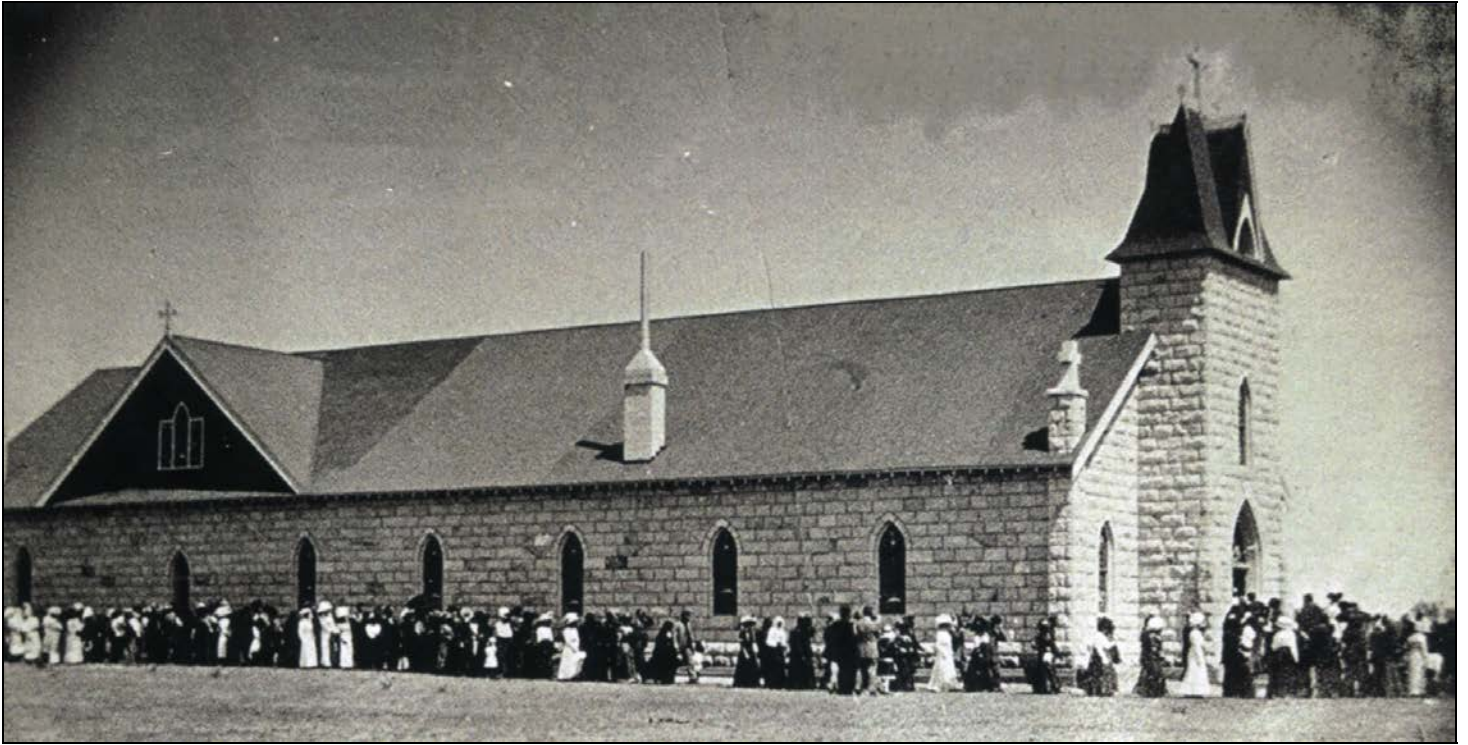
Figure 3. Bishop Nicholas Matz of the Diocese of Denver blessed the church on 3 July 1913 (view north-northwest). Note that the tower featured a different top at that time. Courtesy of 100 Year, 1912-2012 Anniversary Jubilee (2012), 5.
