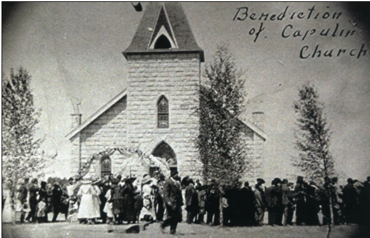
Figure 4. This view west shows the front (east wall) of the church at the 3 July 1913 blessing. Note the different tower design, presence of stained glass, and the absence of the one-story stone section to the north (right). Courtesy of 100 Year, 1912-2012 Anniversary Jubilee (2012), 5.
