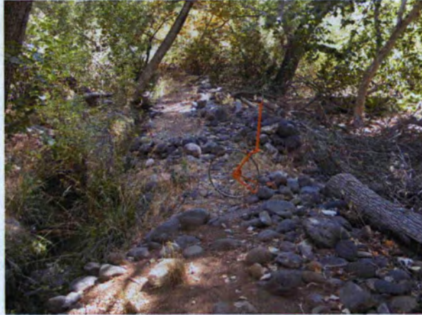
Location along ditch where water was likely diverted at some point in the past, based on squared corners in walls.
