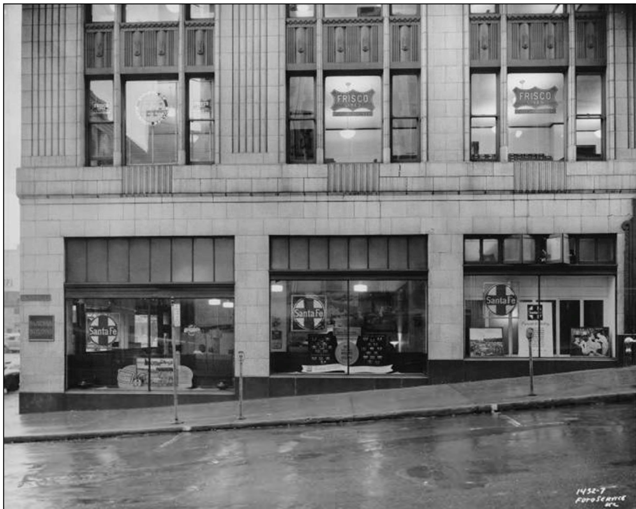
Figure 18: Fairfax Building 1943, detail of Main or north façade facing south.
