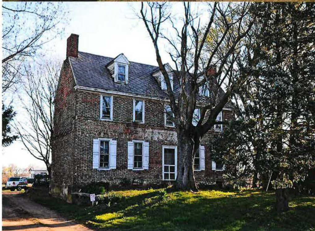
Figure 2: Top photo: Homestead Hall's four-bay front elevation with paired entry doors. Bottom photo: Hill Island Farm (Noxontown Farm), Thomas Rothwell III's later five-bay Georgian dwelling with central entry door and stair hall.
