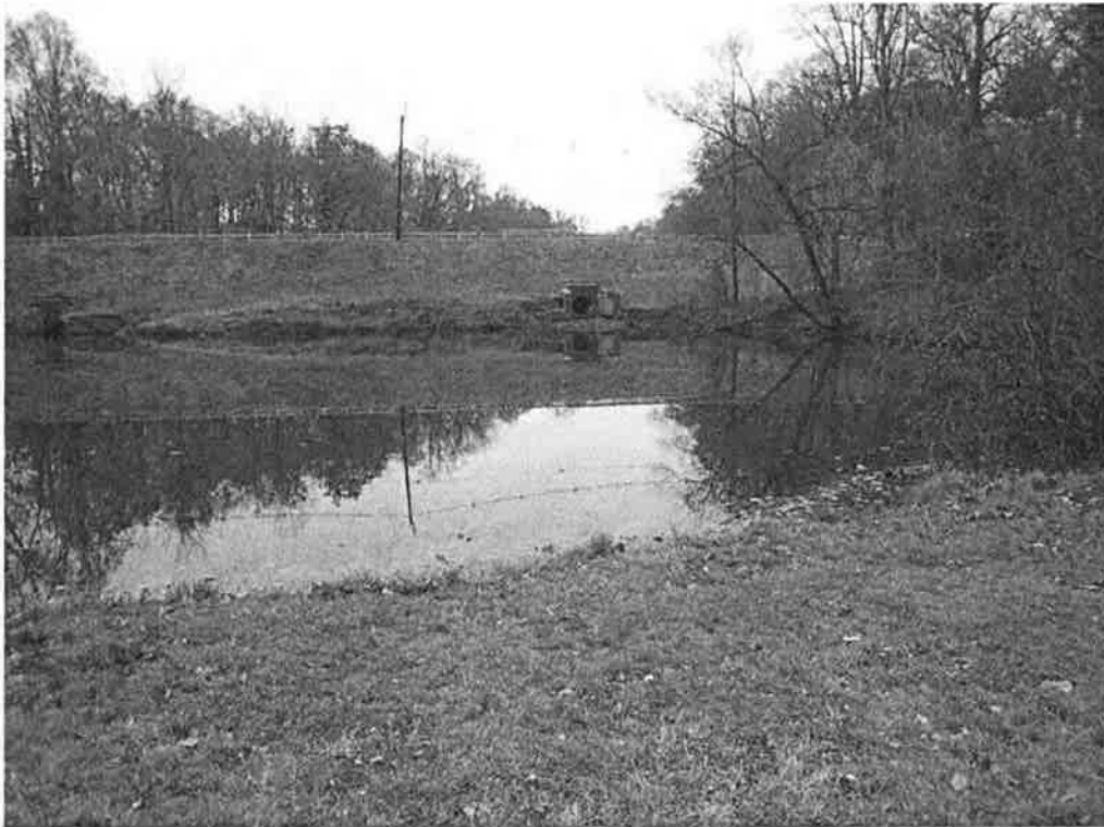
Cooper River Park Historic District, Camden County, NJ Photo 54 (RS) Hopkins Pond Dam (non-contributing resource) north side, view from Driscoll Pond (foreground), Camera facing west
