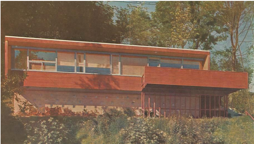
Alden Mason House I, 2545 Boyer Ave E., Seattle. 1949 (Courtesy, MCCalls Book of Modern Houses).
