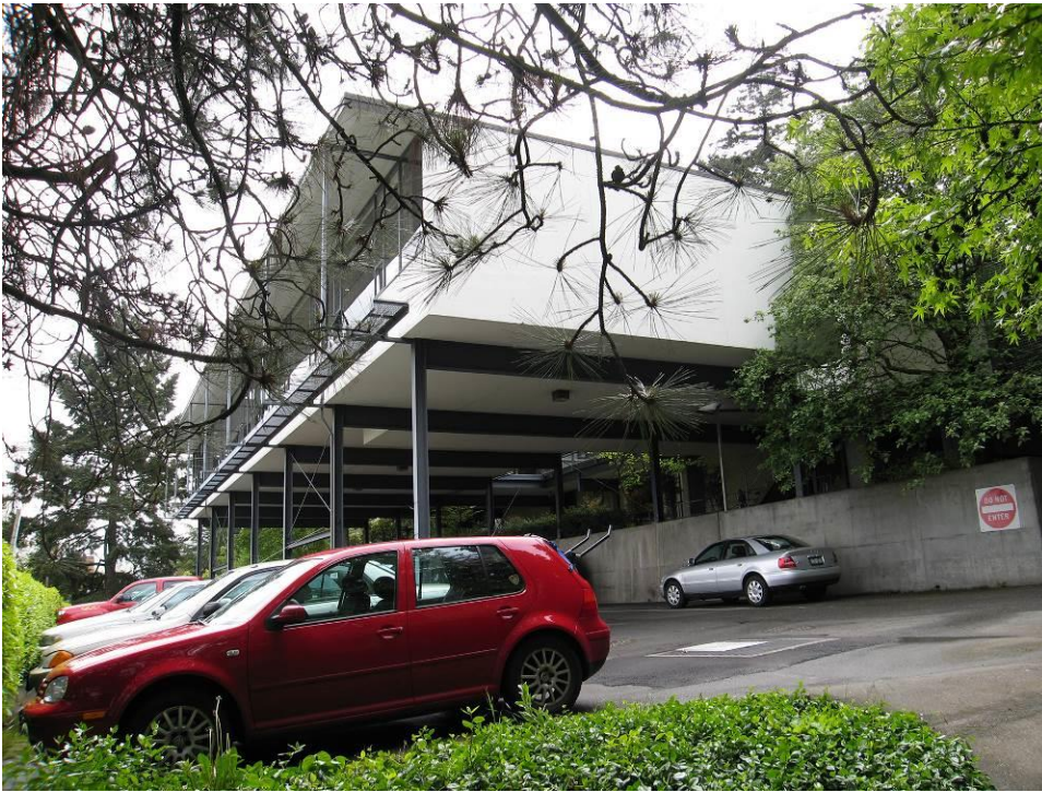
04. WA_KingCounty_UWFacultyClub_0004.tif Rear dining hall projection with covered parking.
