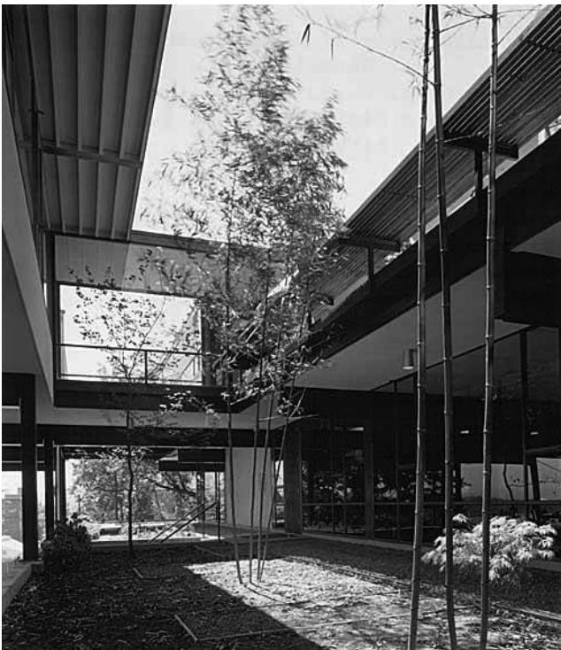
The gap between the dining room and the main building, looking at the open central courtyard to the upper right (seating bench slats visible), 1960 (Courtesy, University of Washington Libraries, Special Collections Division, Dearborn Massar Photograph Collection)
