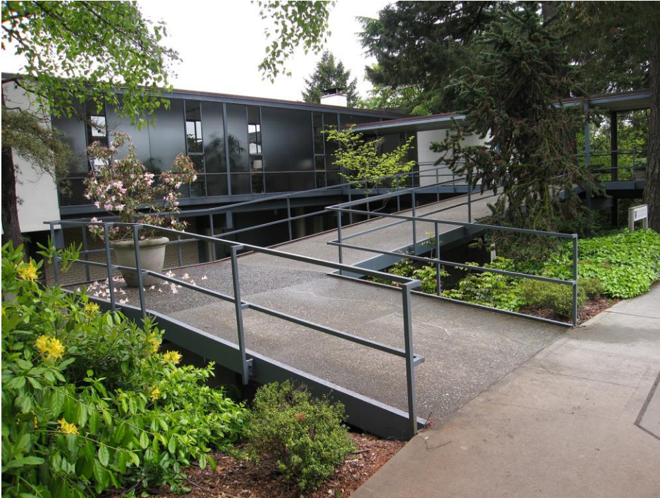
16. WA_KingCounty_UWFacultyClub_0016.tif Entry ramp of Stevens Way.
