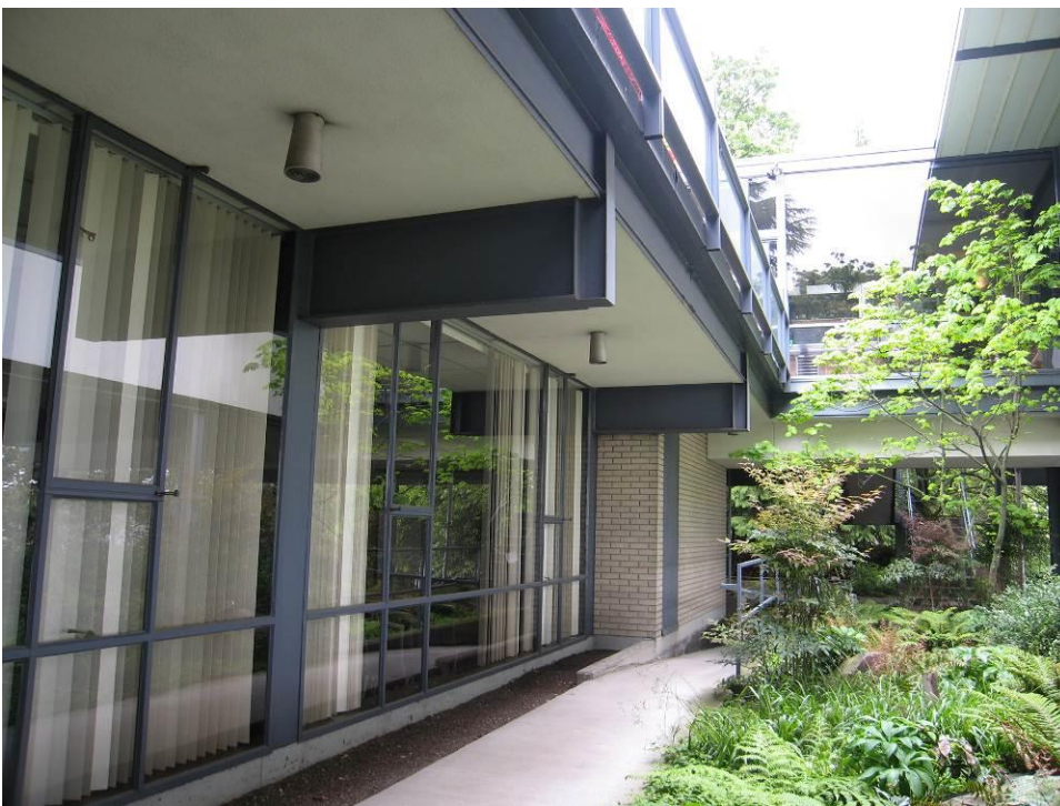
05. WA_KingCounty_UWFacultyClub_0005.tif Lower level of interior courtyard showing wall detailing.
