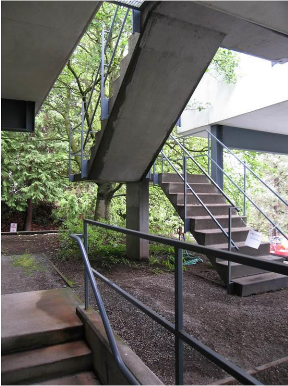
06. WA_KingCounty_UWFacultyClub_0006.tif Secondary exterior stair from courtyard to covered parking.
