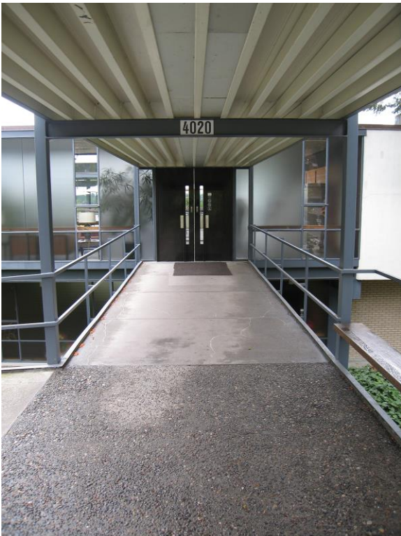
15. WA_KingCounty_UWFacultyClub_0015.tif Entry ramp detail leading to main entry door.
