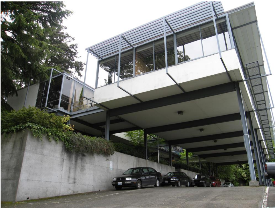
17. WA_KingCounty_UWFacultyClub_0017.tif Rear covered parking area.
