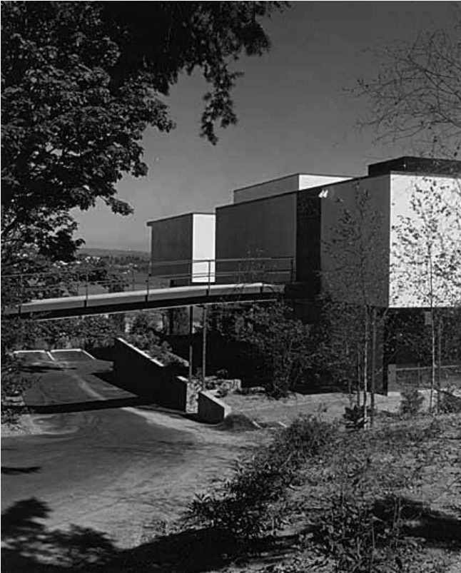
North façade, Faculty Club, 1960. To the east (left) of the walkway, a cantilevered walk-in refrigerator was added in 1987 and sided in corrugated metal to distinguish it from the original building (Courtesy, University of Washington Libraries, Special Collections Division, Dearborn Massar Photograph Collection).
