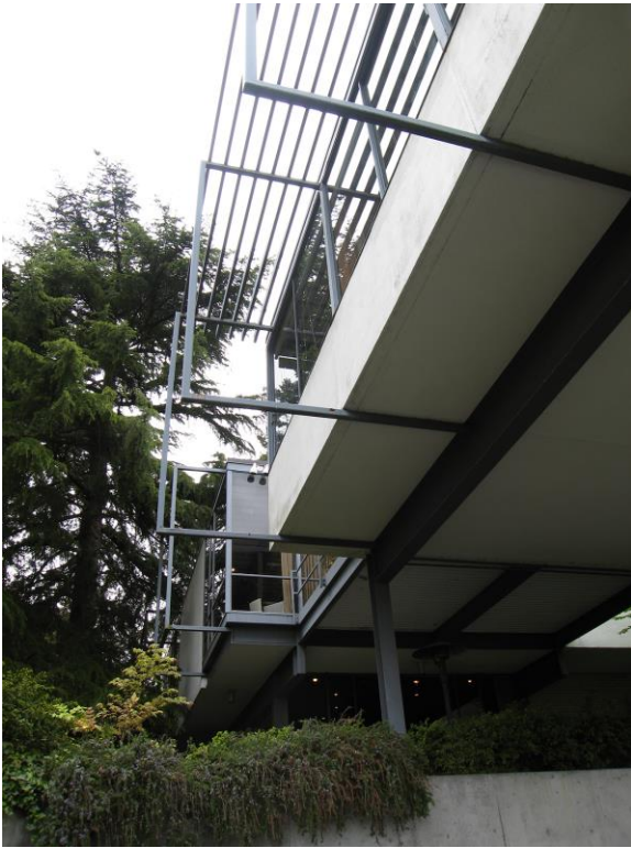
14. WA_KingCounty_UWFacultyClub_0014.tif Detail of dining room cantilever and south facade.
