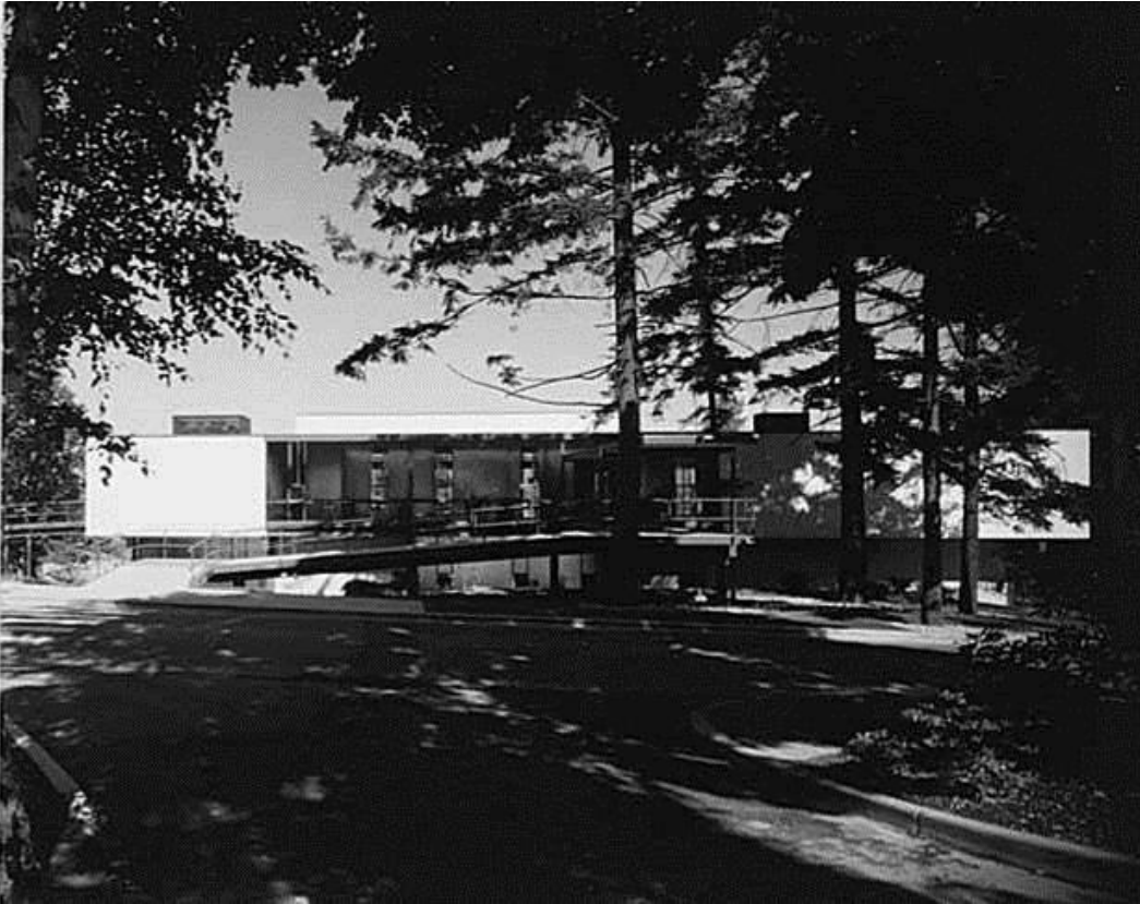
Exterior view, front (west) façade, 1960. With the exception of the walk-in addition to the left (north) façade, the façade remains the same. Foliage has matured (Courtesy, University of Washington Libraries, Special Collections Division, Dearborn Massar Photograph Collection).
