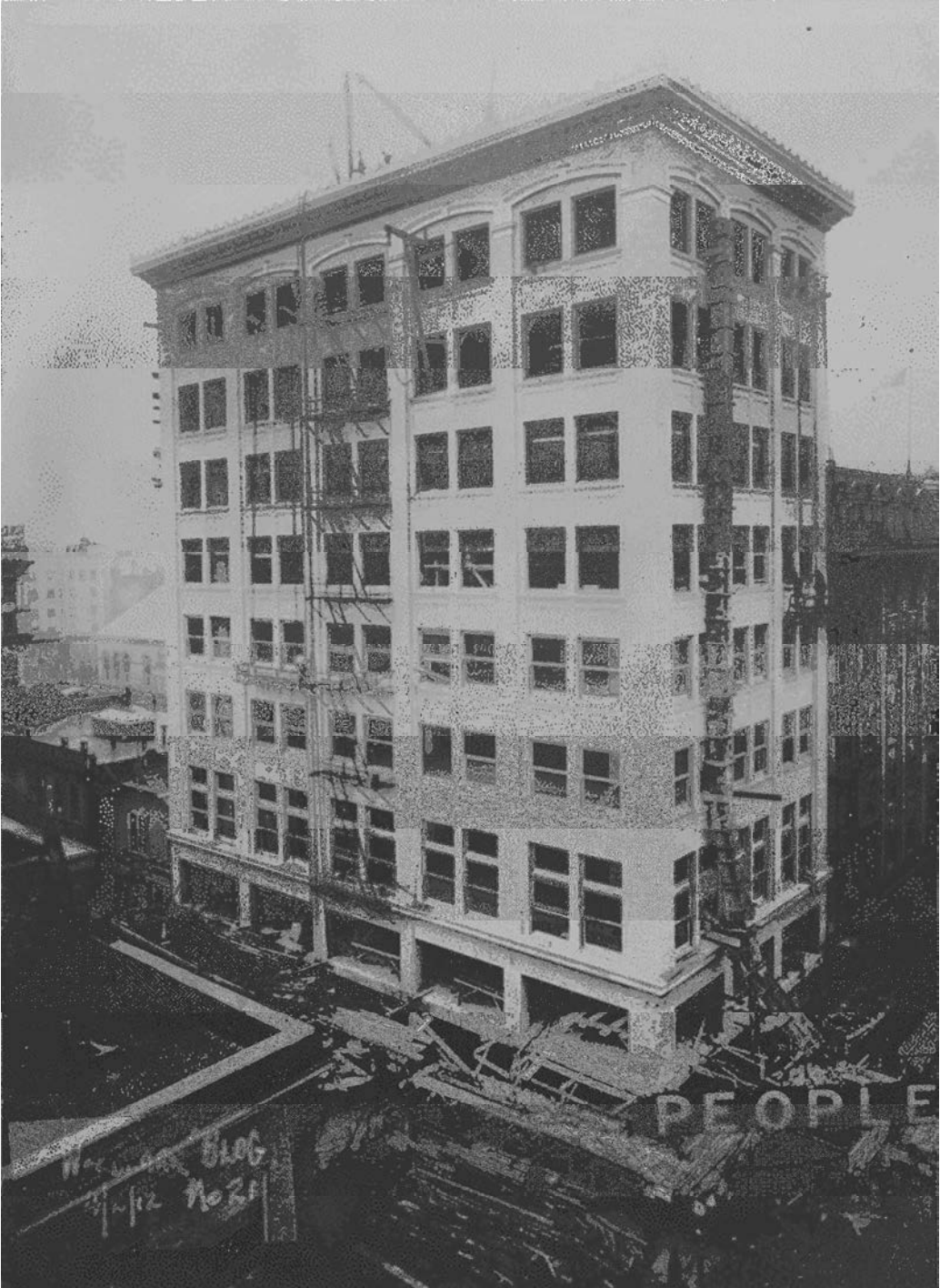
FIGURE 7: Woodlark Building Construction, April 2, 1912 (OHS bb011290)
